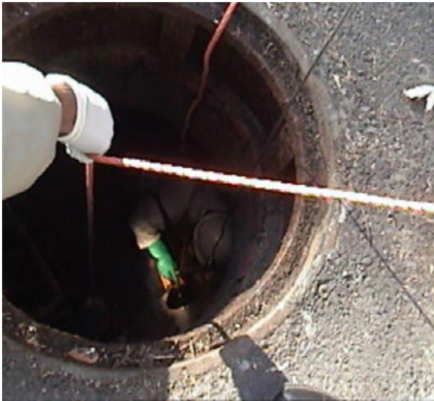
DEP staff begins sewer investigation
