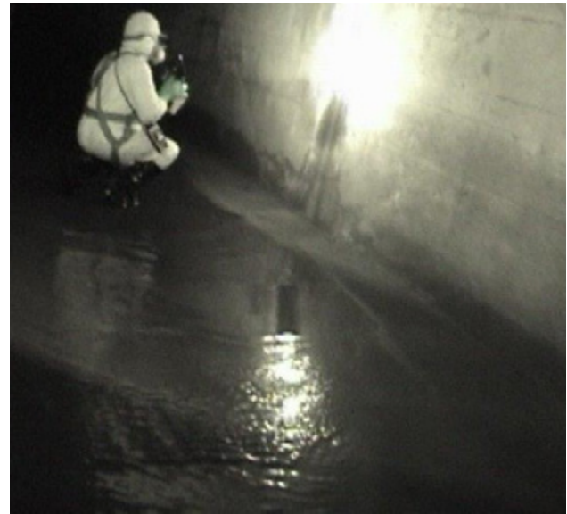
DEP staff conducts in-sewer investigation
