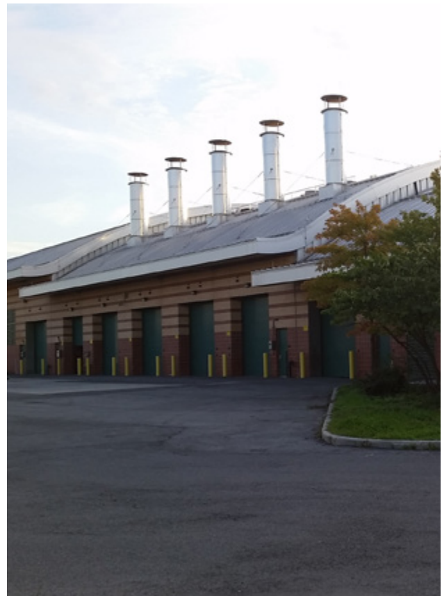
Paerdegat Basin CSO facility
