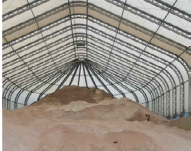
DSNY salt shed
