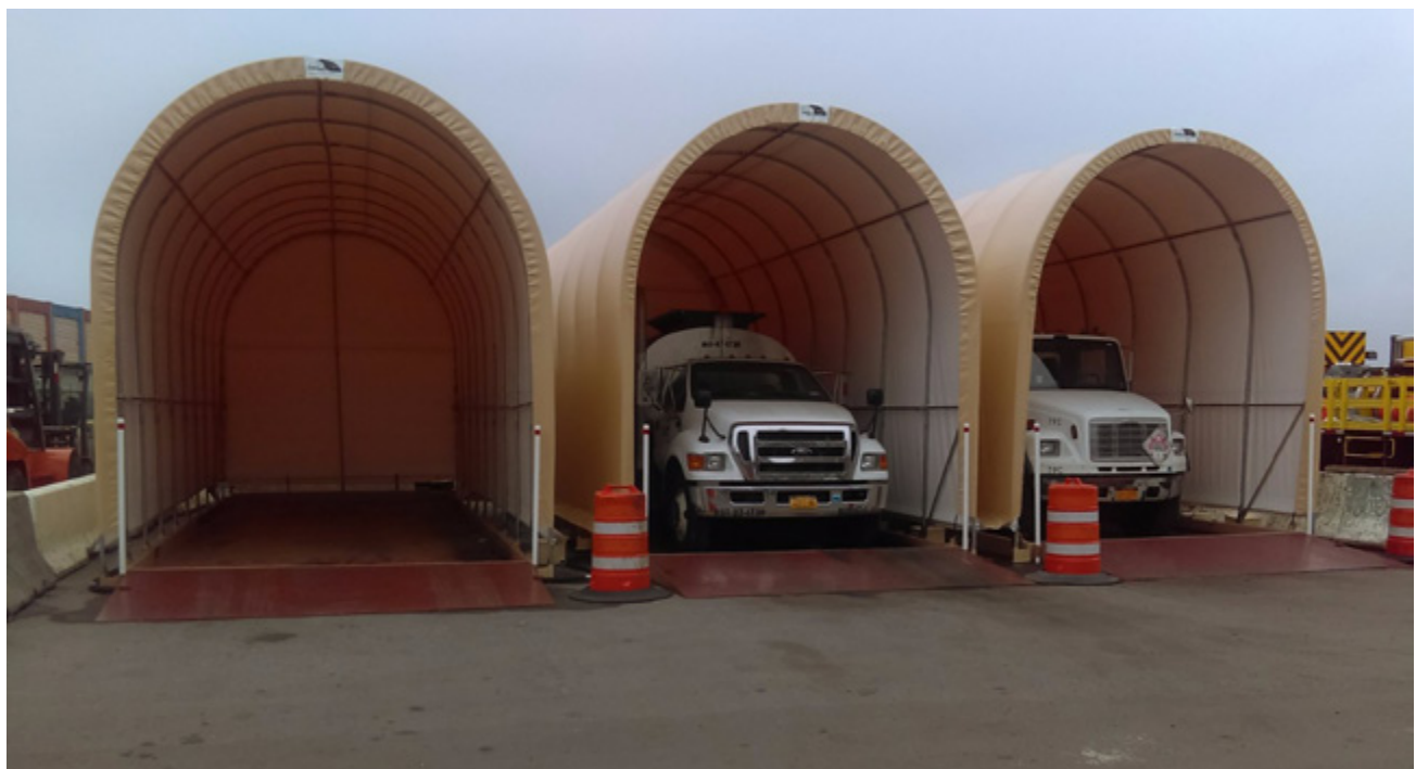
DOT trucks under cover and within secondary containment
