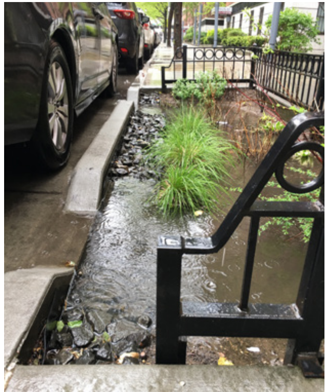
Rain garden construction in Flushing, Queens
