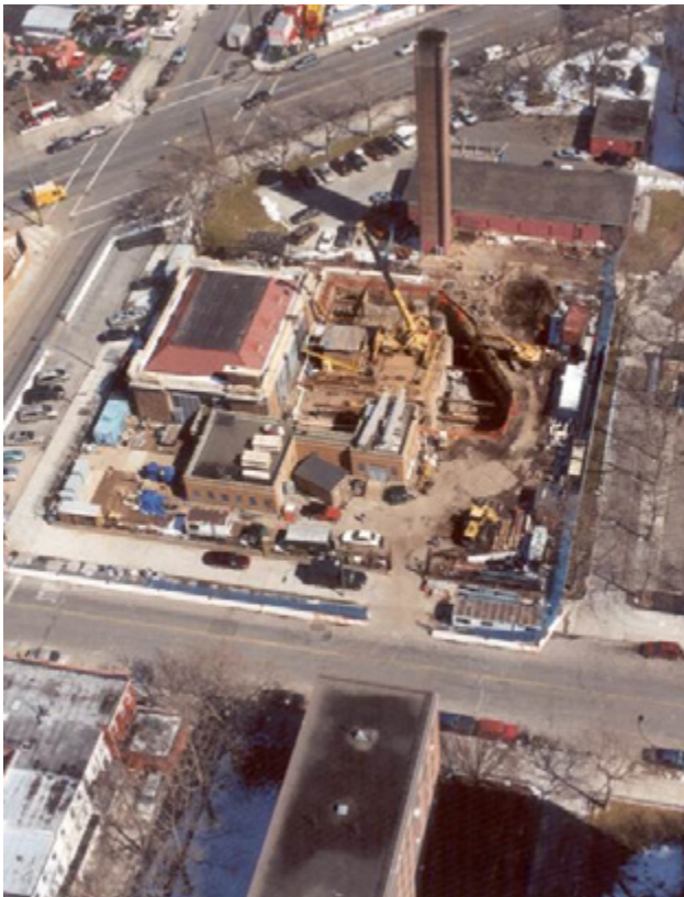
Construction at Avenue V pump station
