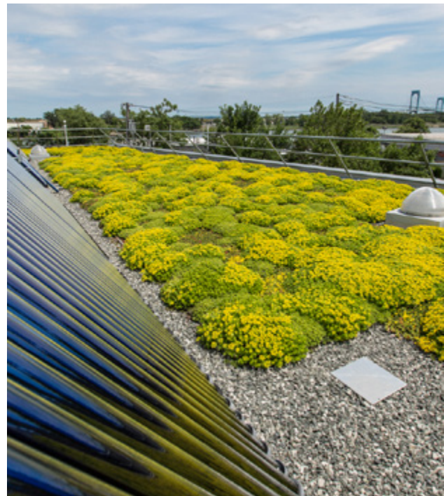
Green Roof at Zerega EMS Station
