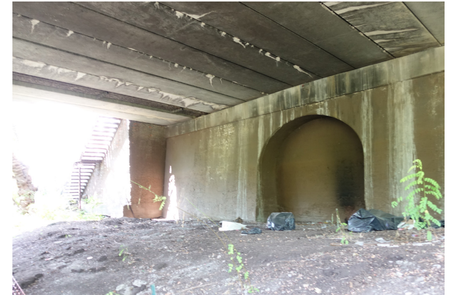
BRIDGE UNDERPASS (W. 233RD ST)
