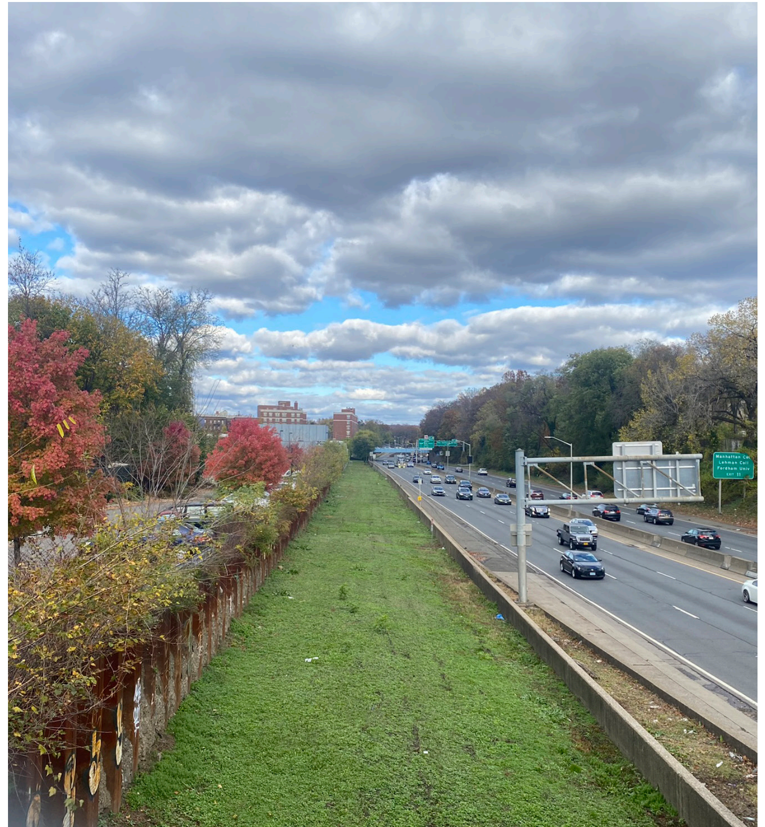
View from W. 234th St, looking North.
