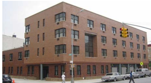
Marcy-Hart – Services for the Underserved, Bedford-Stuyvesant, Brooklyn
