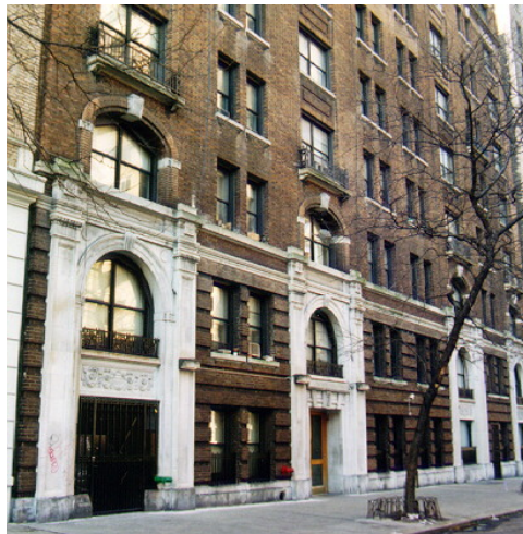
Capitol Hall Residence – Goddard Riverside Community Center, Upper West Side, Manhattan
