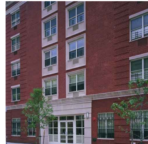
DeKalb Avenue Apartments – Dunn Development/Community Access, Inc., Bedford-Stuyvesant, Brooklyn
