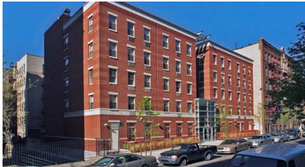
Corner House – Goddard Riverside Community Center, West Harlem, Manhattan
