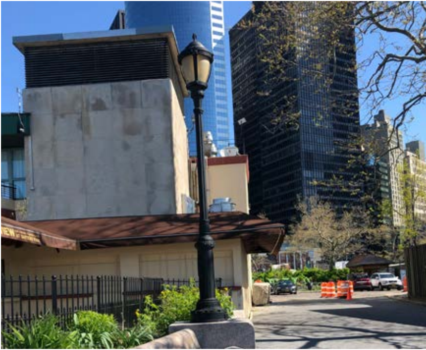
RIVERSIDE LUMINAIRE ON B-POLE LOCATED ON GRANITE BLOCKS OR GROUND ALONG WHARF
