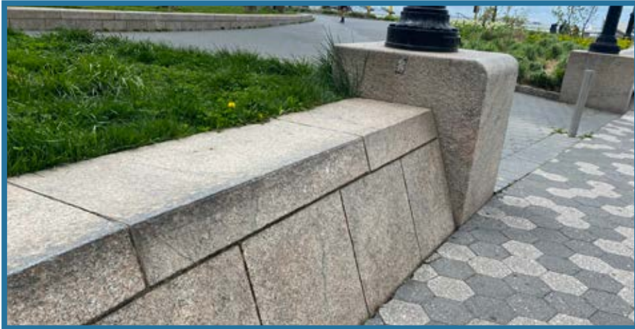
Pier A Planter Wall
