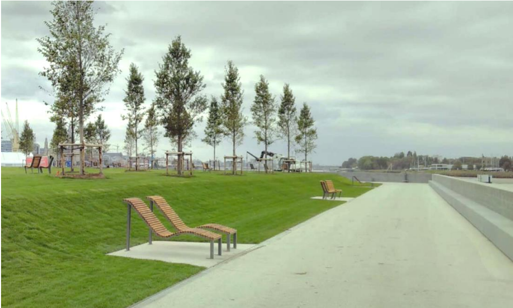
Scheldt Quay; Antwerp, Belgium Flood Protection+ Programmed Waterfront; Stabilization of Historic Quay Wall
