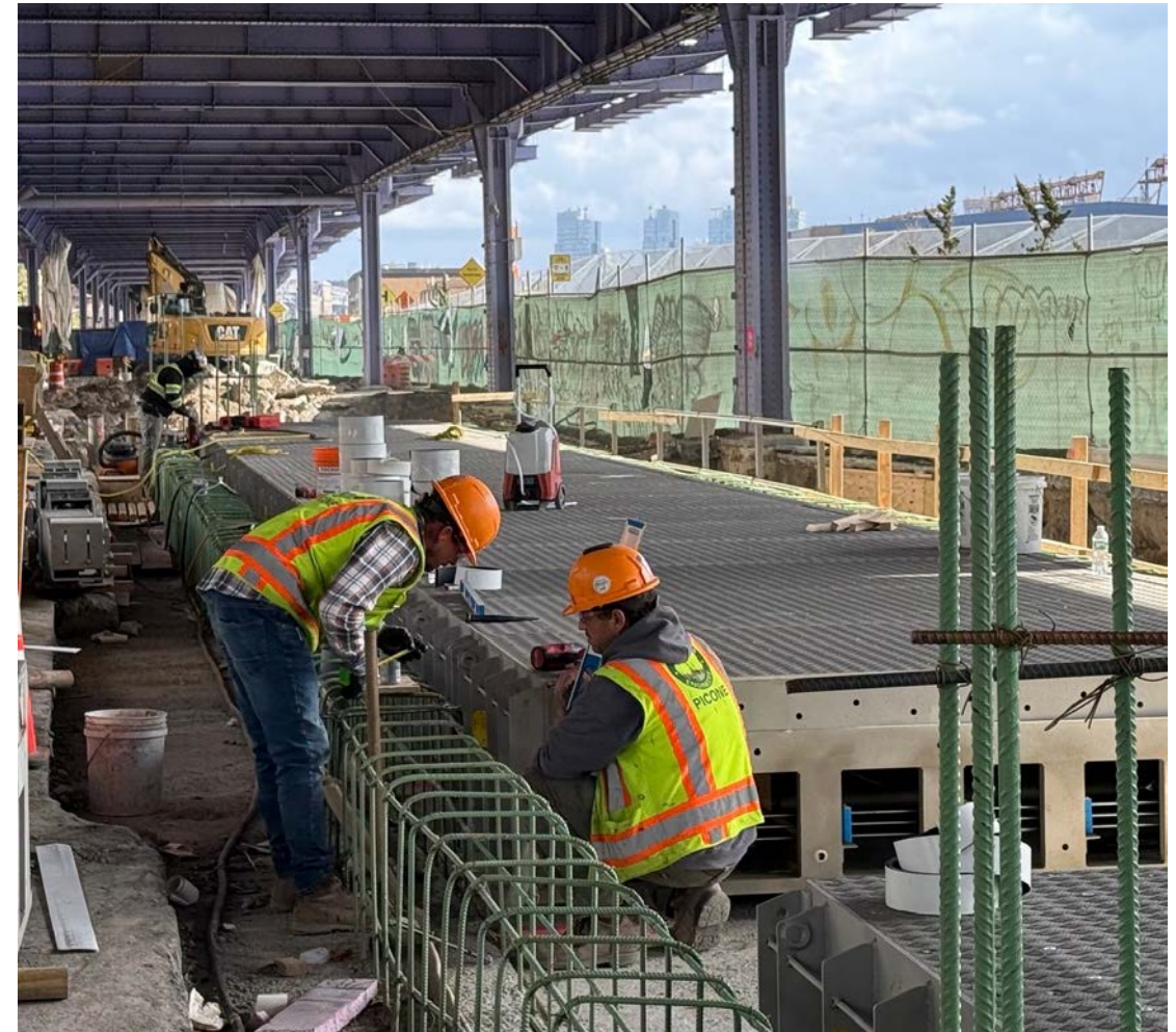
Flip up gates being installed – October 2024
