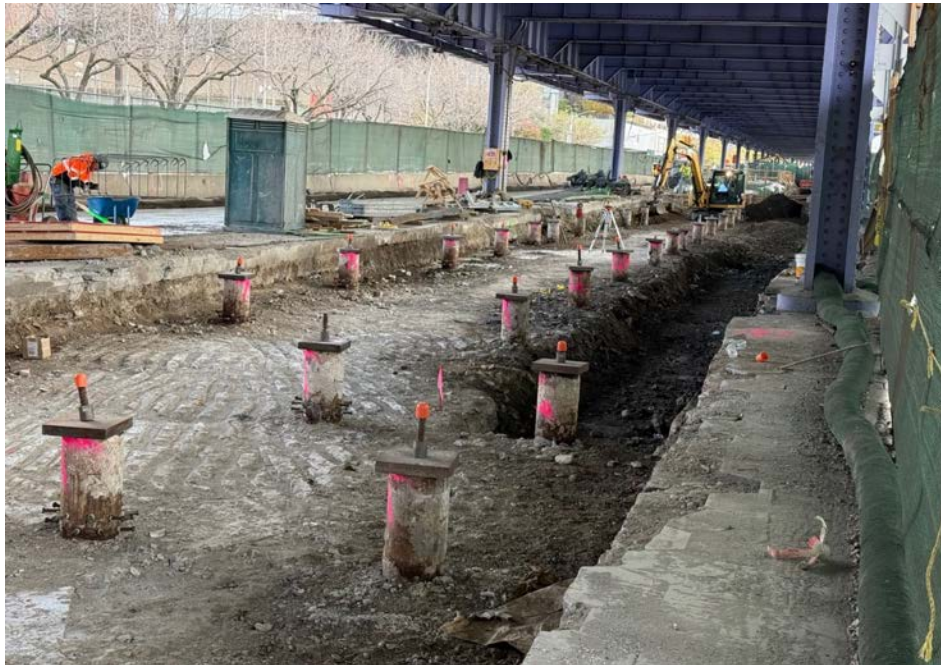
Micro-piles for floodgate foundation – October 2024
