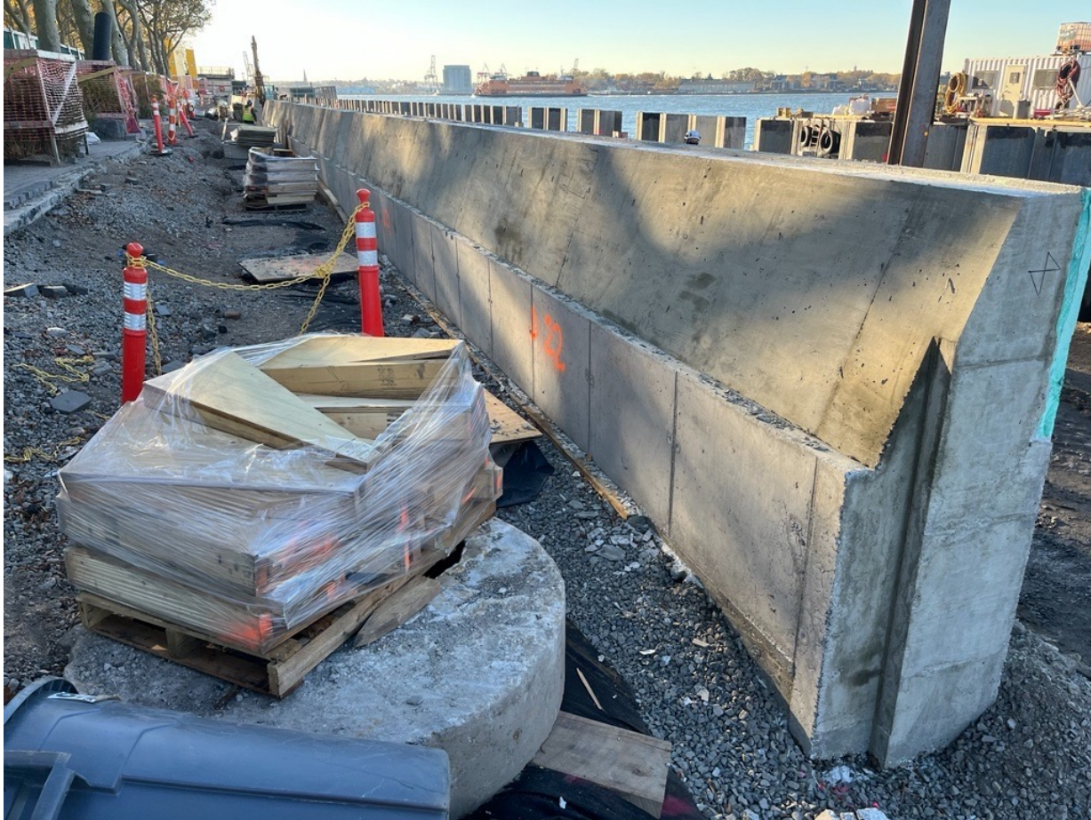
October 2024 – Concrete Benchwall Construction
