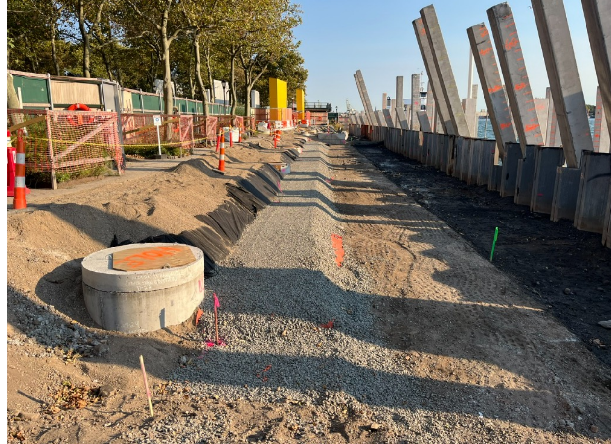
September 2024 – Storm Drainage Backfill and Compaction
