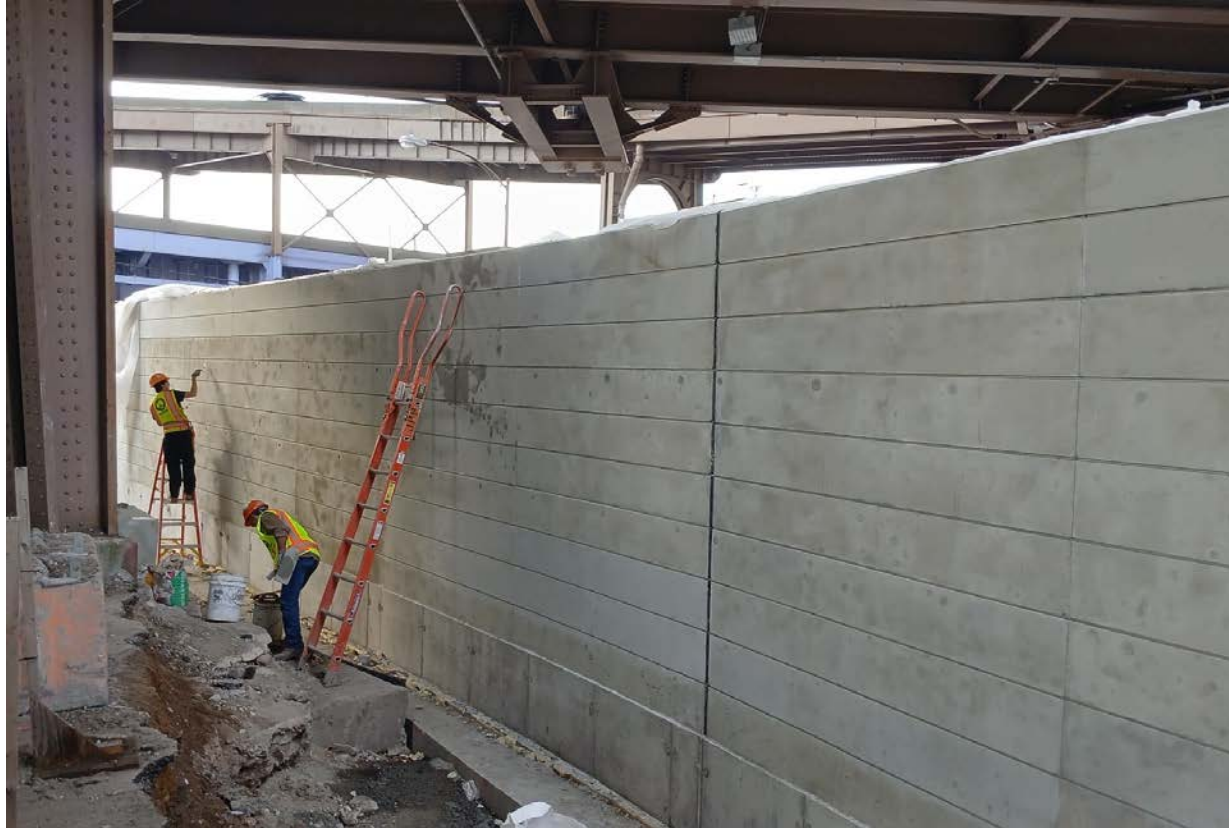
Floodwall near Robert F. Wagner Sr. Place – November 2024
