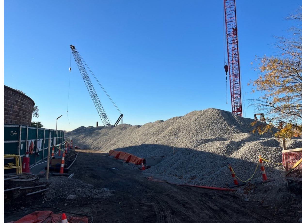
November 2024 – Lightweight Fill Placement
