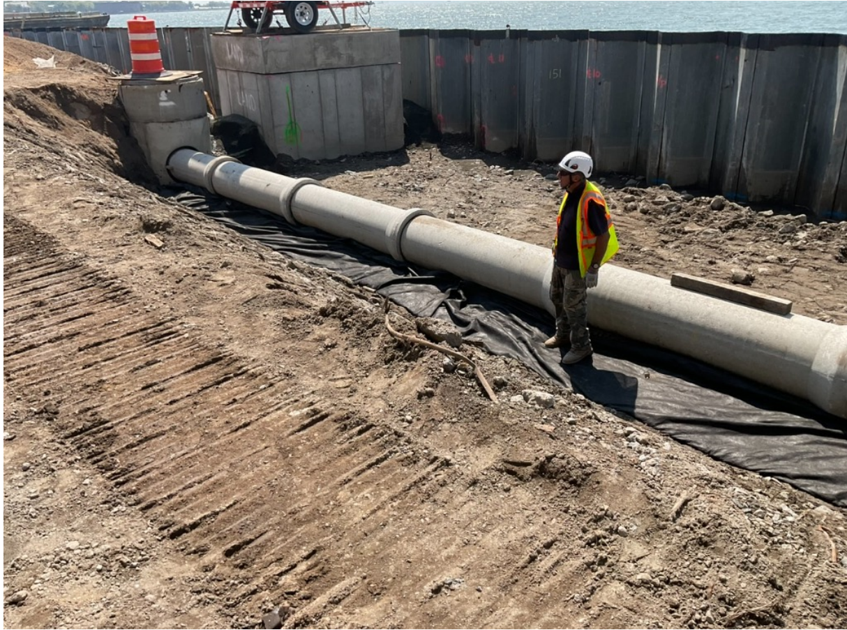
August 2024 – Storm Drainage Structure & Pipe Installation
