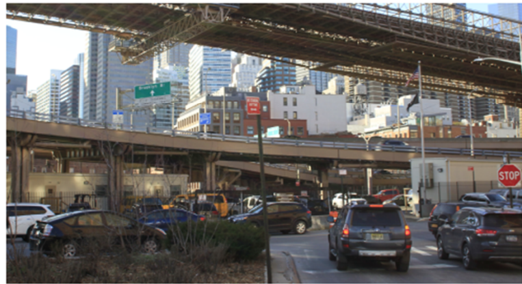
3. VIEW LOOKING WEST FROM SLIP STREET
