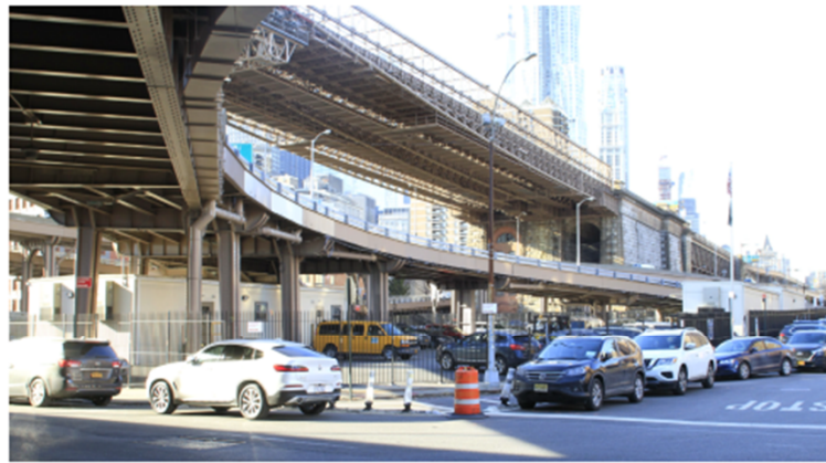
2. VIEW LOOKING NORTH FROM SOUTH STREET
