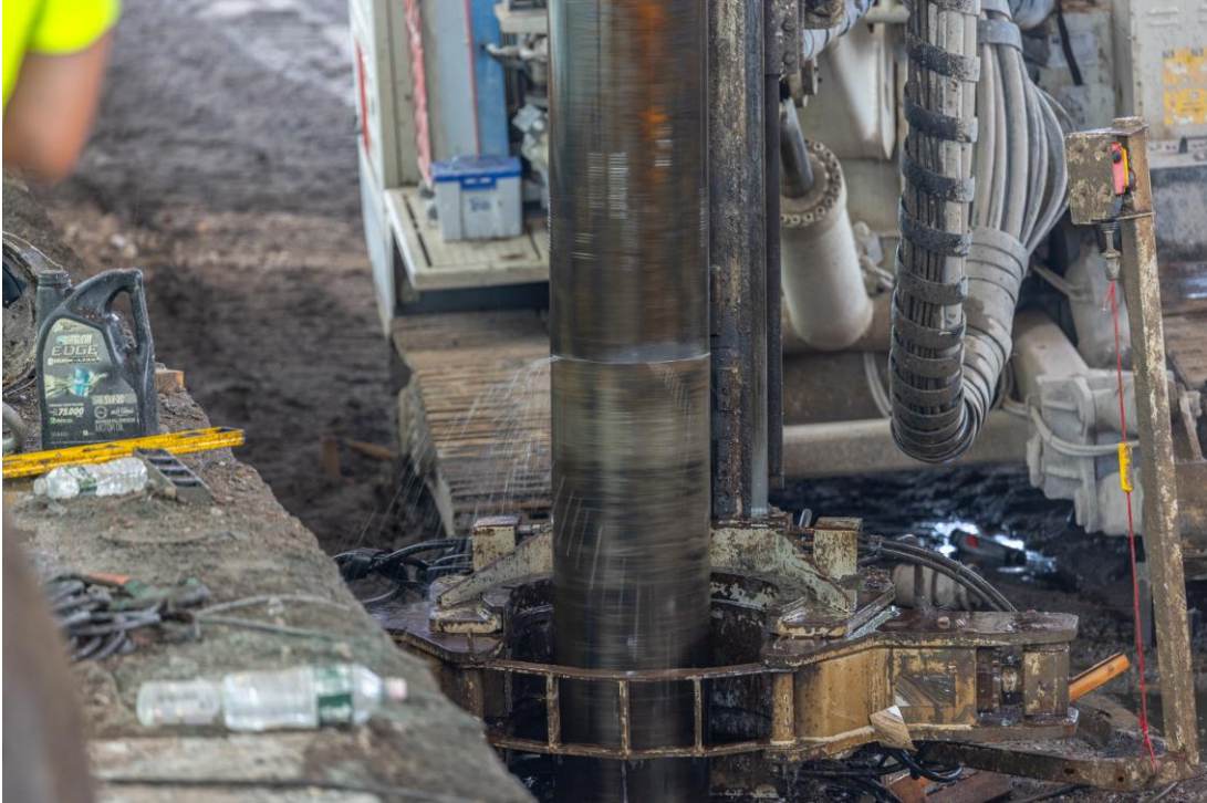
Micropile Installation – September 2023
