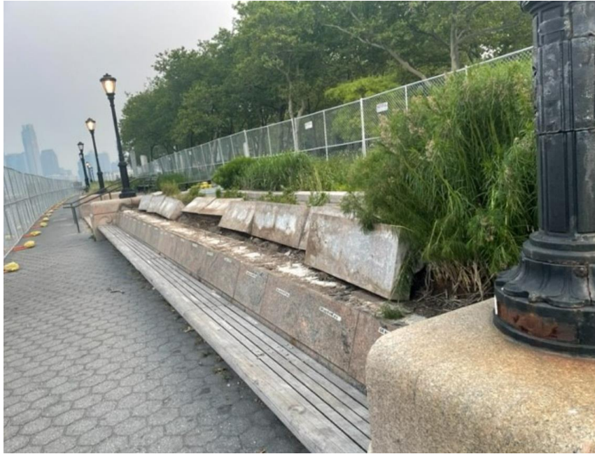
Early Salvage Operations In progress Along the southern end of the wharf
