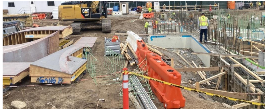
Foundation Work – Wagner Park Pavilion
