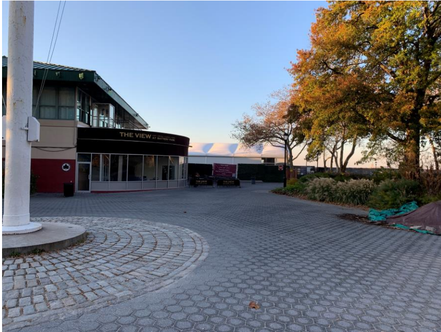
Temporary Security Tent Front view looking towards the restaurant entrance
