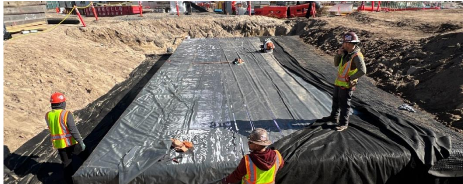
Cistern Installation – Wagner Park
