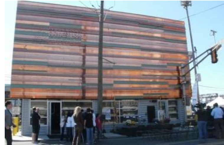
Pump Station in Hoboken, NJ Source: NJ.com
