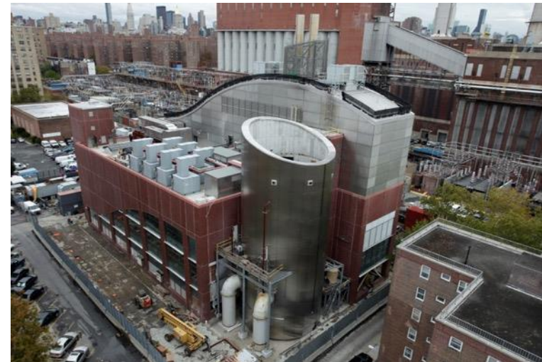
Manhattan Pump Station
