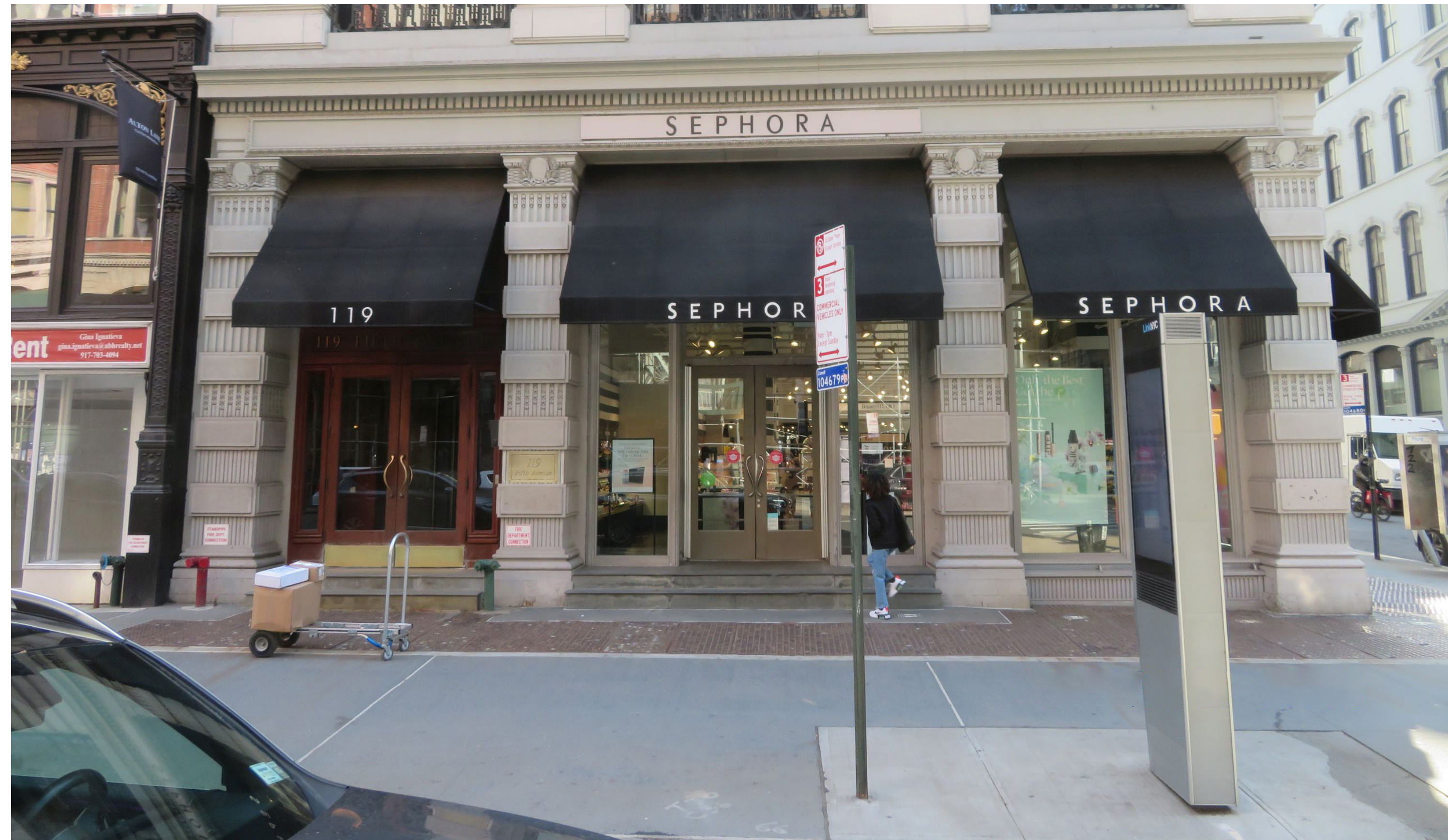
EXISTING CORNER AT 5TH AVE & EAST 19TH ST
