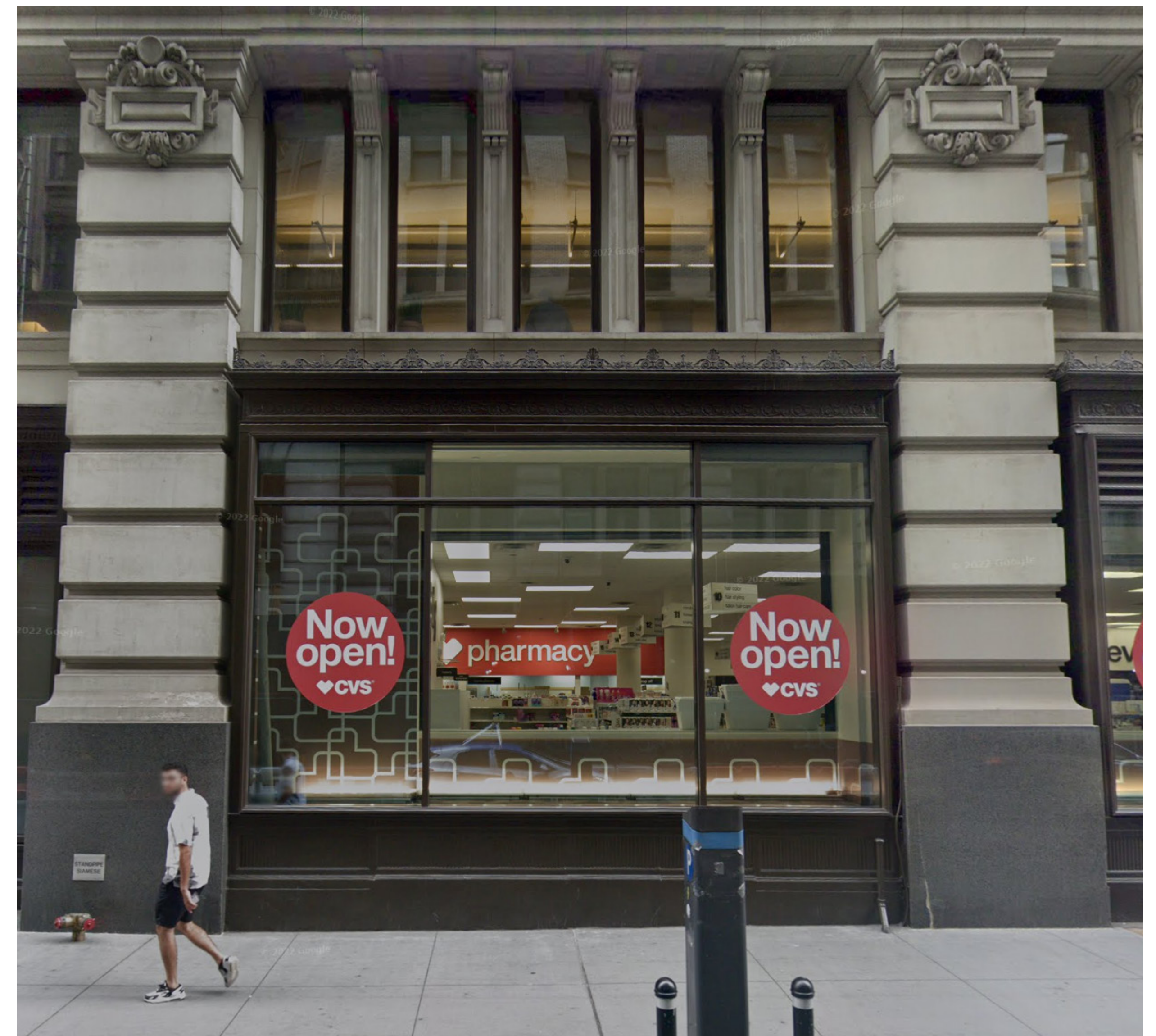
CVS WINDOW BAY ON WEST 18TH STREET
