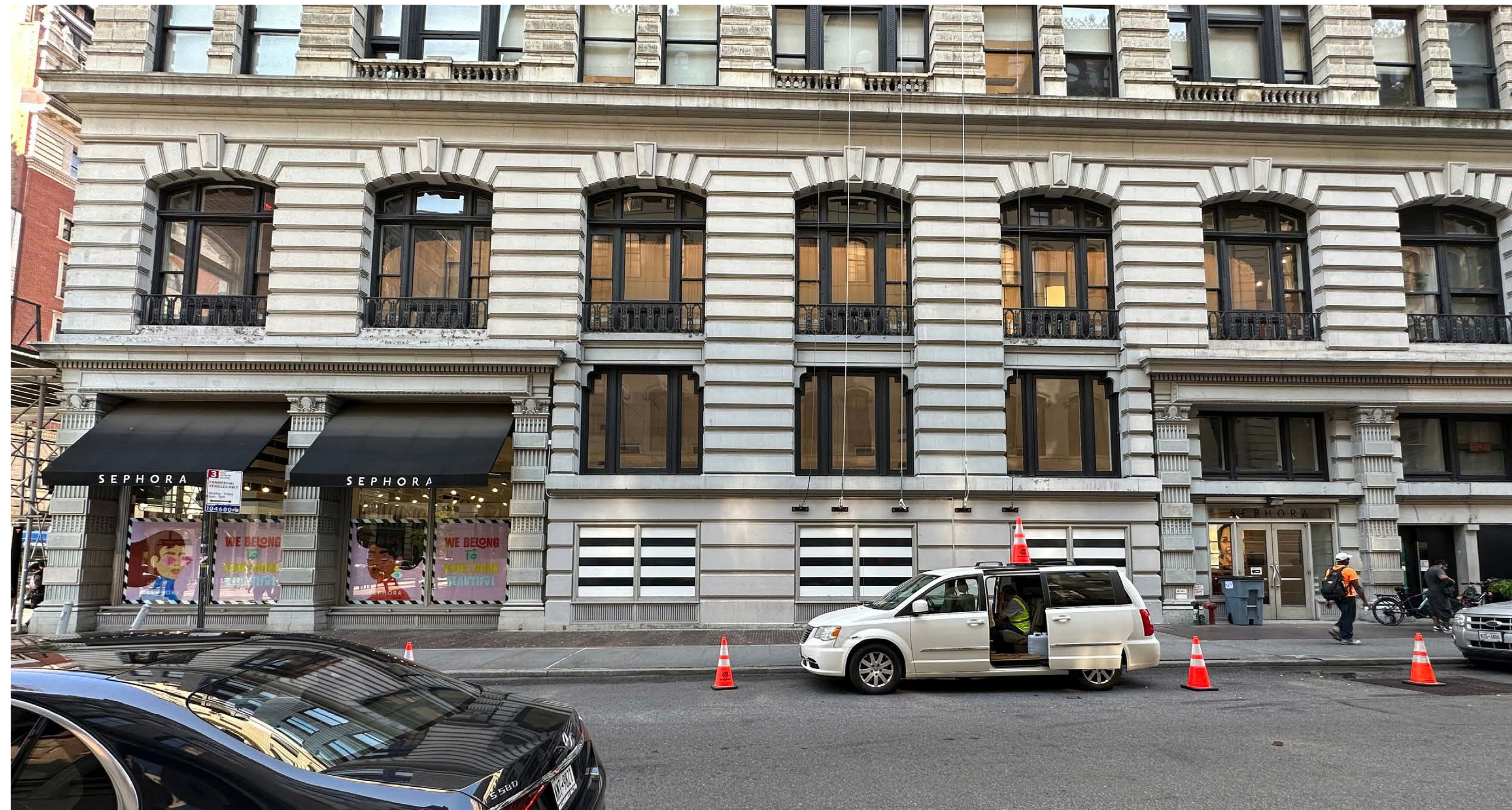
EXISTING FACADE AT EAST 19TH ST
