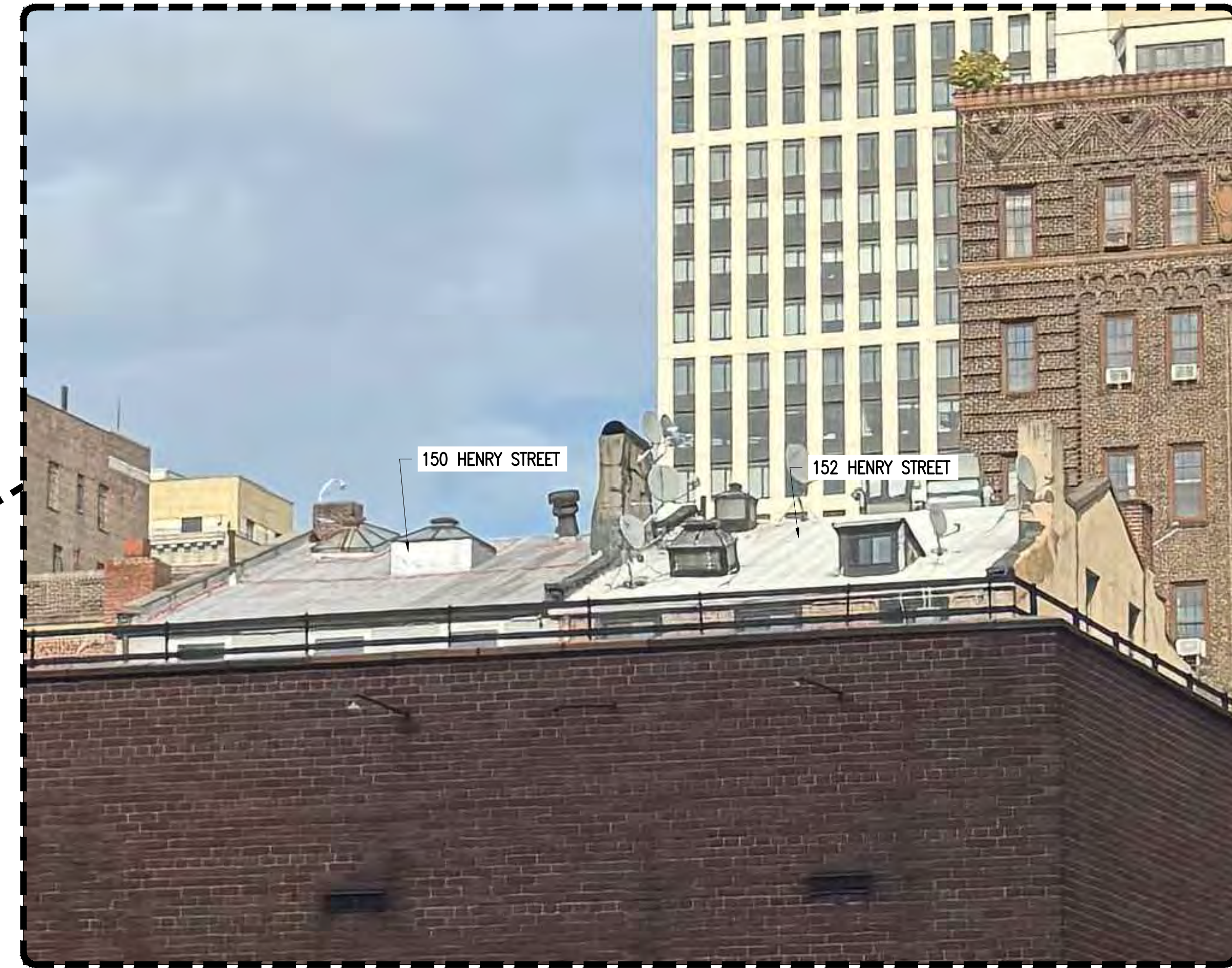
3 PHOTO OF MOCK-UP AT 150 HENRY STREET - ZOOMED IN LPC-6 NOT TO SCALE
