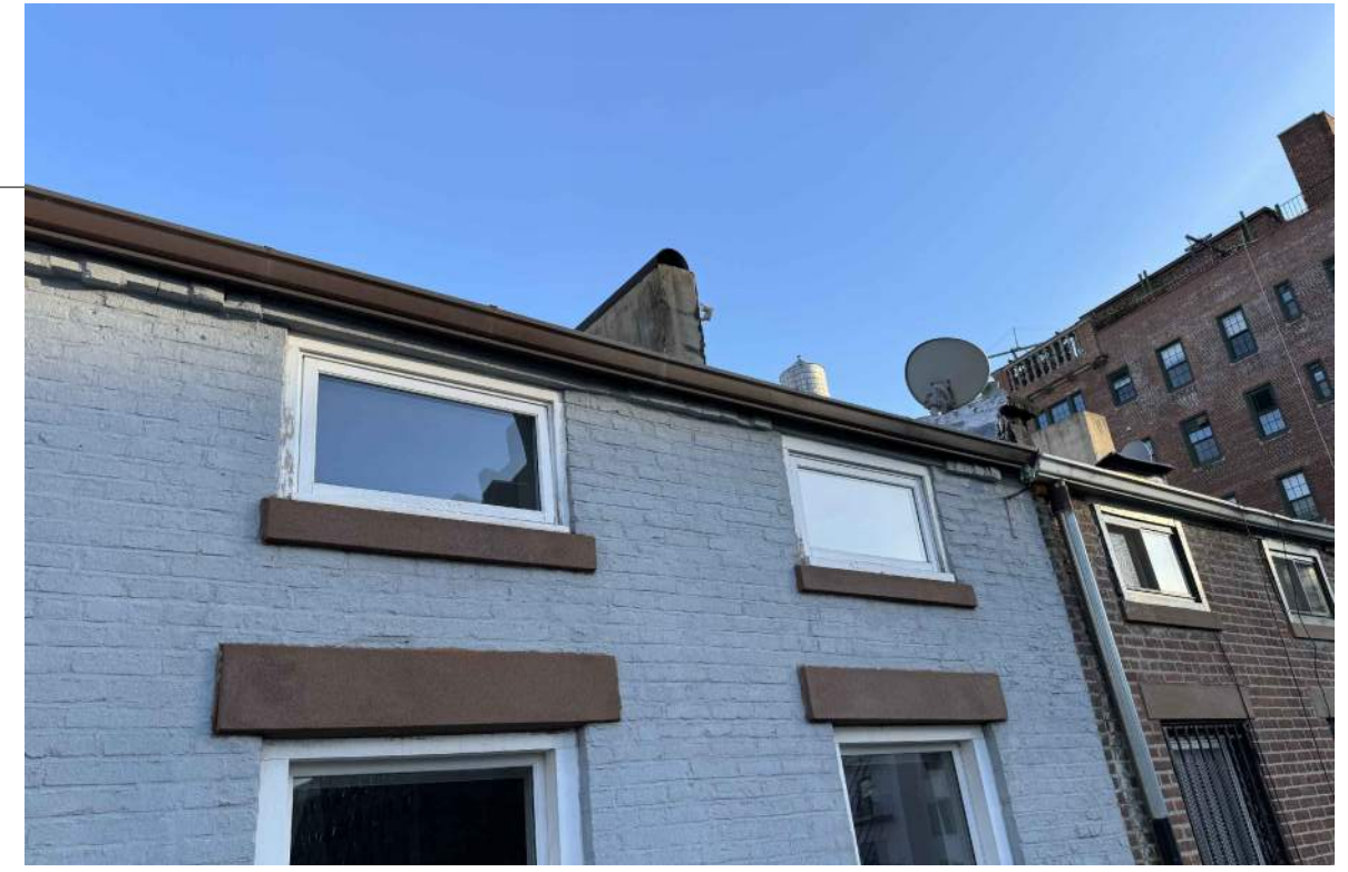
EXISTING CONDITION - REAR CORNICE
