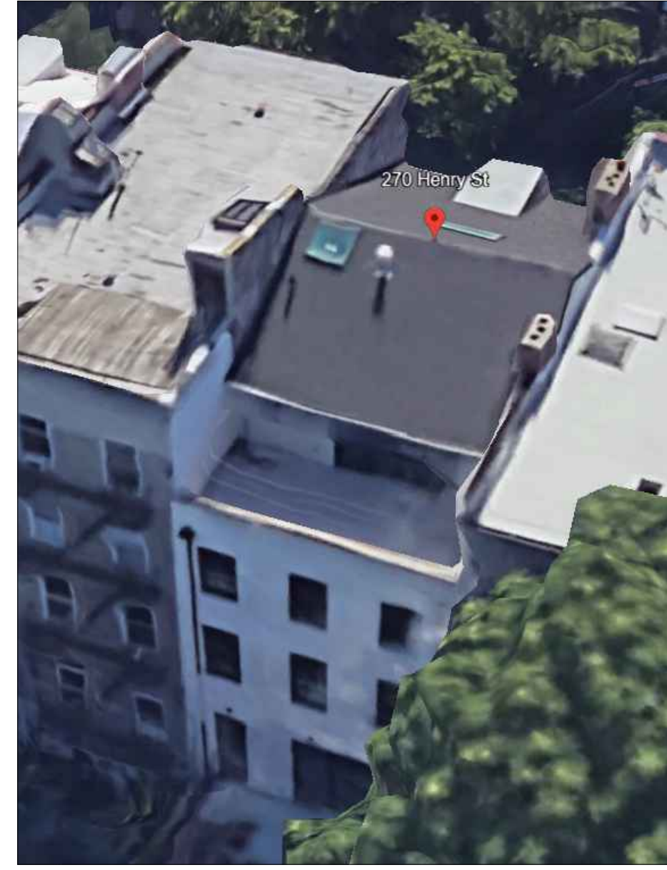
270 HENRY STREET, FULL WIDTH TERRACE REAR ROOF
