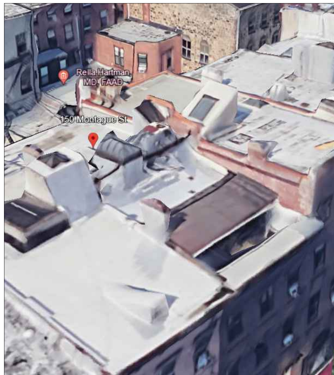
150 MONTAGUE STREET, FULL WIDTH CUT OUT AT FRONT ROOF
