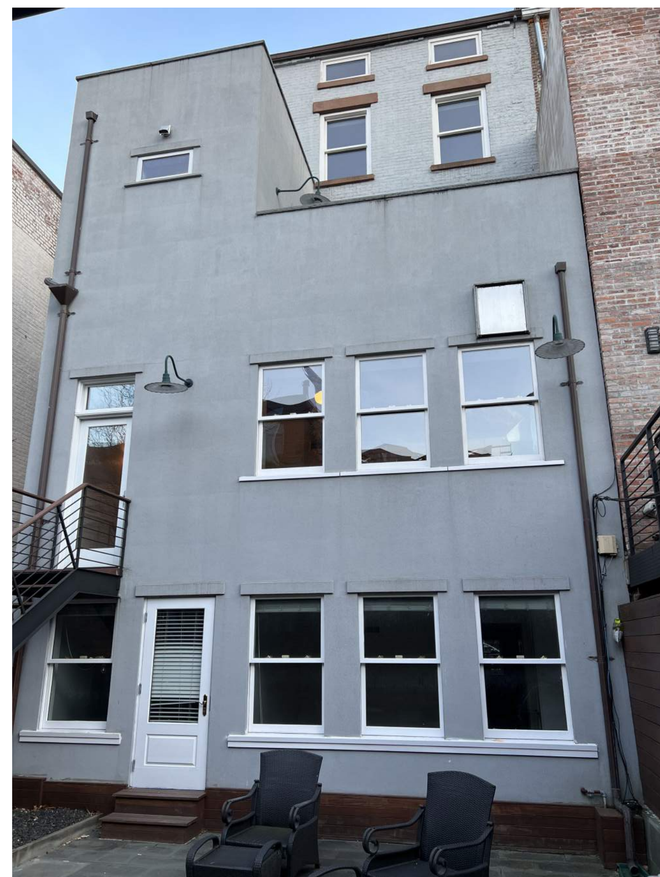
EXISTING REAR FACADE PHOTO
