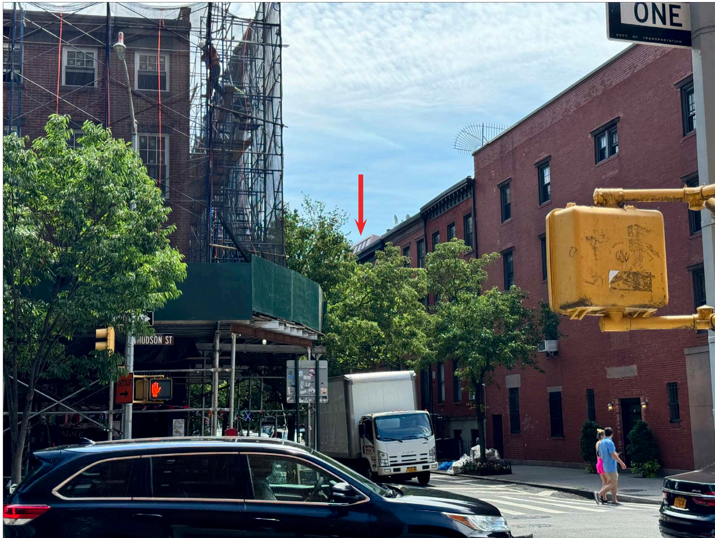
C VIEW FROM NORTH-WEST CORNER OF JANE STREET AND HUDSON STREET
