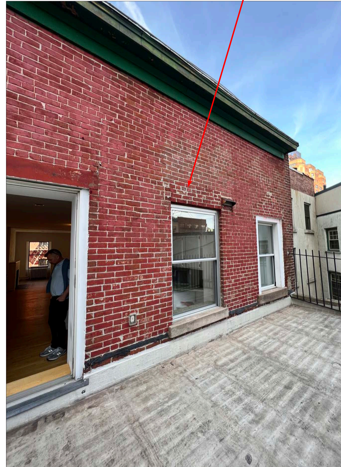
UPPER PORTION OF REAR FACADE
