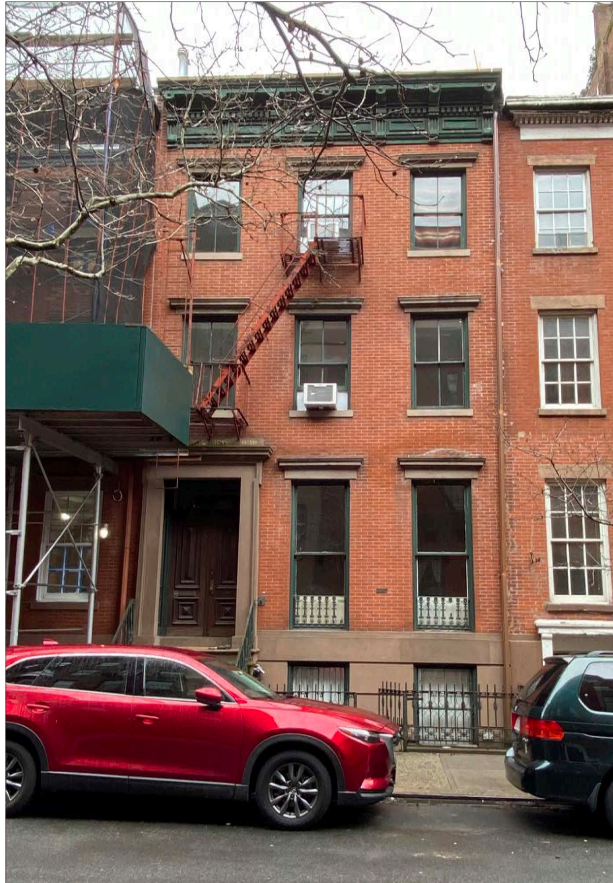
FRONT (NORTH) FACADE
