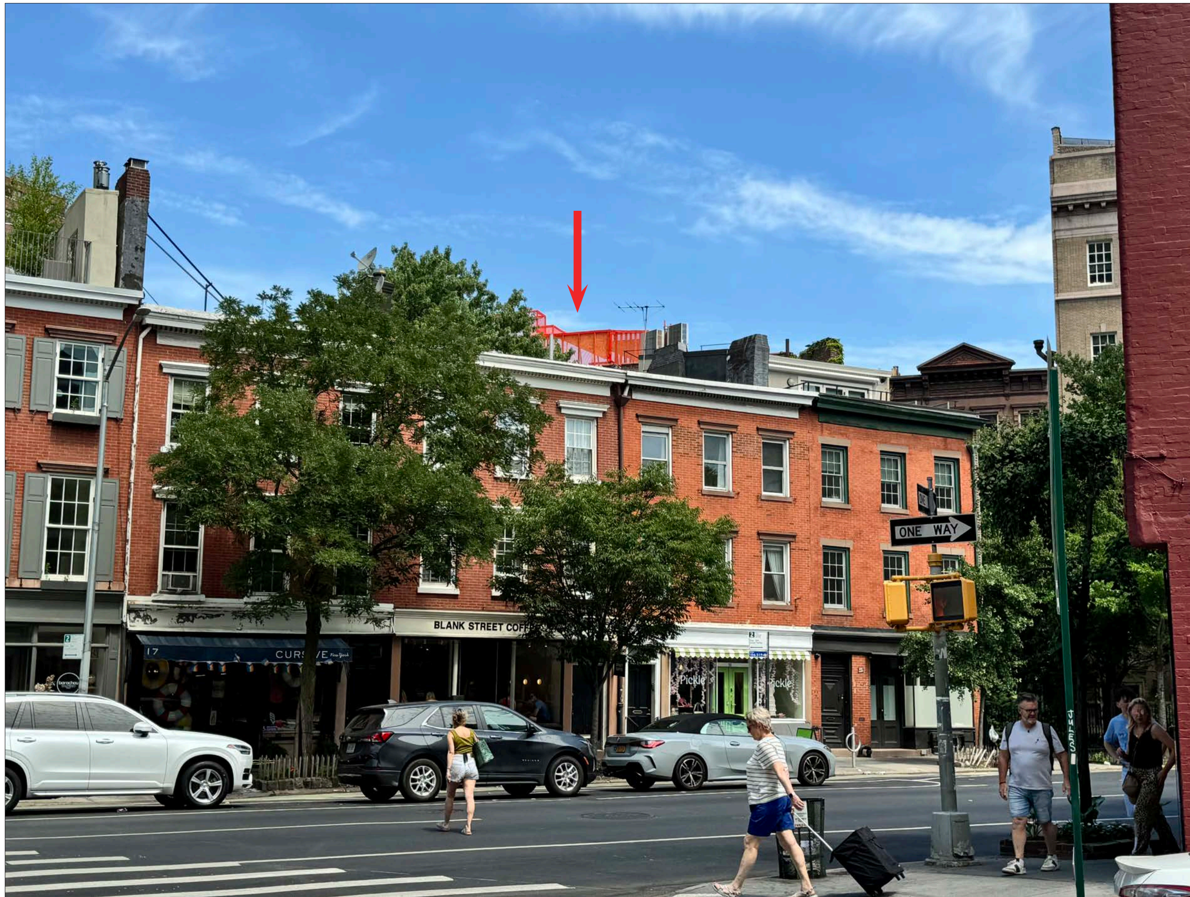
B VIEW FROM 302 WEST 12TH STREET SERVICE ENTRANCE (CHASE BANK ATM)
