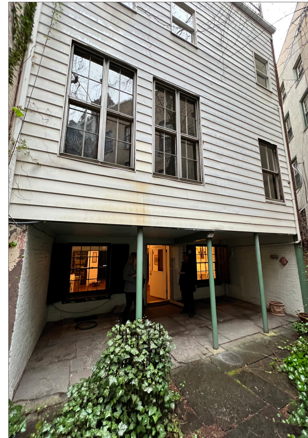
REAR (SOUTH) FACADE
