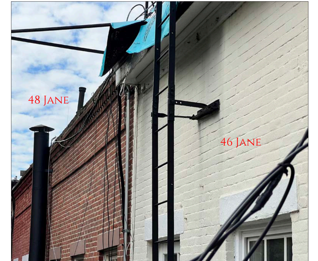
REAR FACADE CORNICES
