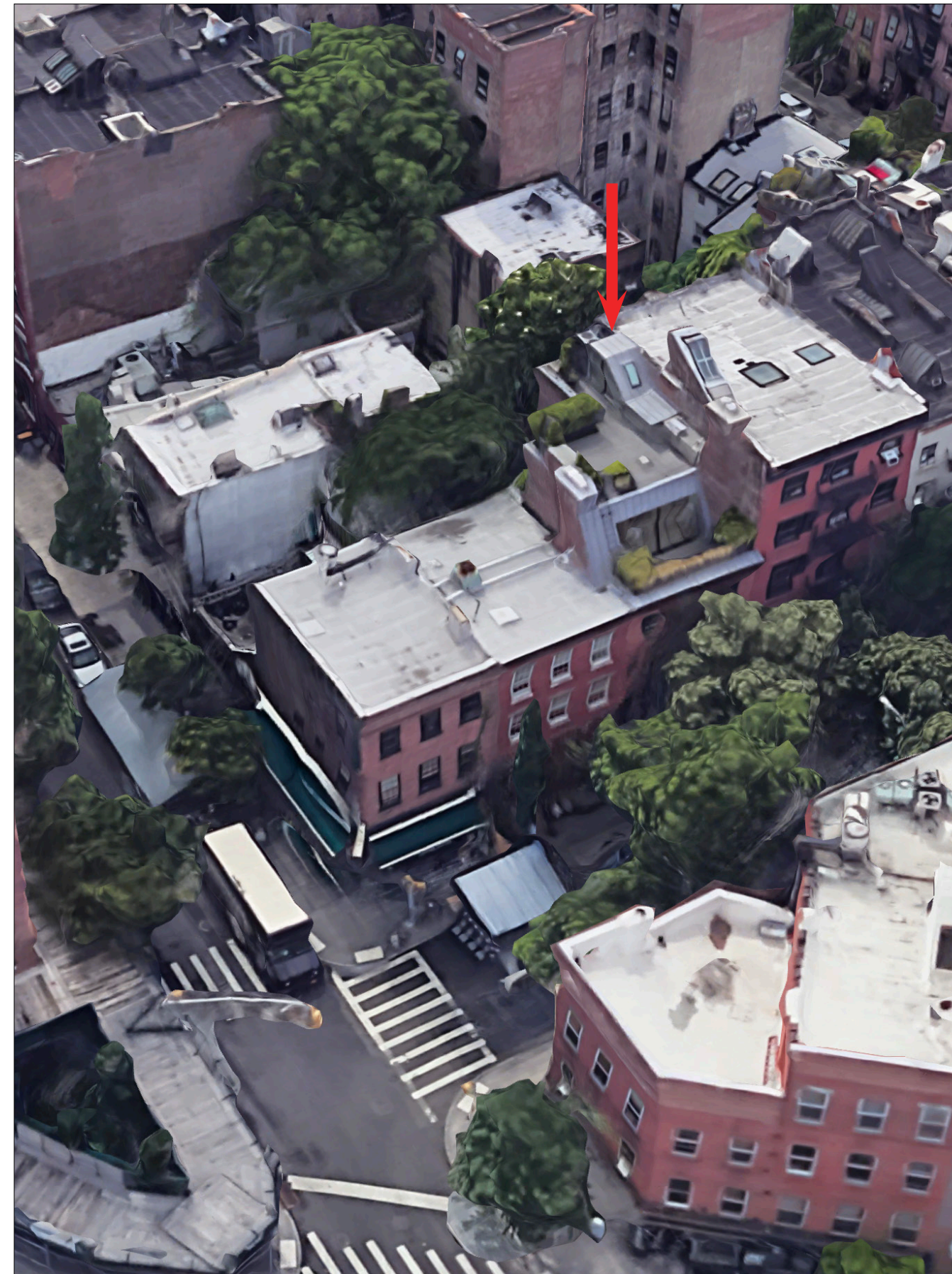
327 WEST 4TH STREET AERIAL VIEW (LPC-19-11323)
