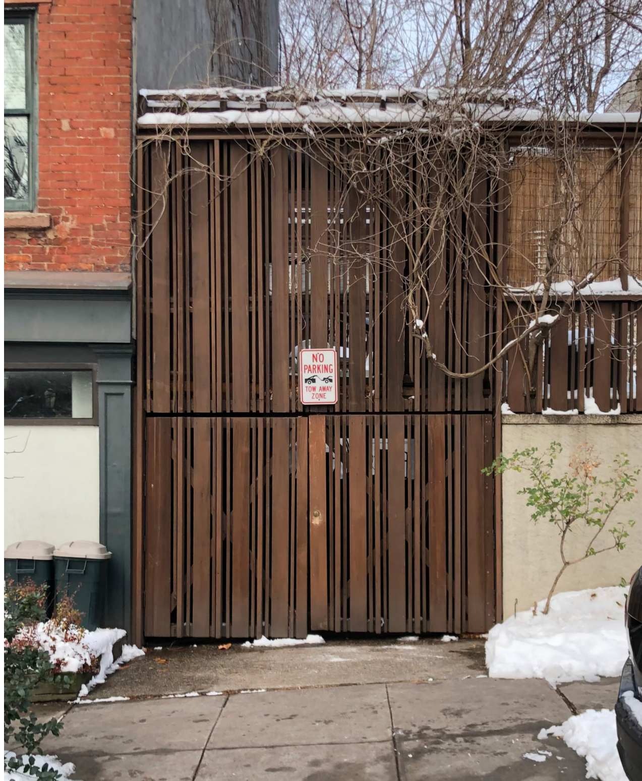
View from State Street - 2023 Fence Condition
