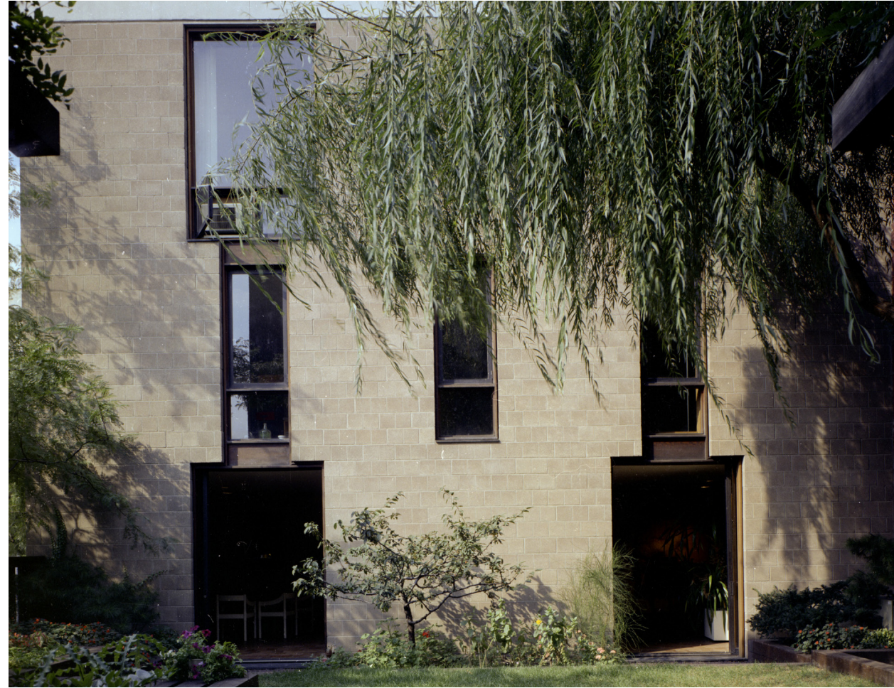
Rear Facade (unknown date)
