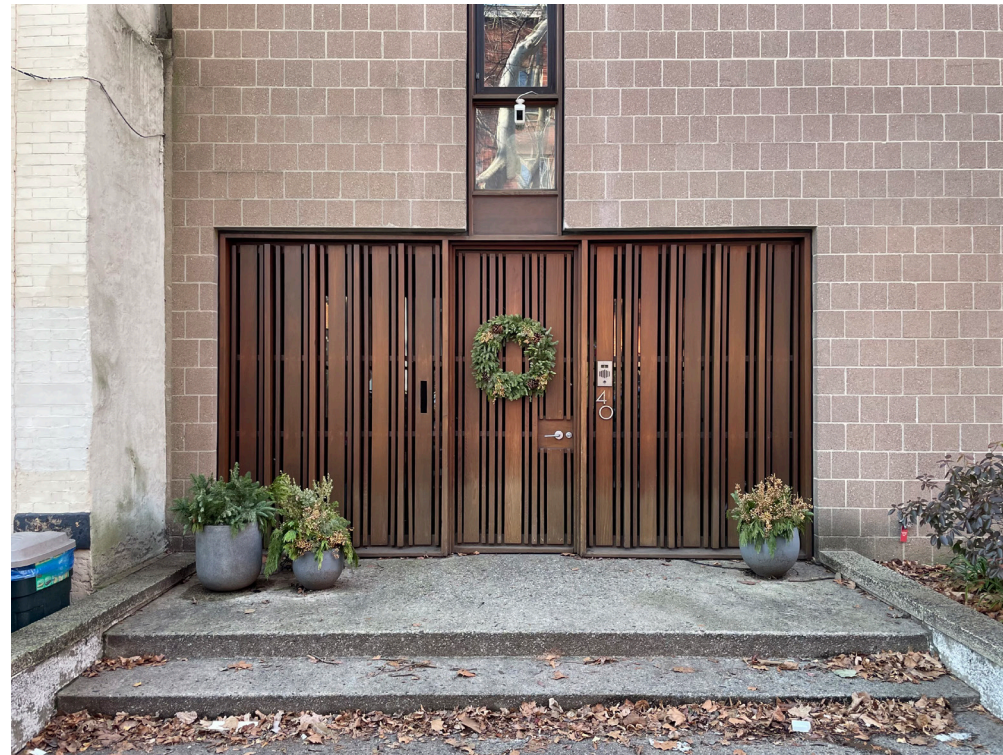
Fence / Screen at 44 Willow Place
