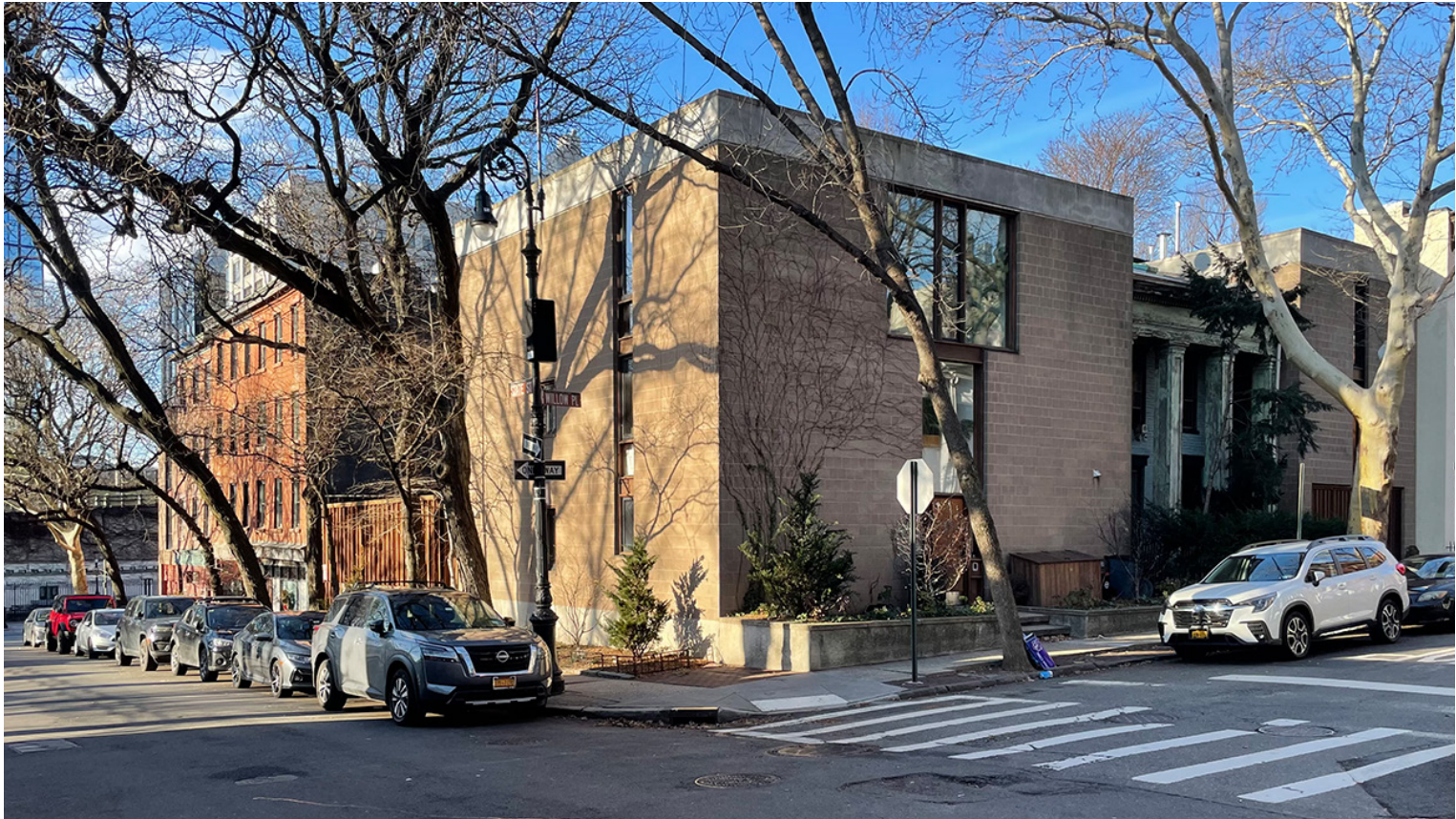
View from State Street - 2024 Fence Condition
