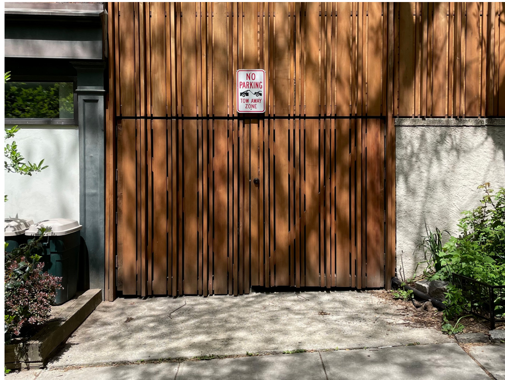
Fence / Screen at 48 Willow Place
