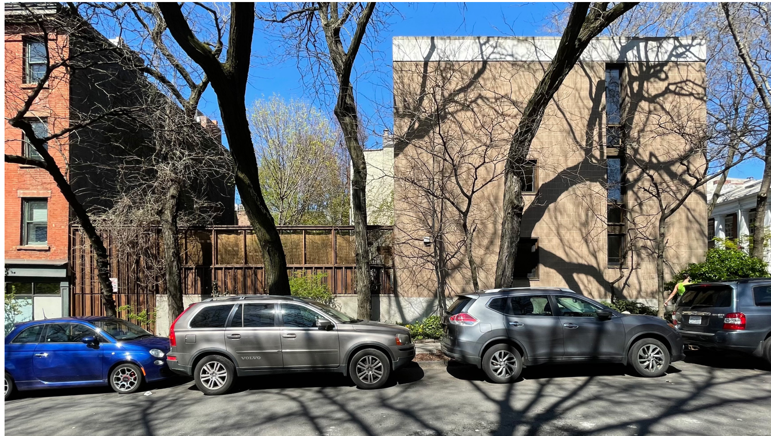
View from State Street - 2023 Fence Condition
