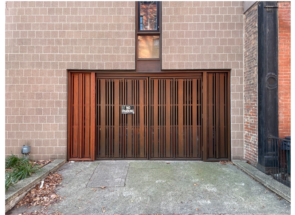
Fence / Screen at 40 Willow Place
