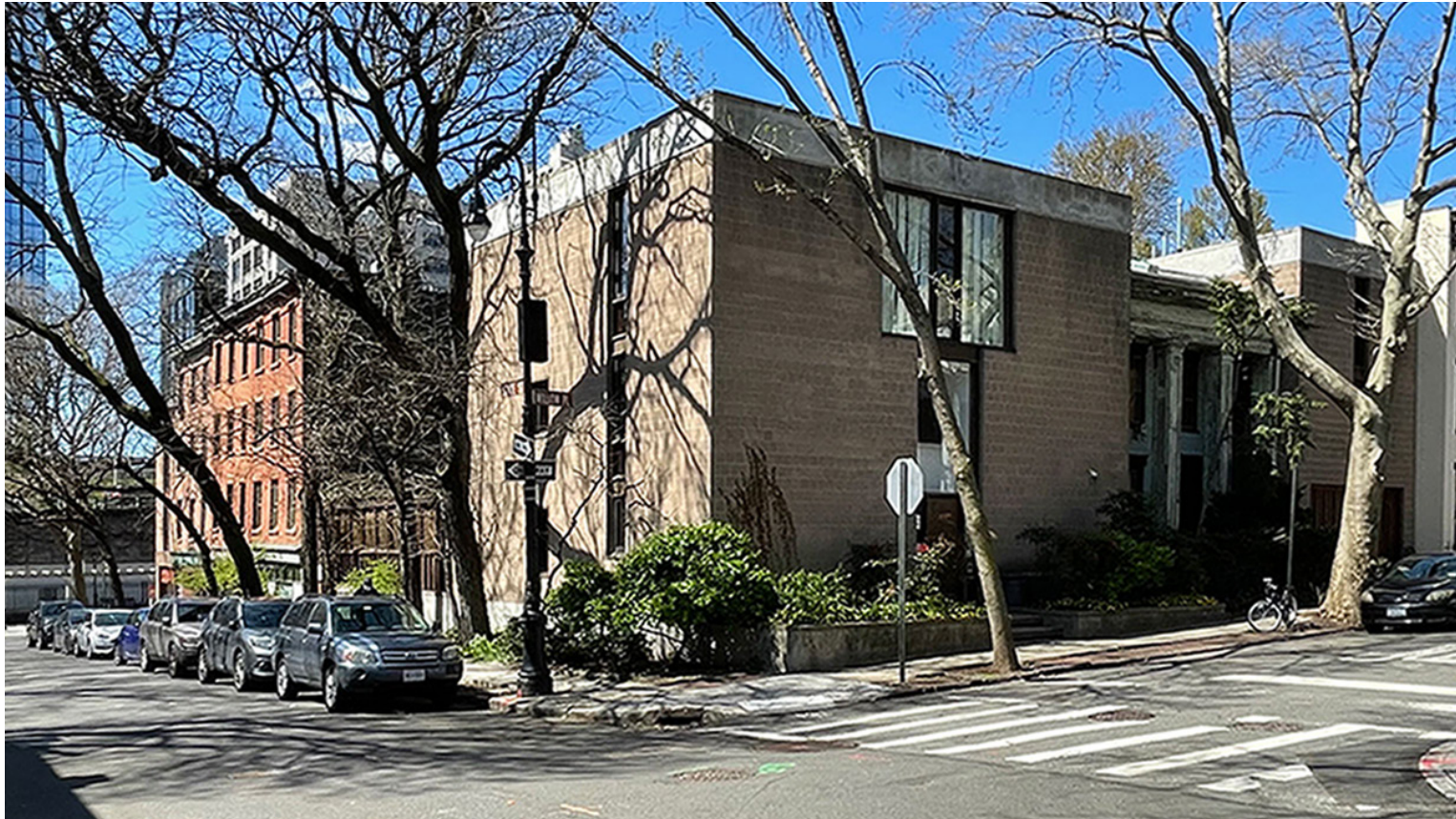
View from State Street - 2023 Fence Condition
