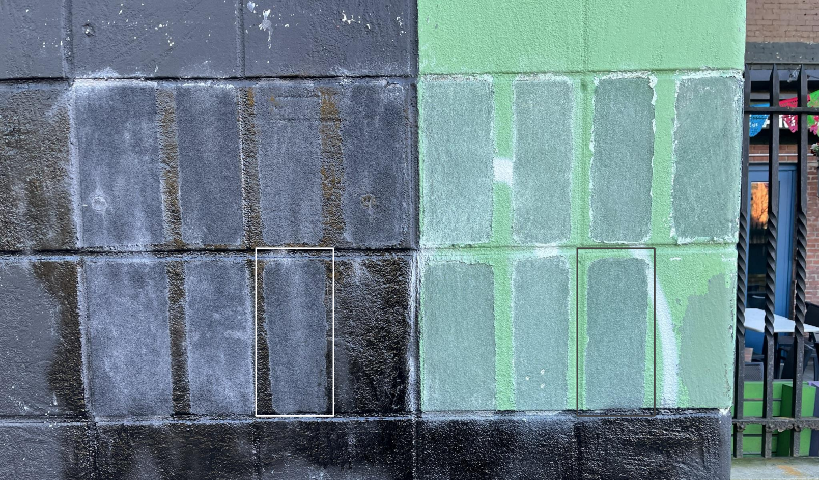
Two overnight applications of Cathedral Stone Light Duty Paint Remover
