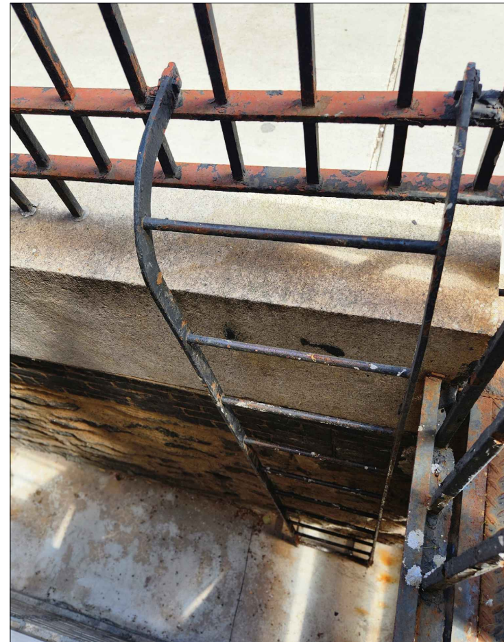
5 EXISTING AREAWAY SERVICE LADDER NOT TO SCALE
