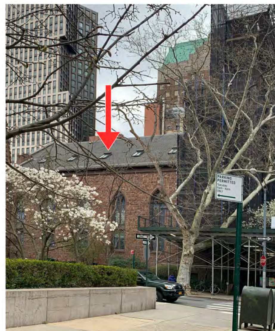
3. View from Pierrepont St. towards North-East Current Condition
