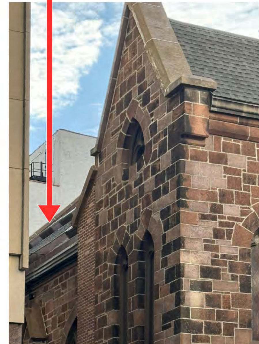
5. View from Remsen St. with visible Skylights
