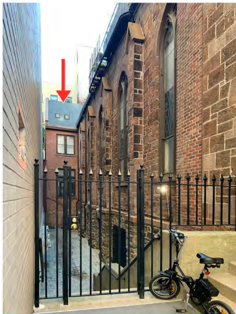
8 VIEW SOUTH FROM SPENCER MEWS Photo taken 12/2023 – Skylights Attic Roof visible
