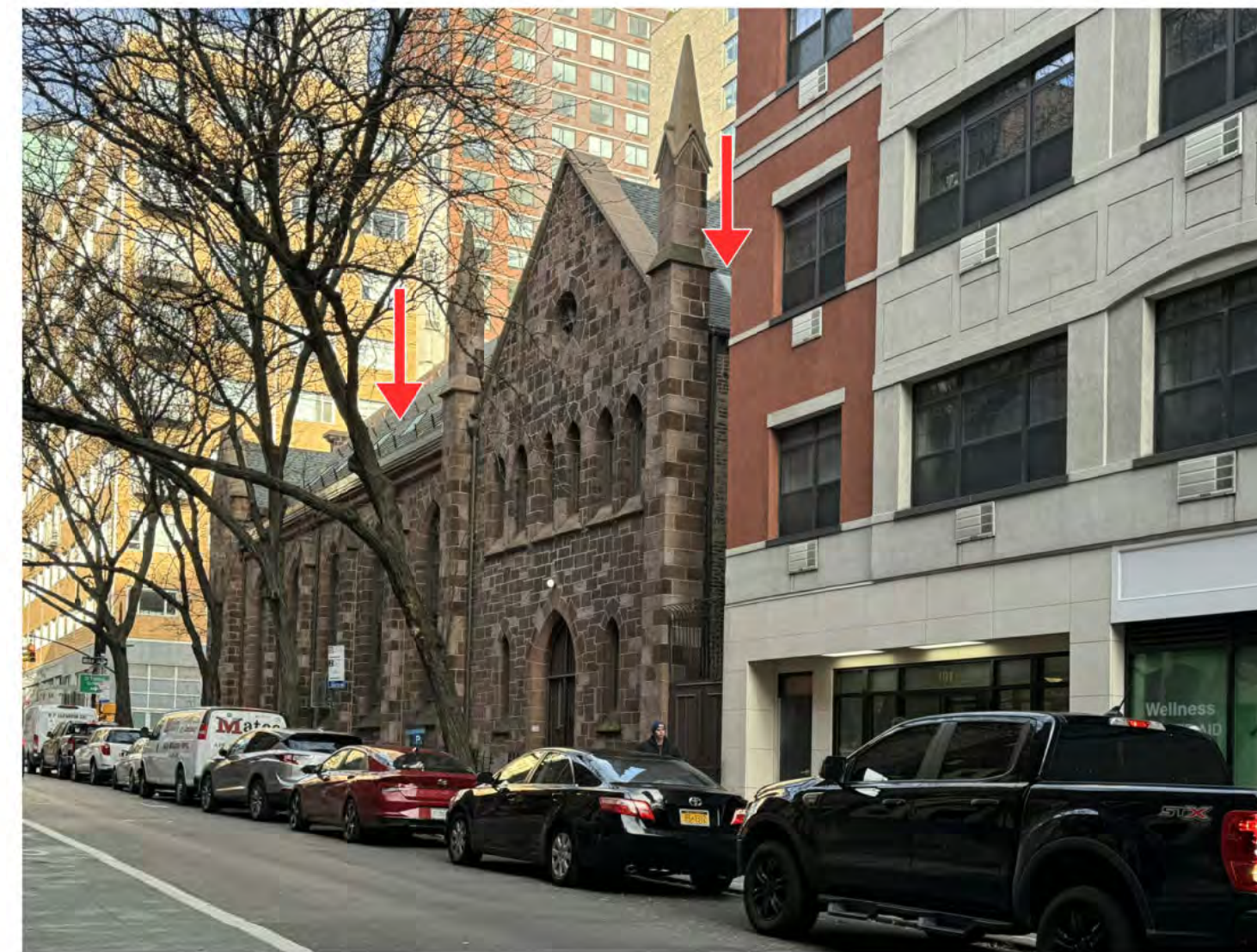
2 VIEW NORTHEAST FROM CLINTON ST. SIDEWALK Photo taken 12/2023 – Skylights visible
