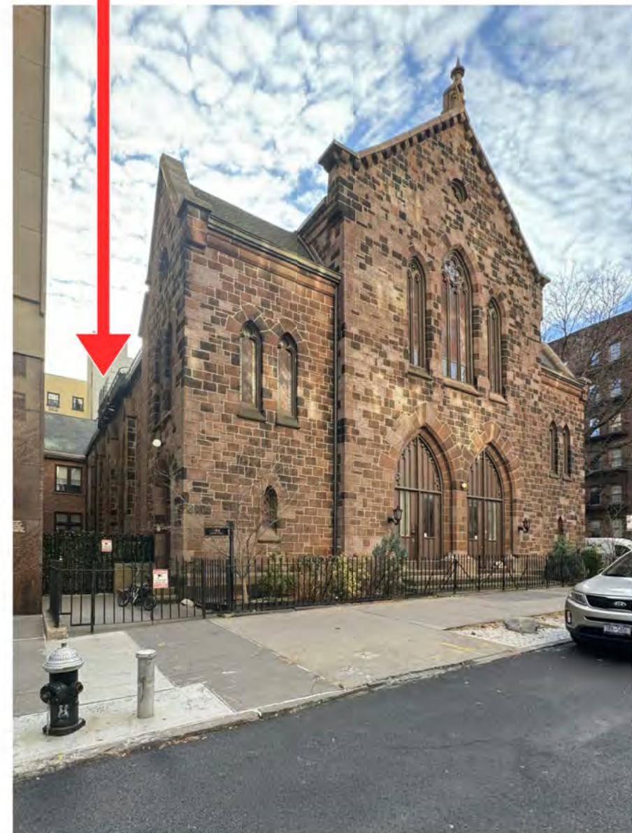
4. View from Remsen St. with visible Balcony
