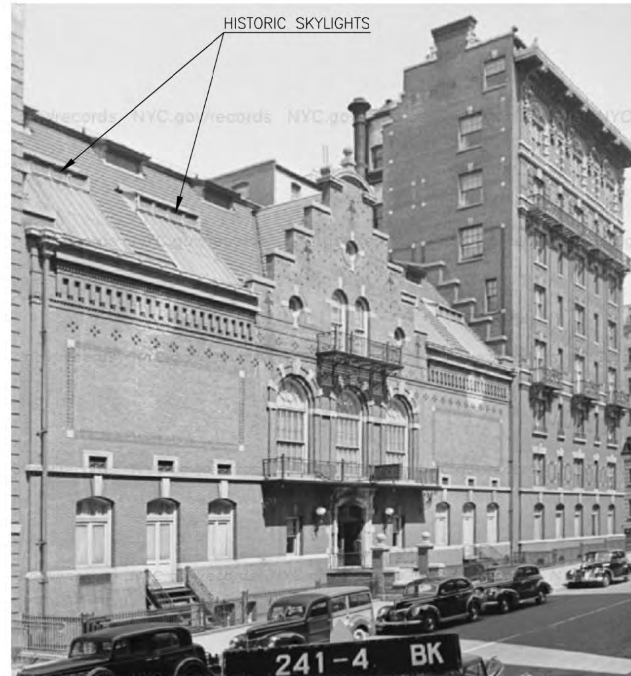
View from Montague St. looking North-East Showing Historic & Original Skylights
