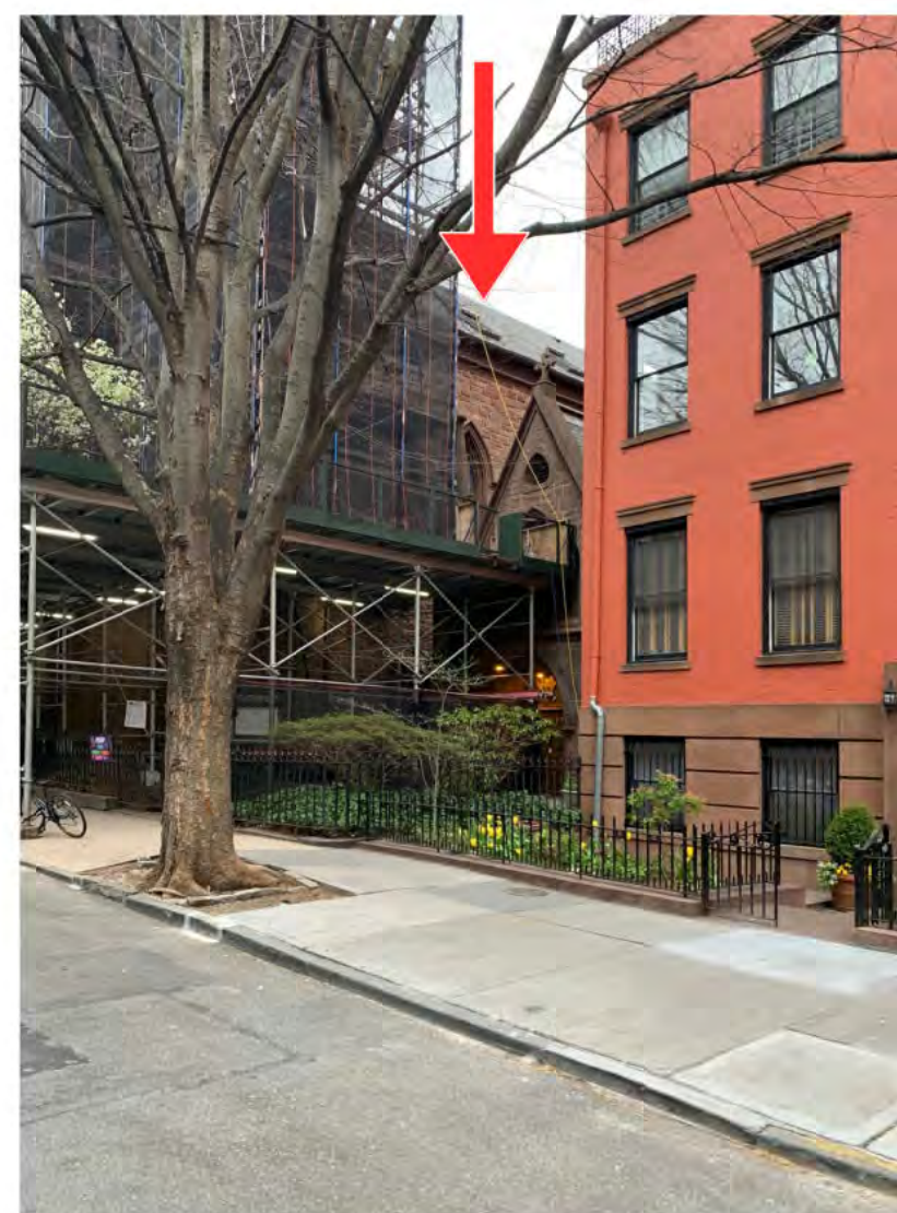
4. View from Pierrepont St. looking North-West, Current Condition
