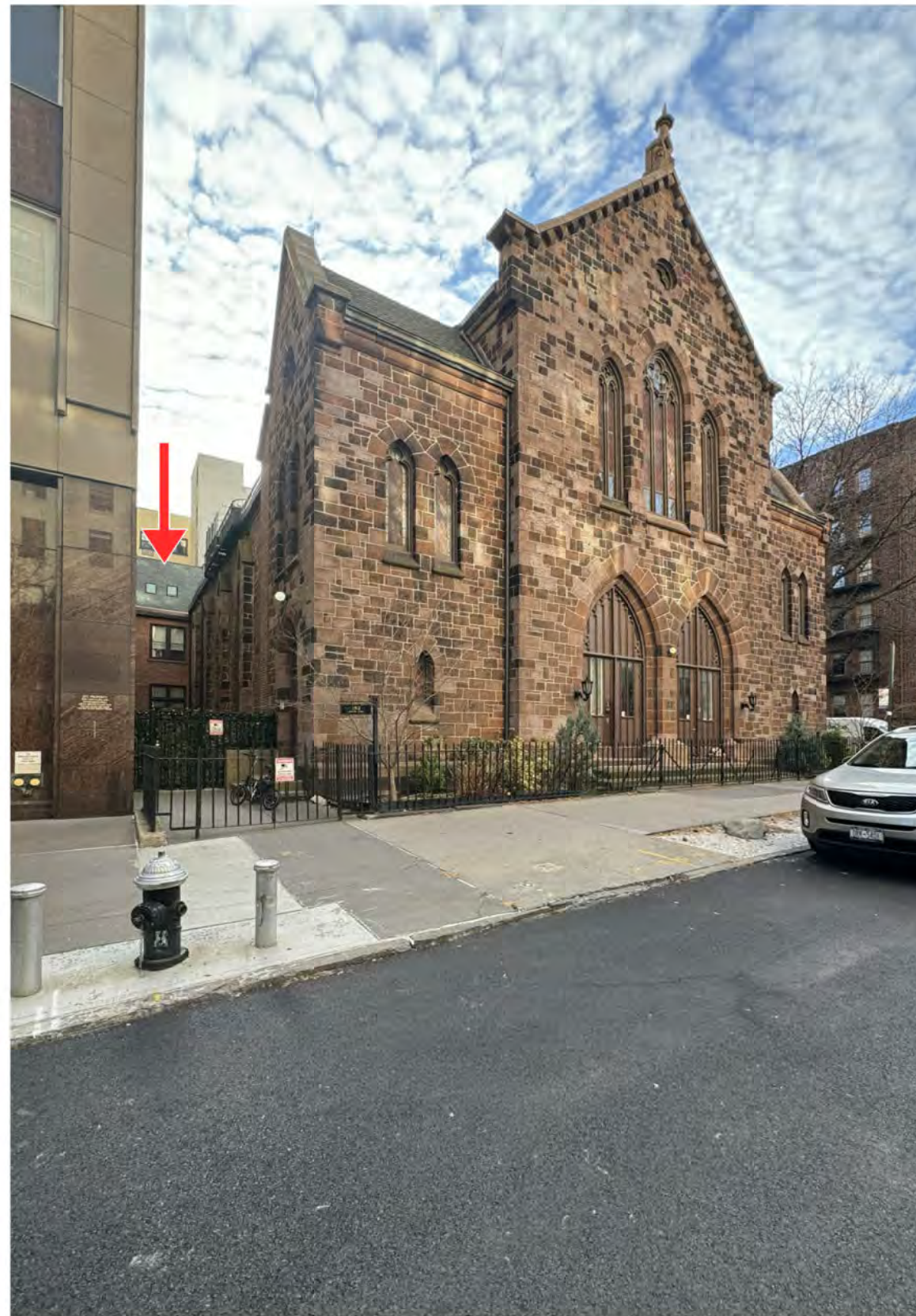
7 VIEW SW ON REMSEN Photo taken 12/2023 – Skylights Attic Roof visible
