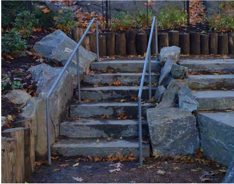
Granite steps at asphalt path
