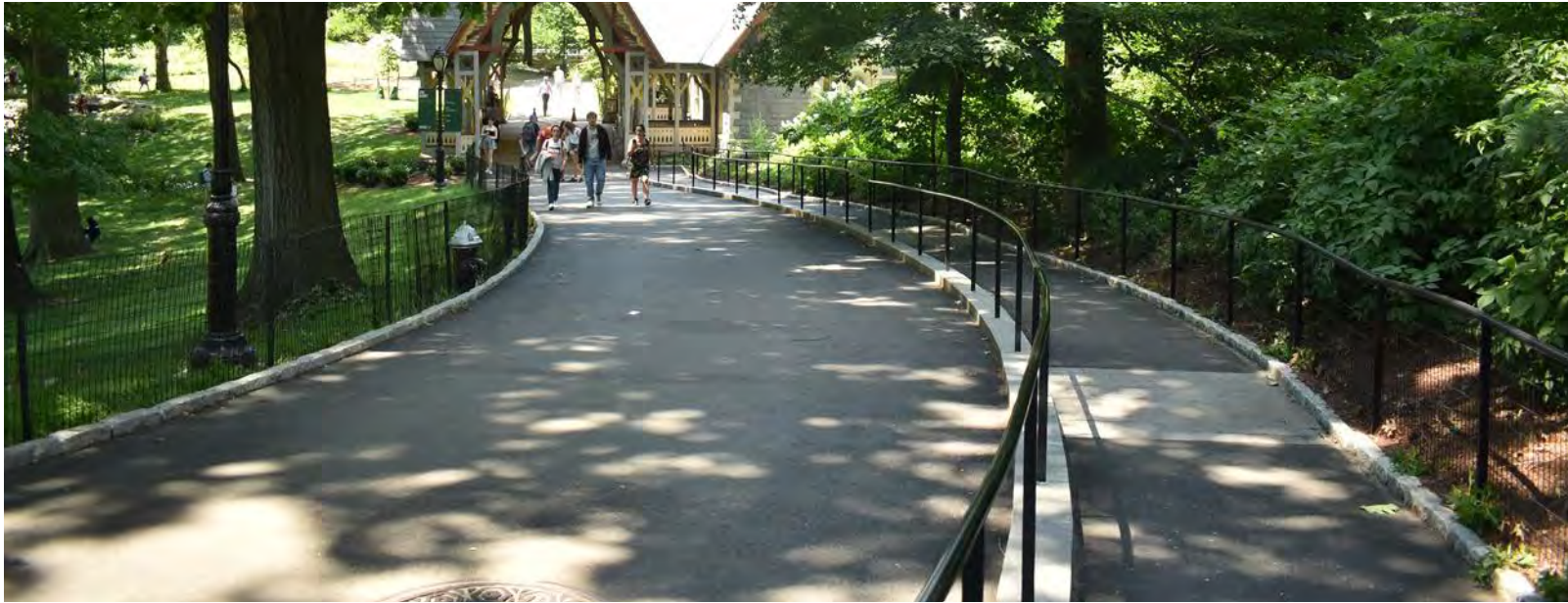
ADA accessible asphalt ramp adjacent to asphalt path - round steel handrail, painted black finish - rectangular asphalt block landings - granite curbing
