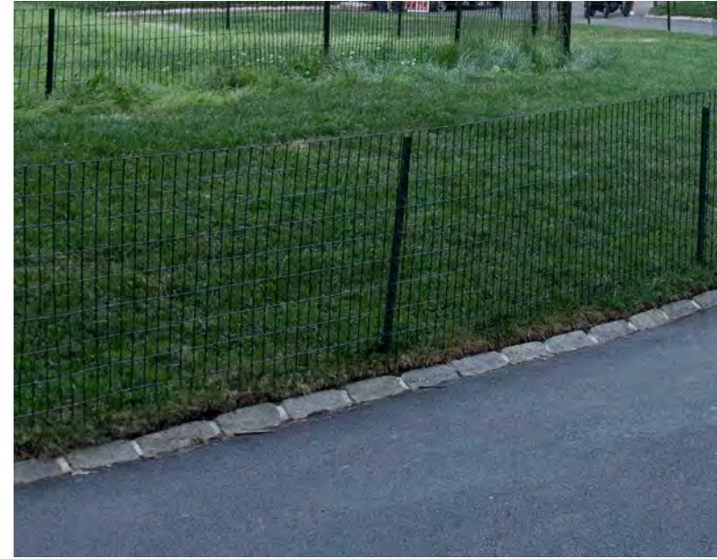
Asphalt paving with sloping granite block curb
