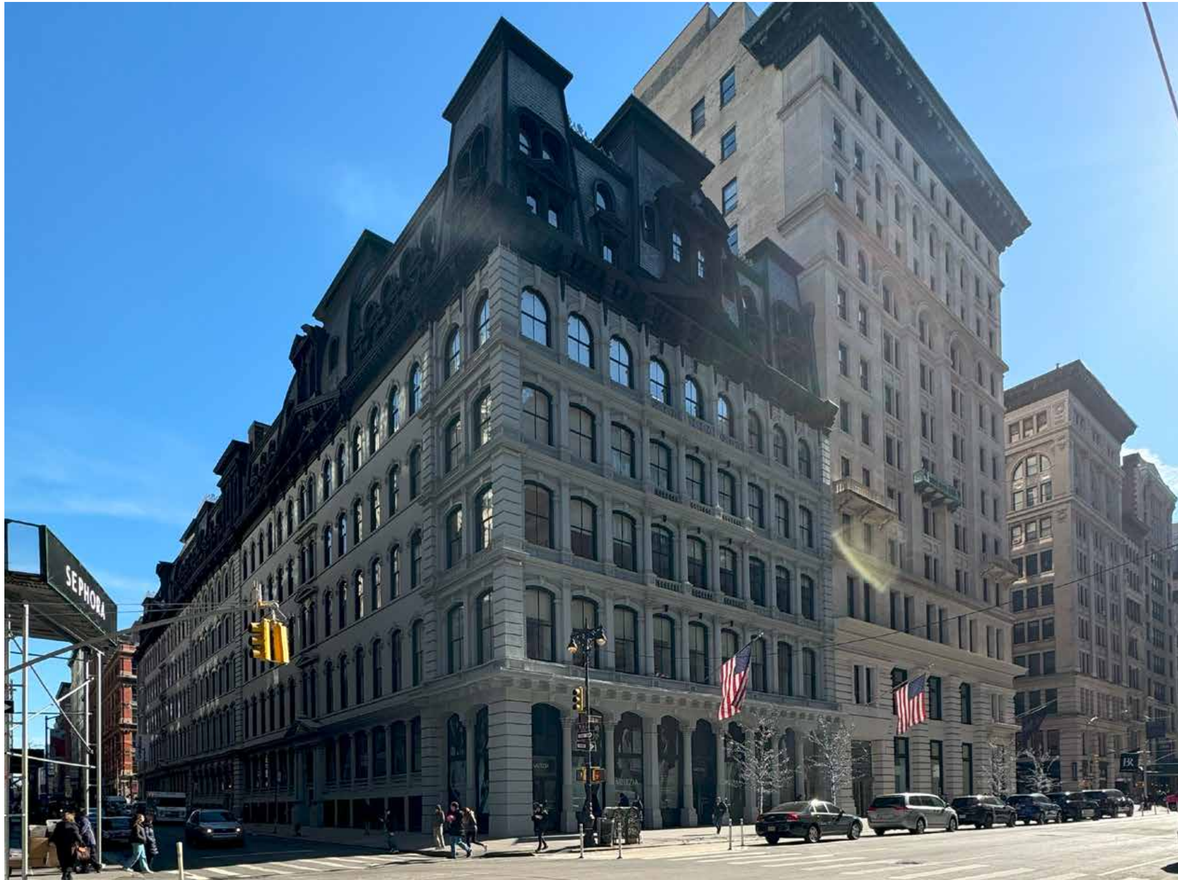
Existing Store Front
