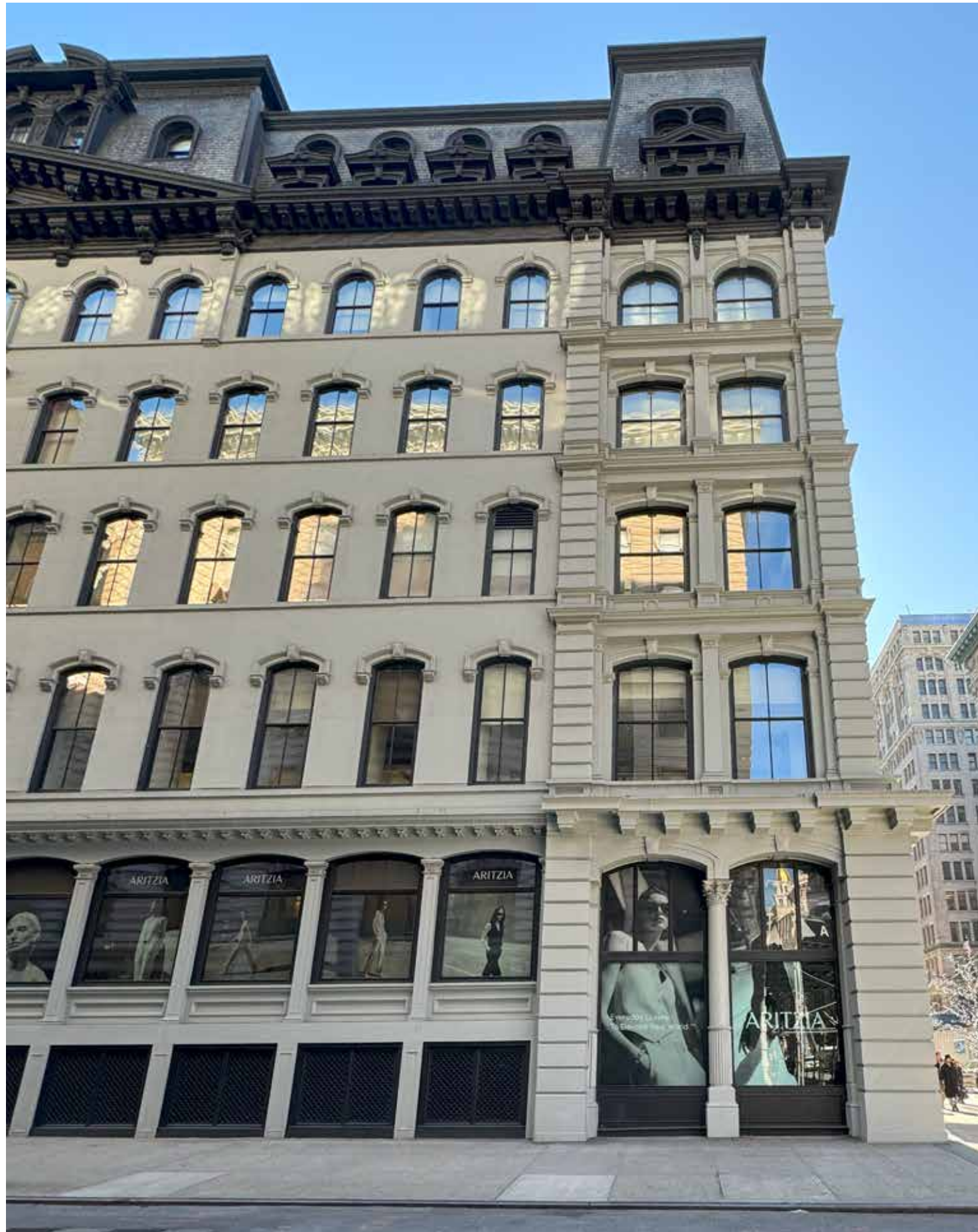
Existing Store Front
