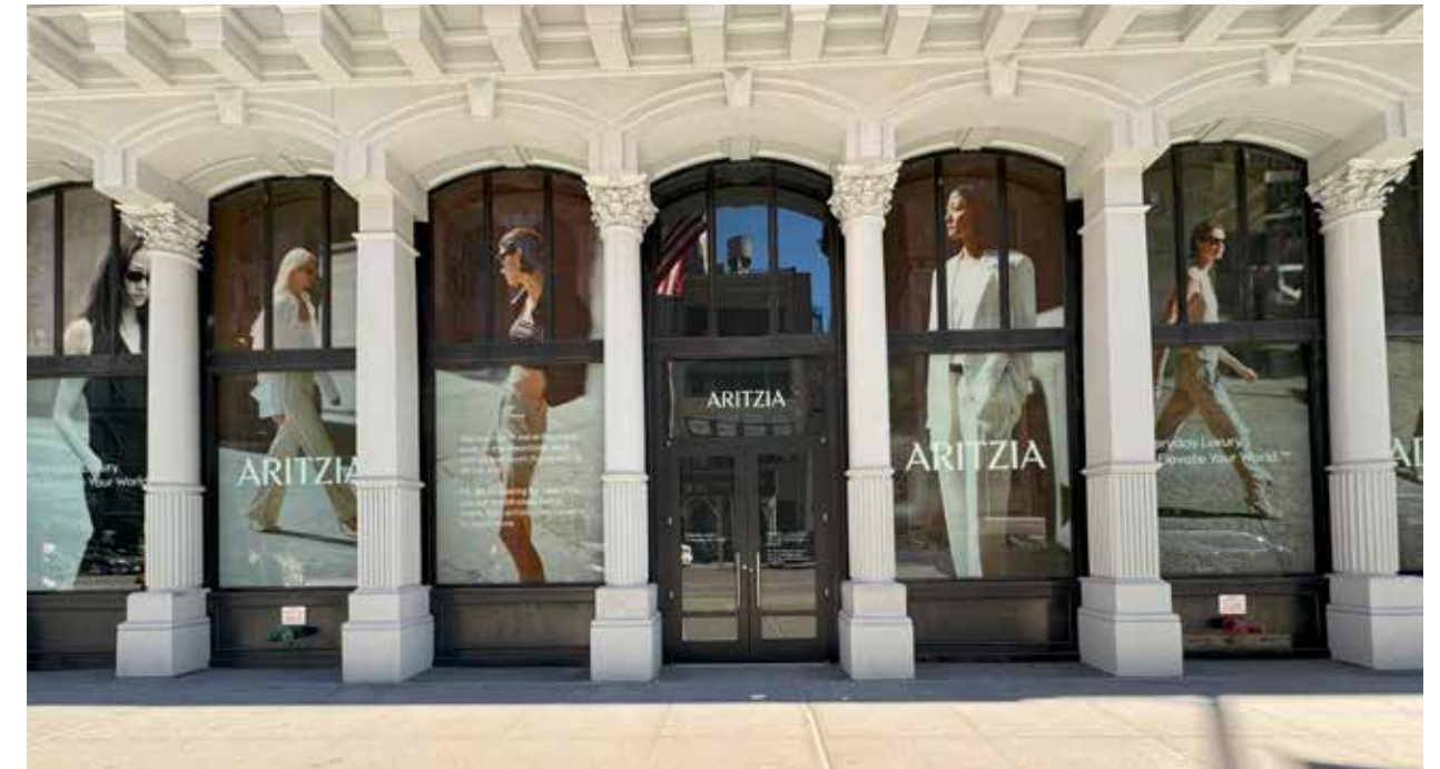
Existing Store Front
