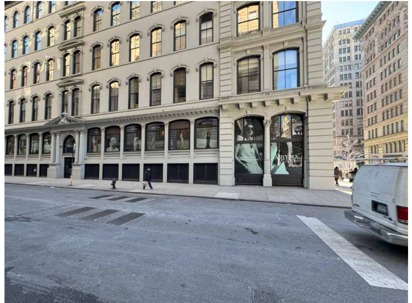
Existing Store Front
