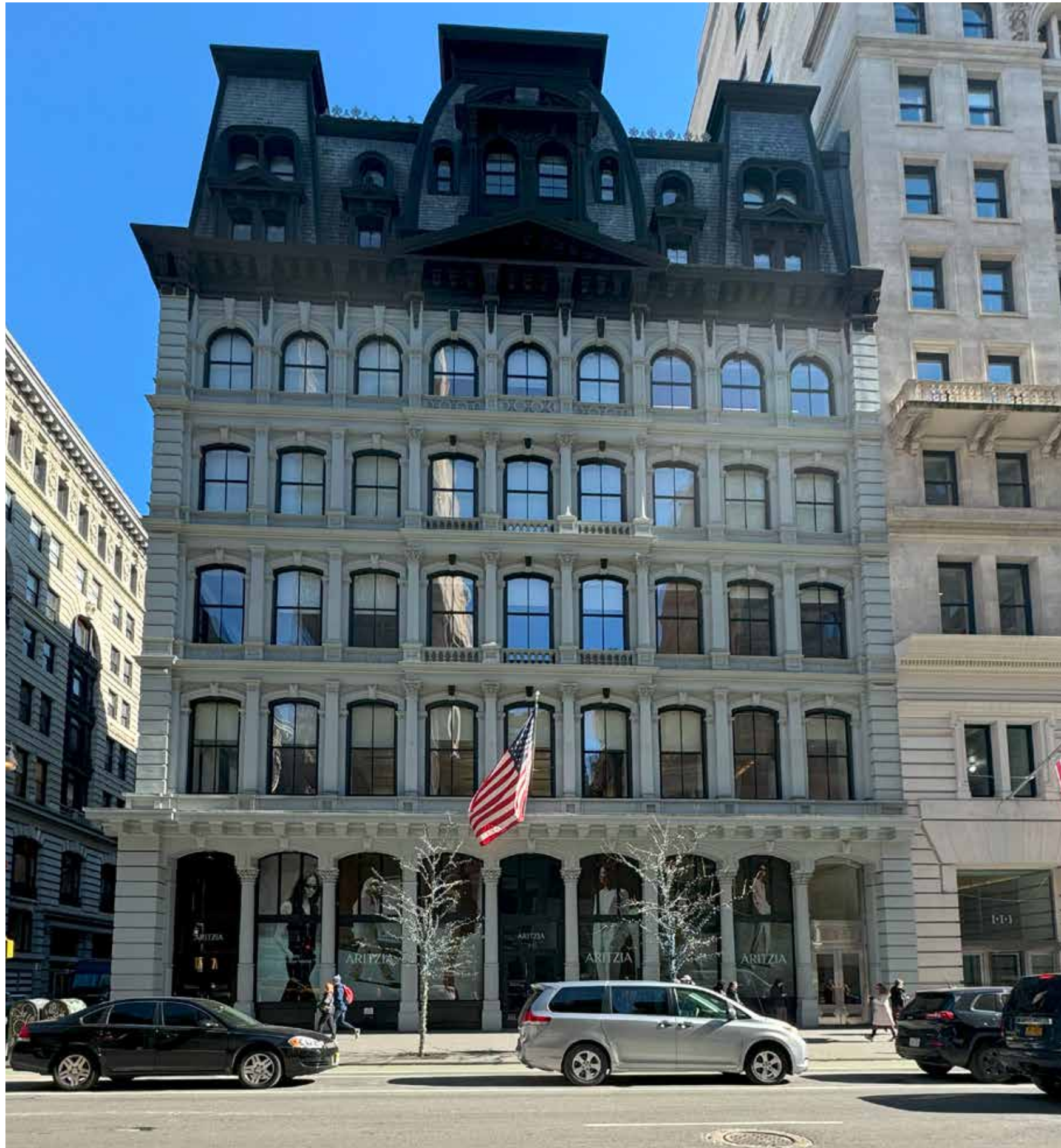
Existing Store Front
