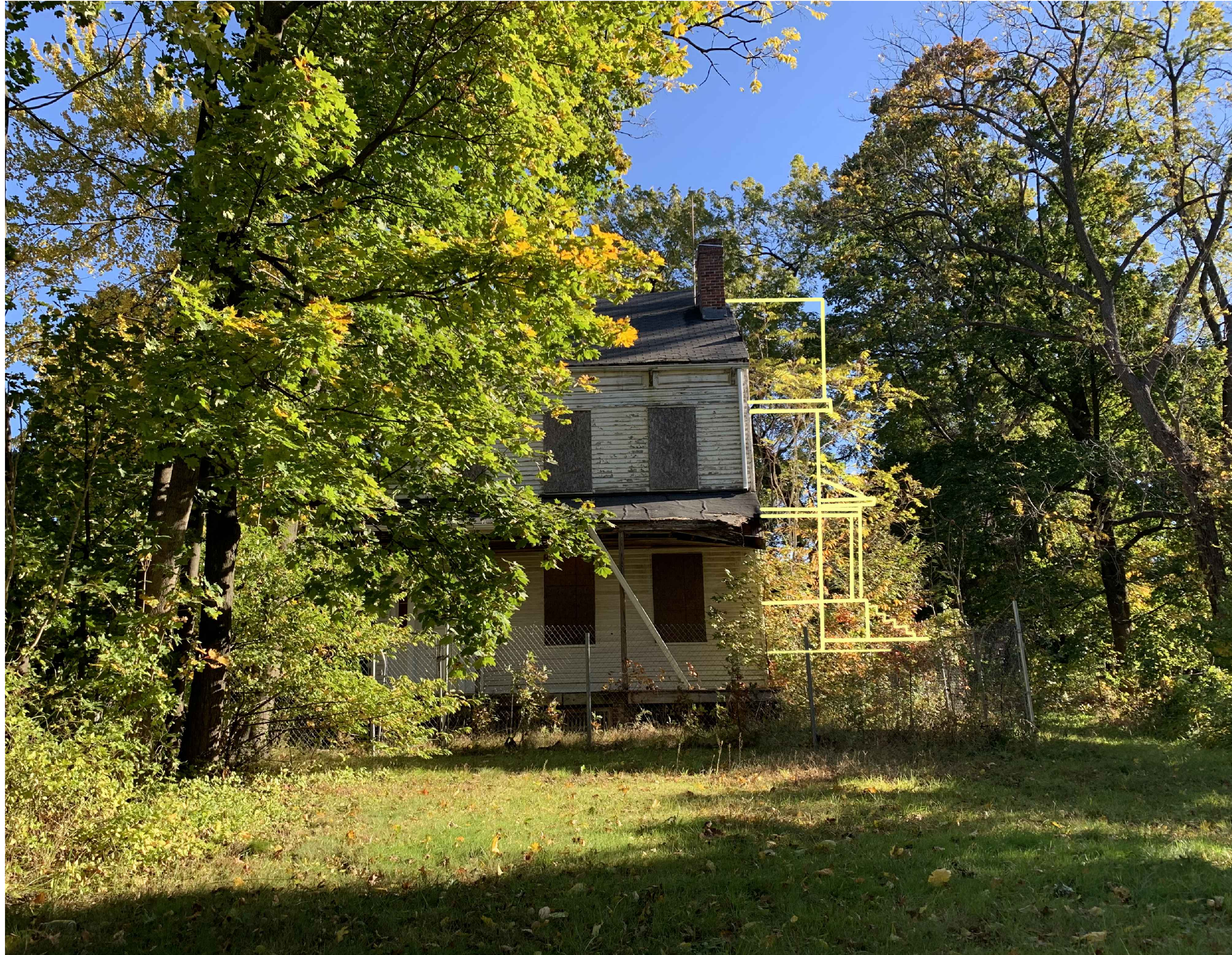
FRONT VIEW JKV HOUSE VIEW FROM CLOVE ROAD
