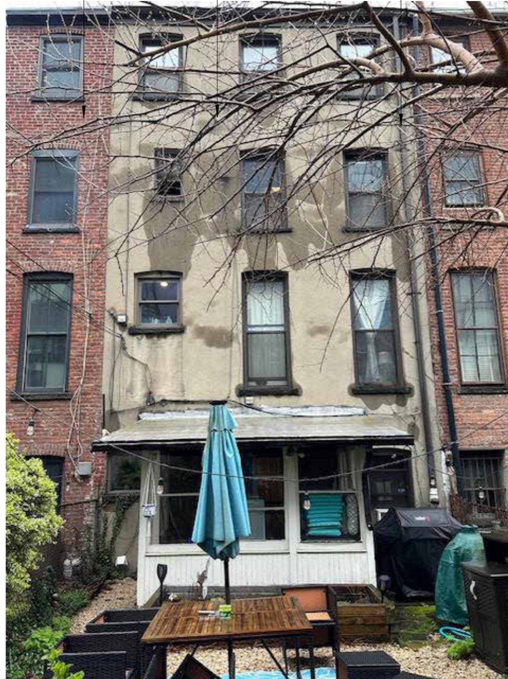
21-33 45TH AVE - REAR FACADE
