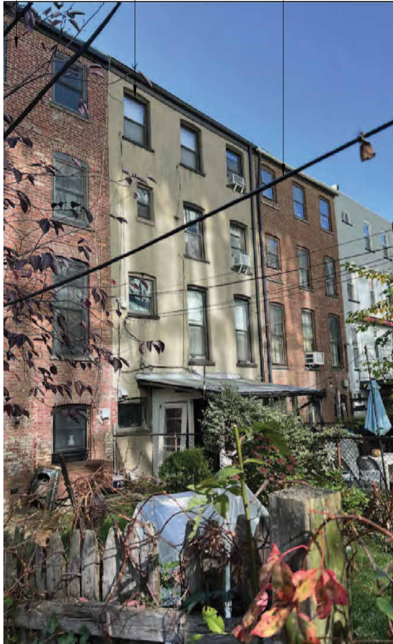
21-33 45TH AVE - REAR FACADE
