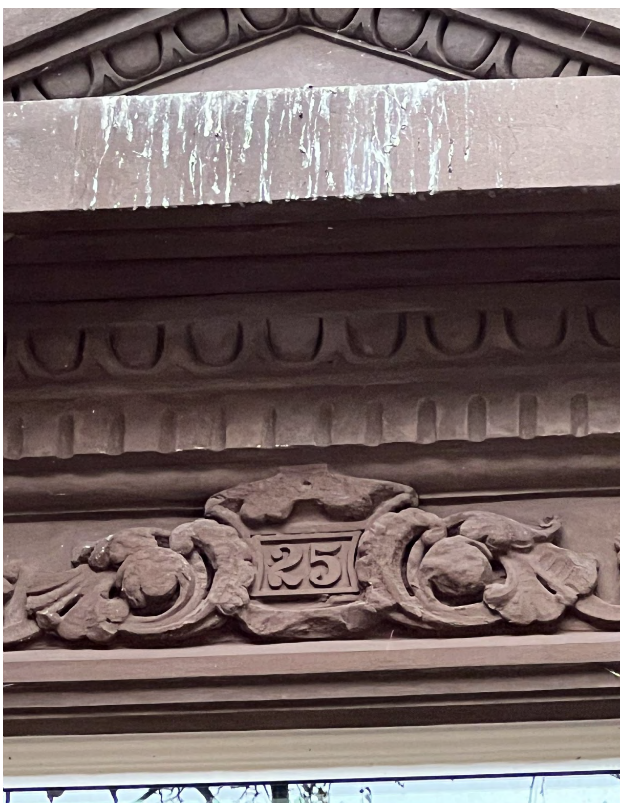
CLOSE-UP DETAILS 23 EAST & 25 EAST 64TH STREET - 2022
