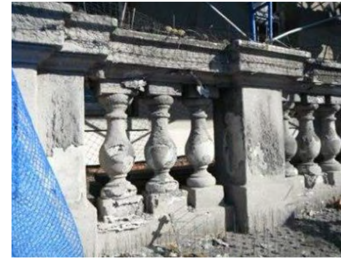
ORIGINAL TERRACE BALUSTER
