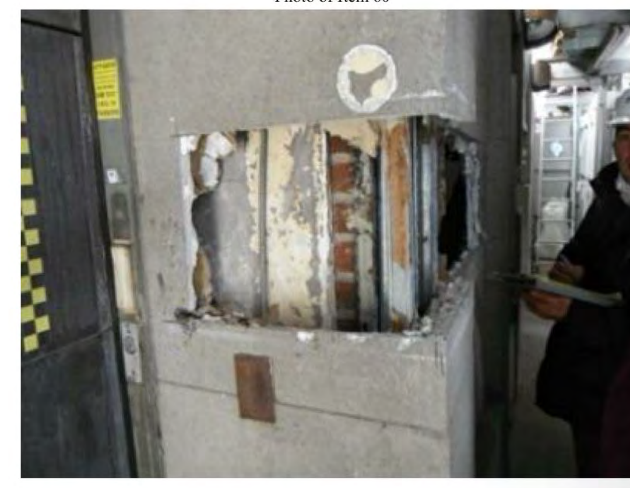
ORIGINAL BRICK HIDDEN BEHIND STUCCO
