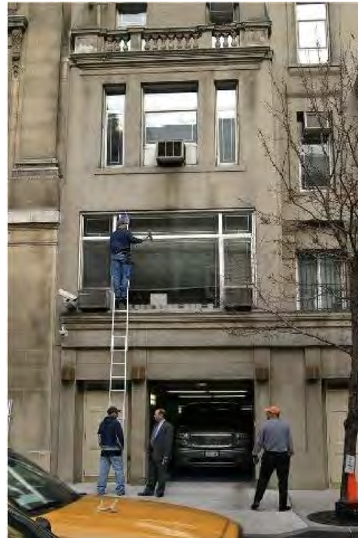
STUCCO FOAM FACADE
