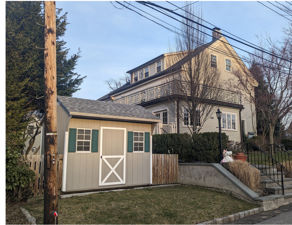
EXISTING NORTH-WEST VIEW - SHED TO BE REMOVED
