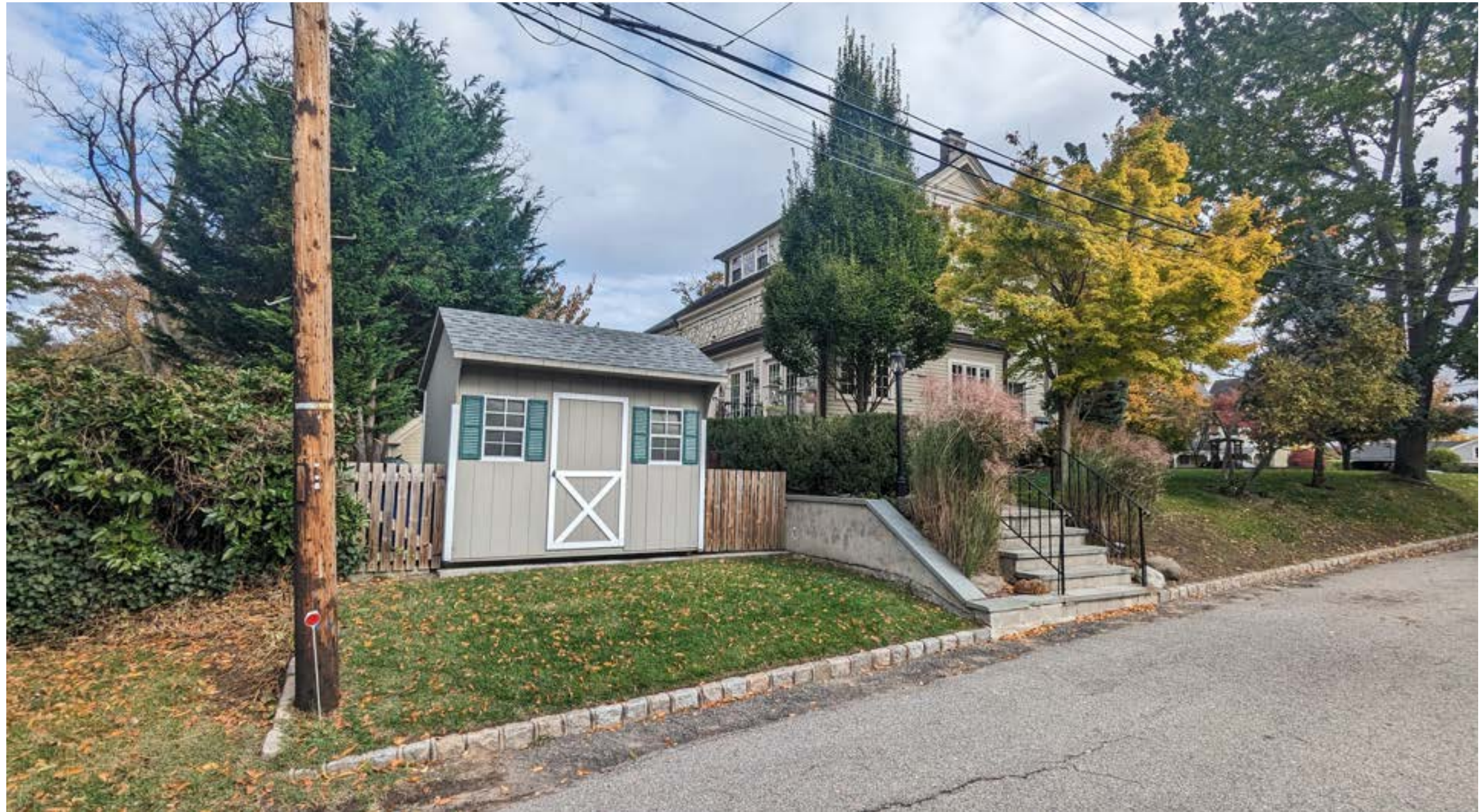
REAR FACADE - NORTH ELEVATION
