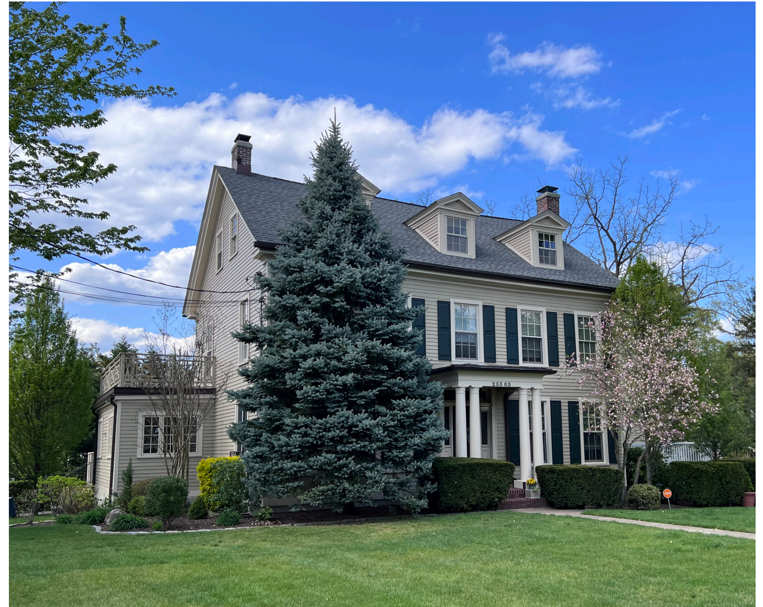
EXISTING SOUTH-WEST VIEW
