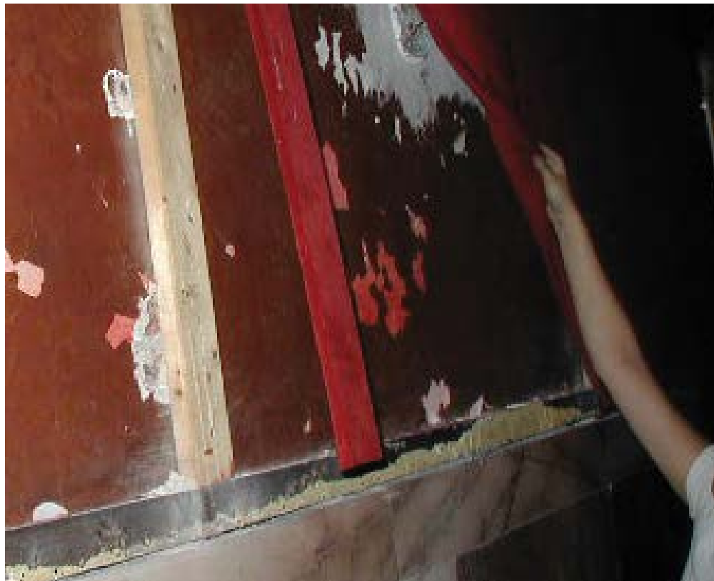
EXISTING FABRIC WRAPPED WALL PANELING DETAILS
