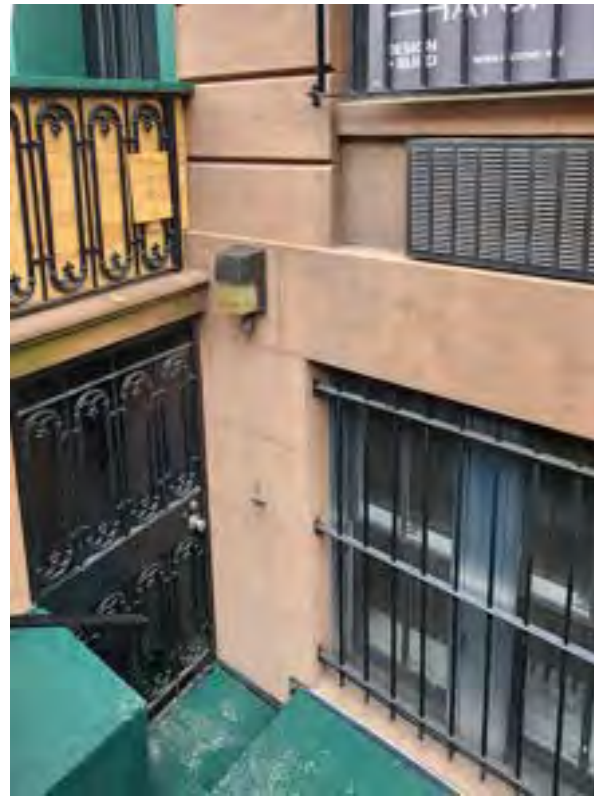
3. #413 CELLAR ACCESS VIEW
