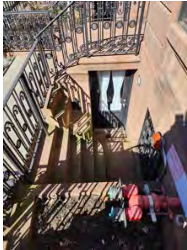
6. #415 CELLAR ACCESS VIEW
