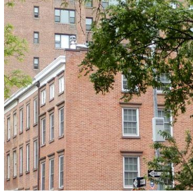
EXISTING (CLOSE UP)
