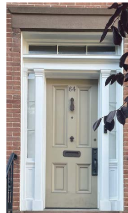
EXISTING FRONT DOOR
