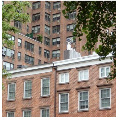
EXISTING (CLOSE UP)
