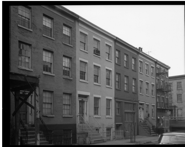
58-66 HORATIO STREET HORATIO STREET SIDE
