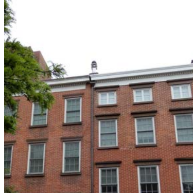
EXISTING (CLOSE UP)
