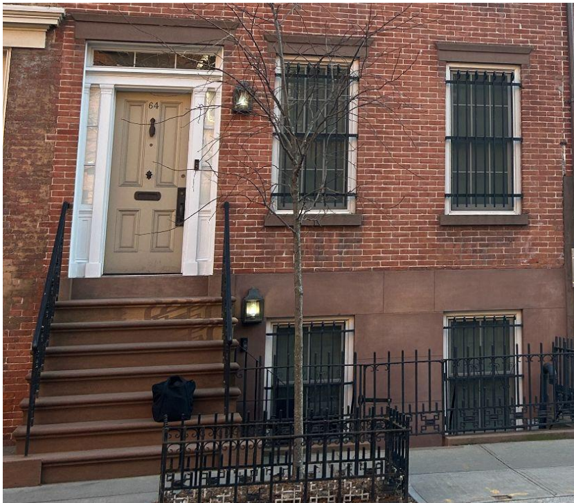
EXISTING FRONT FACADE
