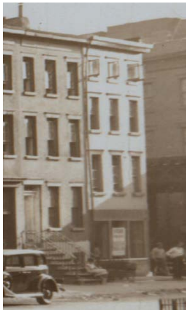
64 & 66 HORATIO STREET HORATIO STREET SIDE
