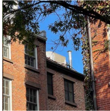
EXISTING (CLOSE UP)
