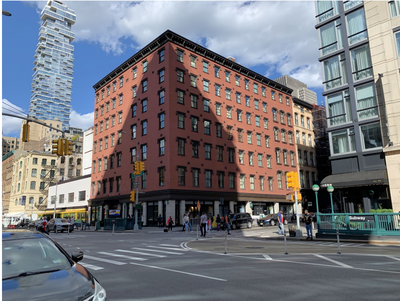
125 CHAMBERS LOOKING NORTHEAST
