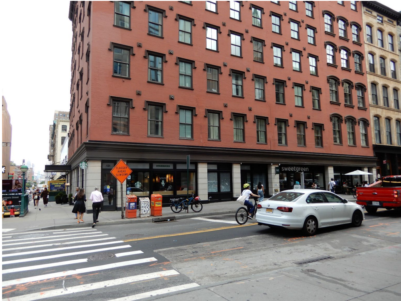
125 CHAMBERS LOOKING NORTHEAST
