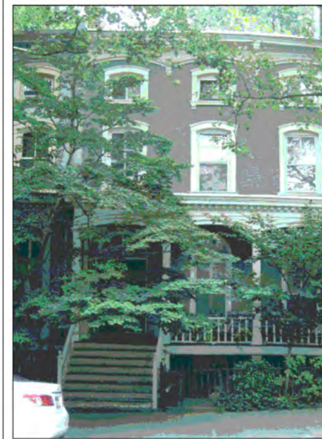
2 VANDERBILT AVENUE WEST FACING ELEVATION [PHOTO] SCALE: 3/32" = 1'-0"
