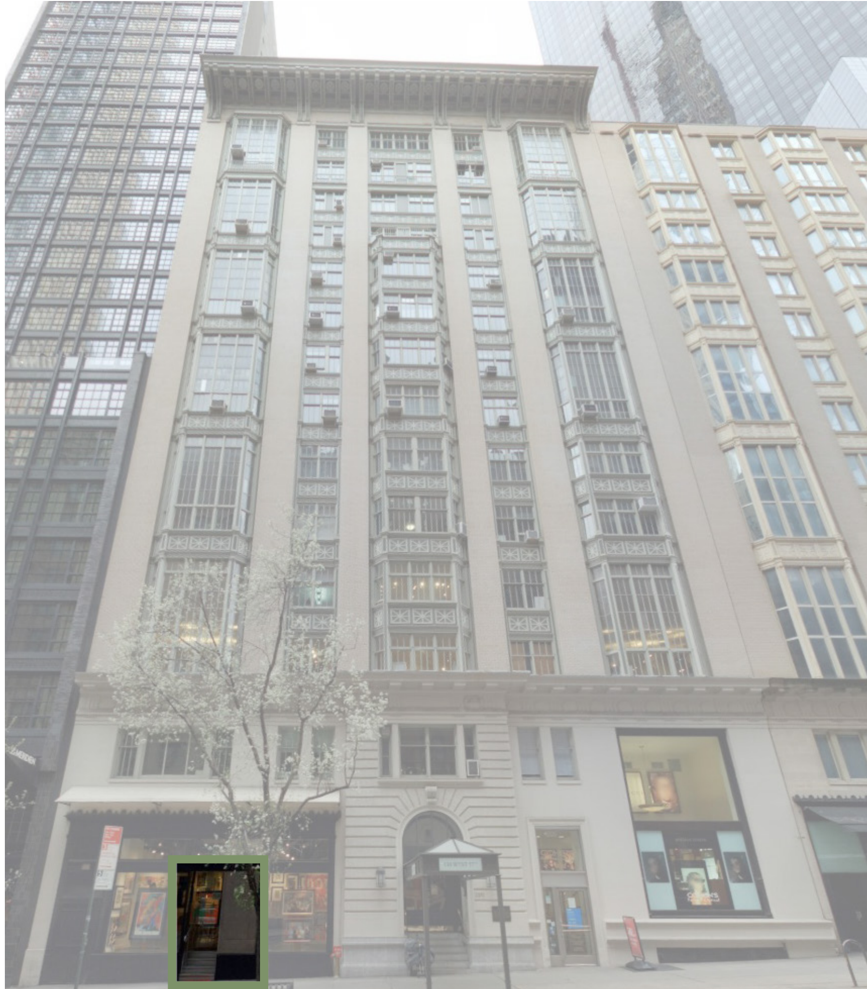
AREA OF WORK
