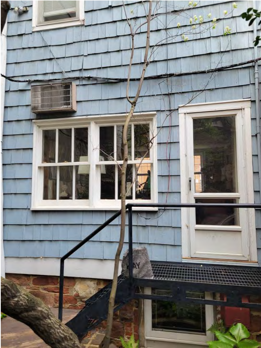
Partial Rear Facade
