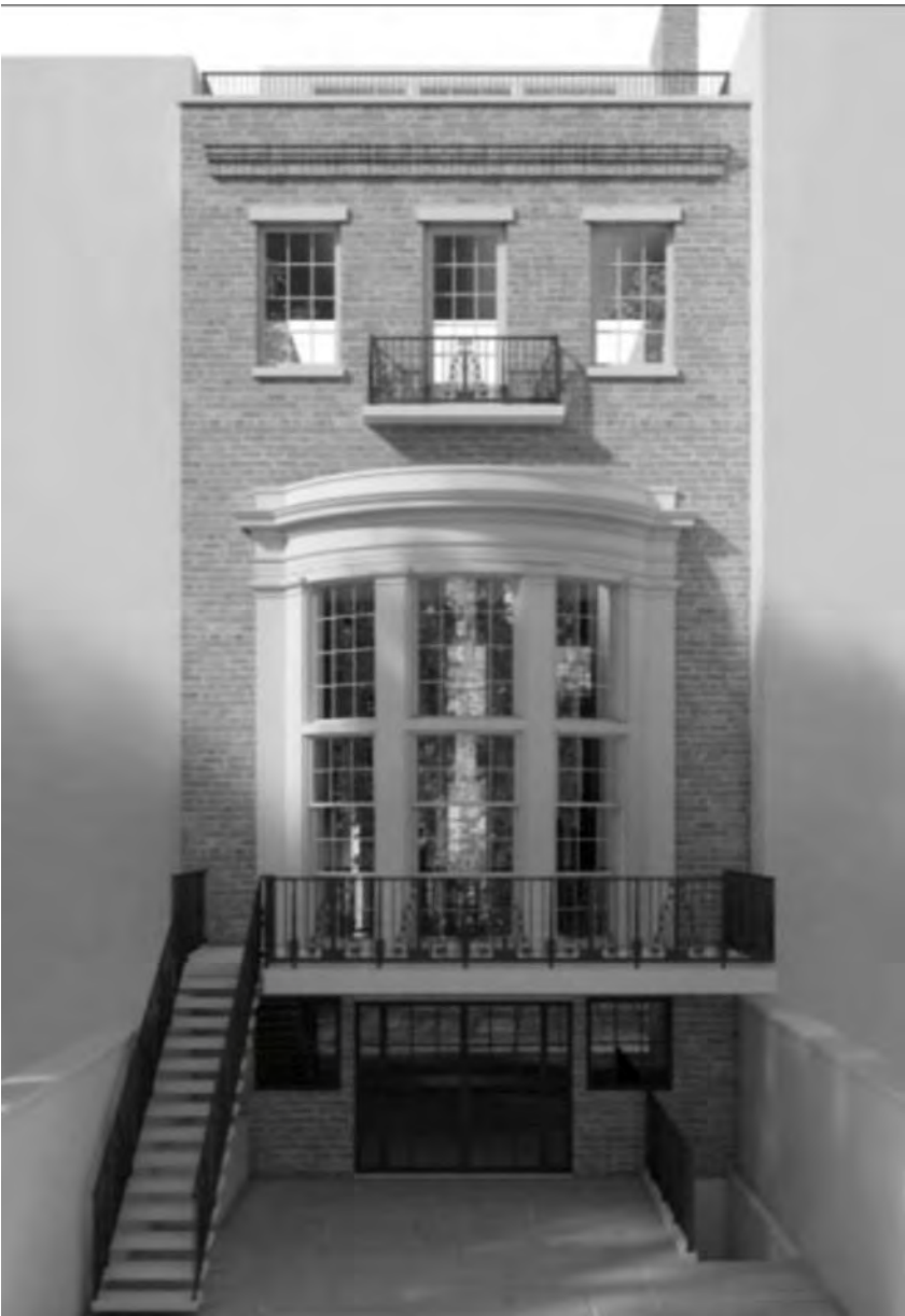
25 EAST 11TH STREET ADDITION WITH BOWED 2-STORY WOOD CLAD PROJECTING BAY, APPROVED IN 2022
