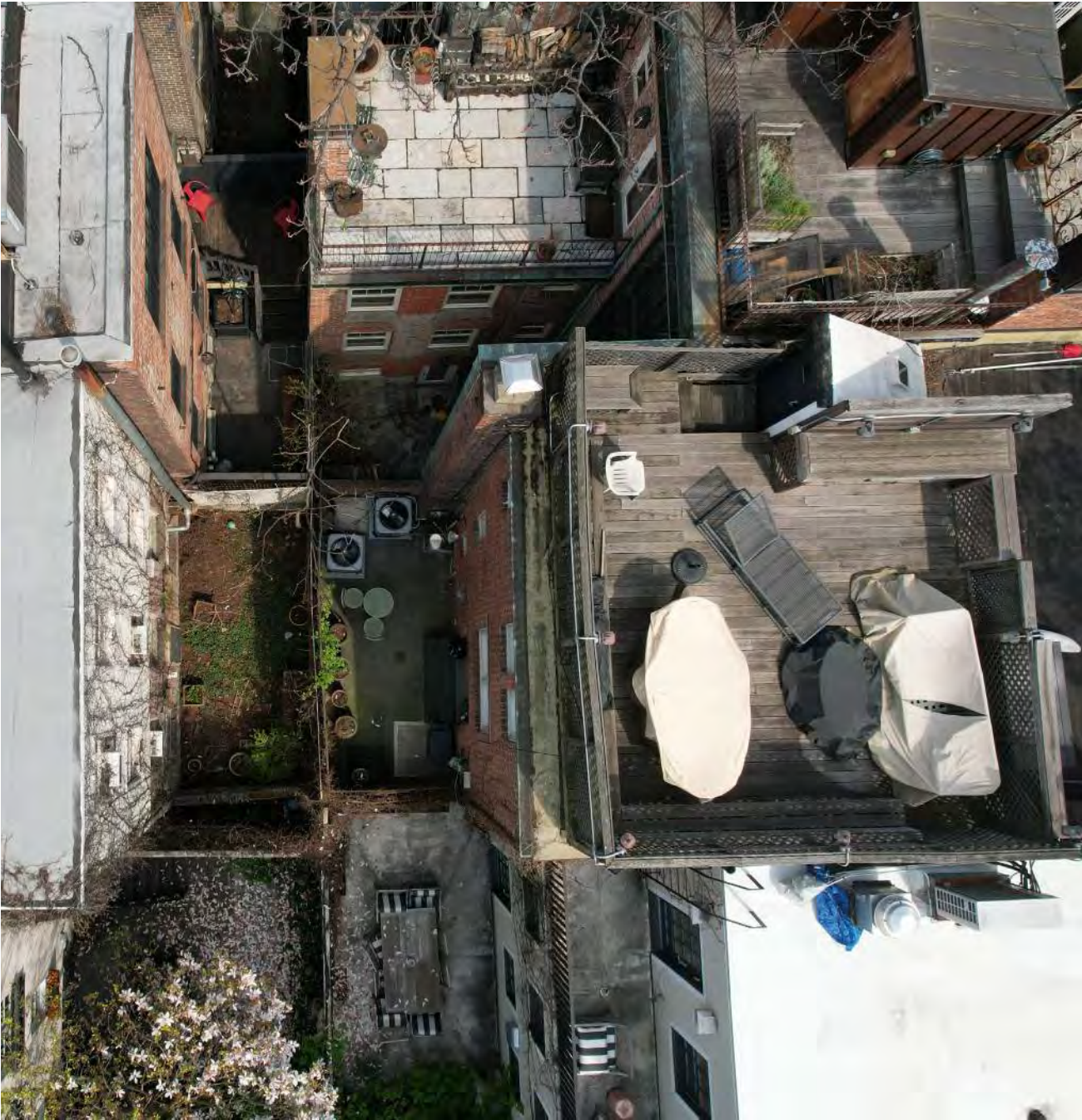
Roof Decks in the Block Center
