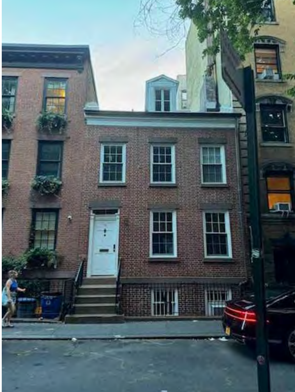
Photo of Primary Facade
