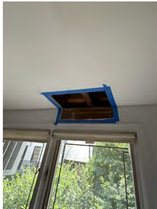
Probe 22 at roof and attic rear wall showing newer framing at existing roof
