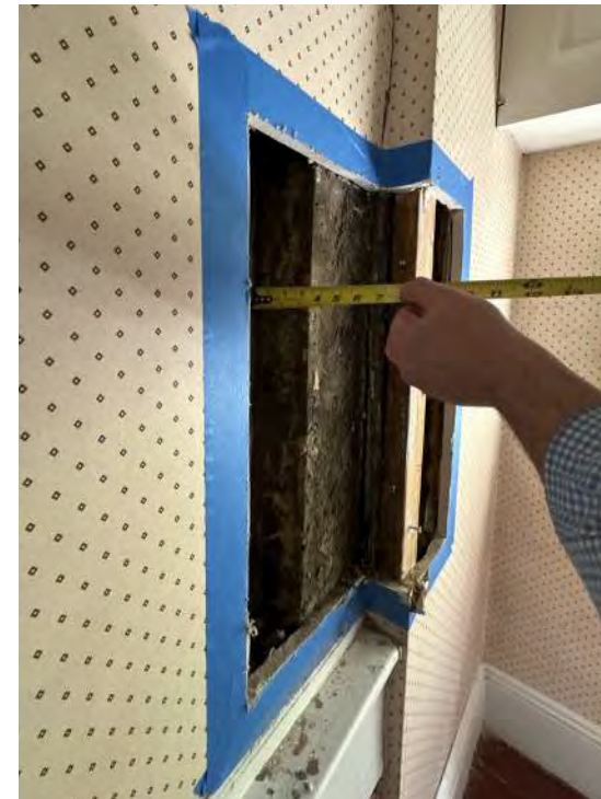
Probe 16 at party wall showing original wood frame and newer wood frame towards the rear wall
