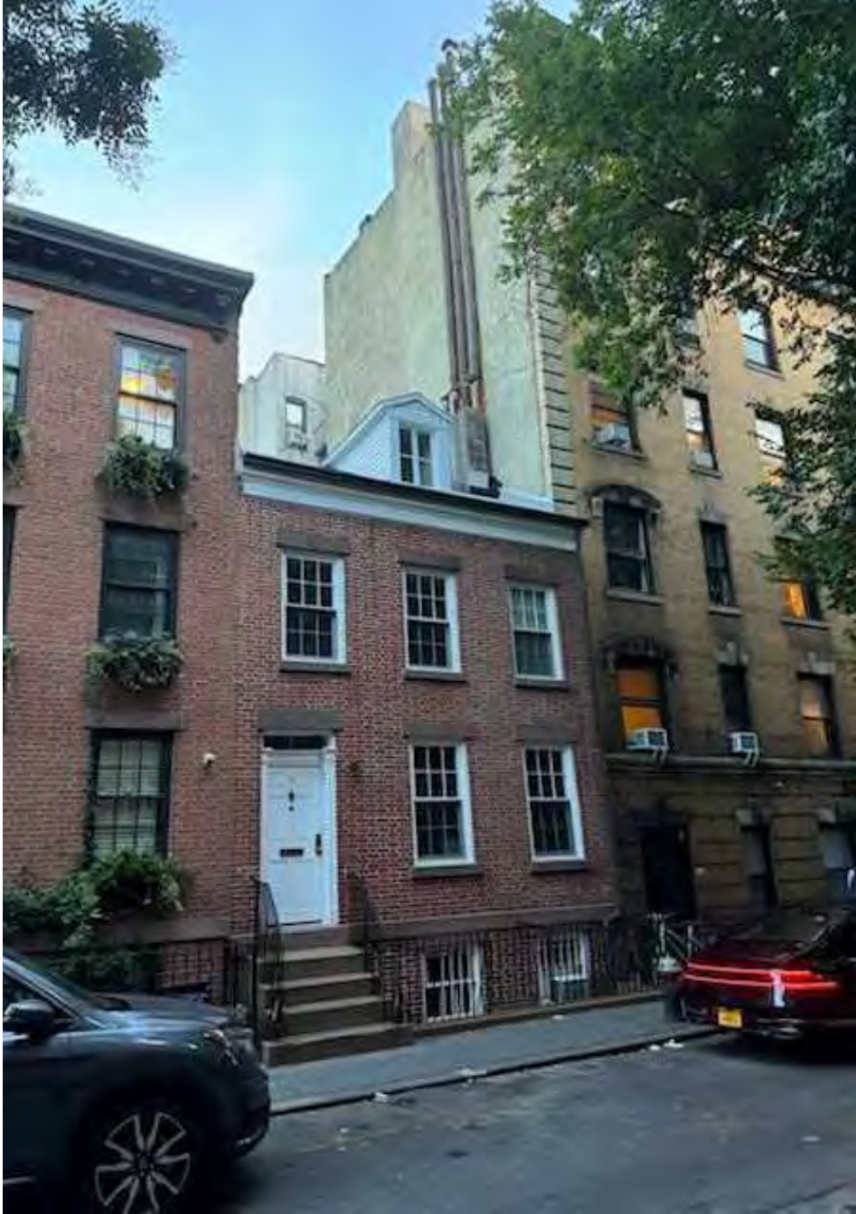
Photo of Primary Facade looking West
