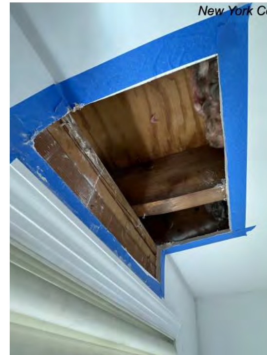
Probe 22 at roof and attic rear wall showing newer framing at existing roof
