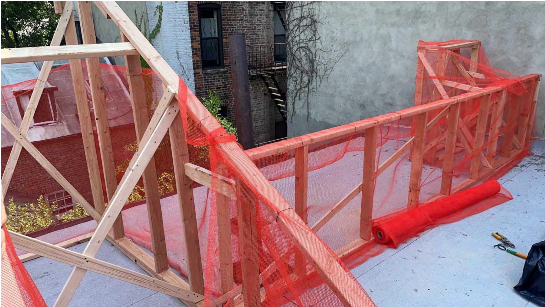
Photo of Railing and HVAC Unit looking West
