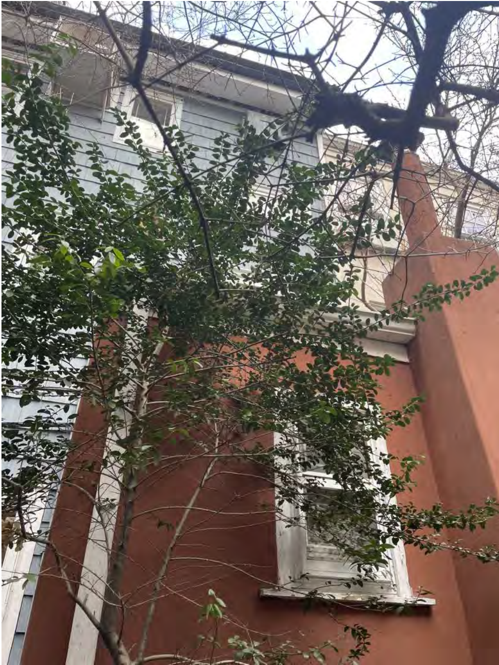
Partial View of the Existing Rear Addition
