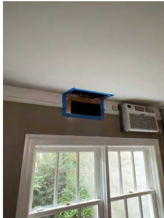
Probe 5 at first floor rear wall and ceiling
