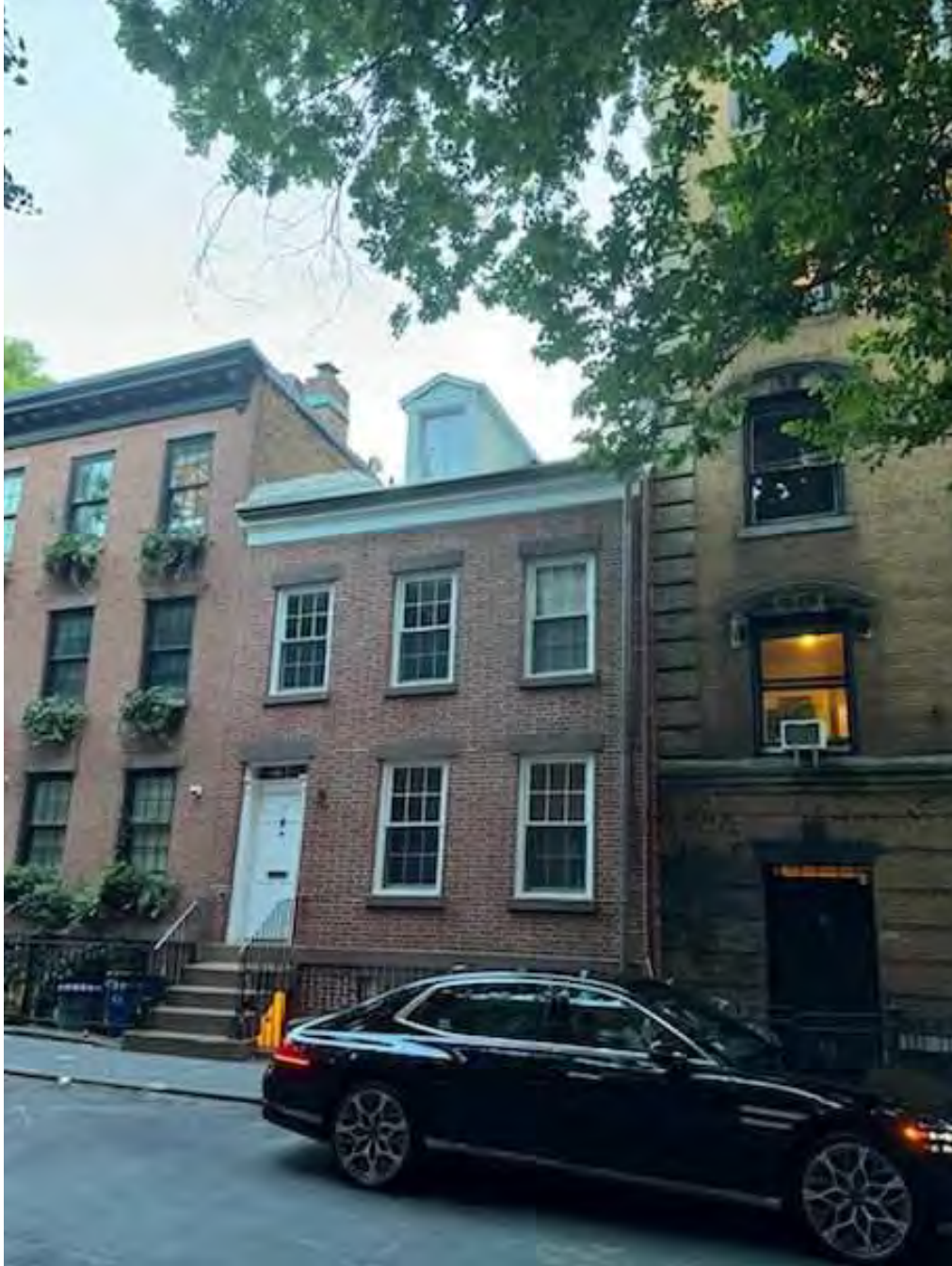
Photo of Primary Facade looking East
