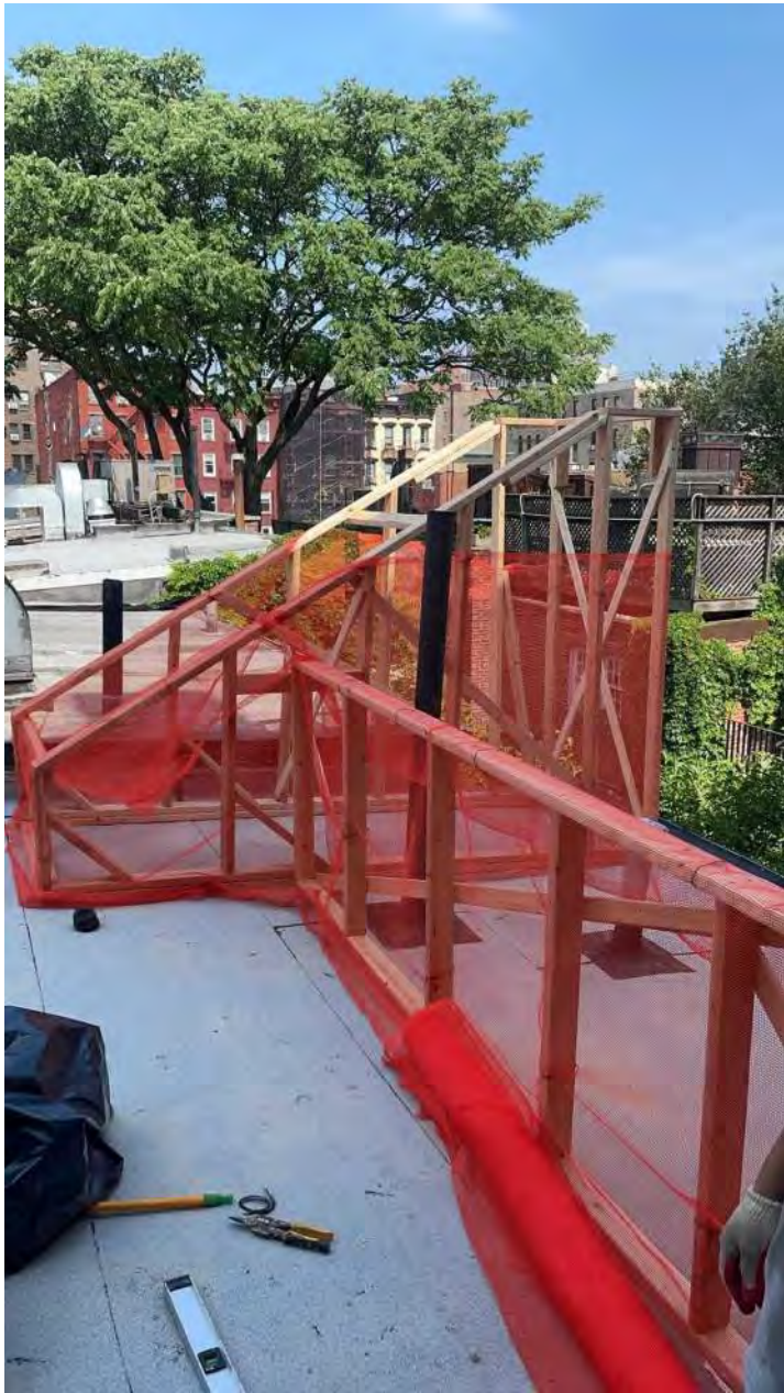
Photo of Bulkhead looking East
