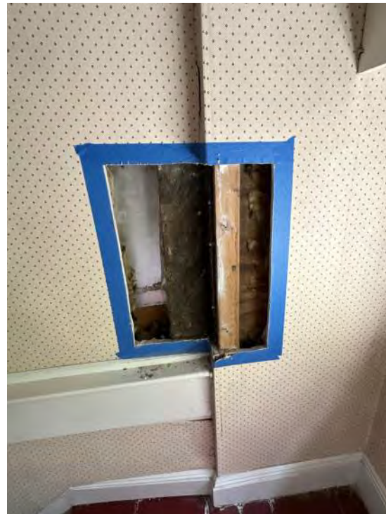
Probe 16 at party wall showing original wood frame and newer wood frame towards the rear wall
