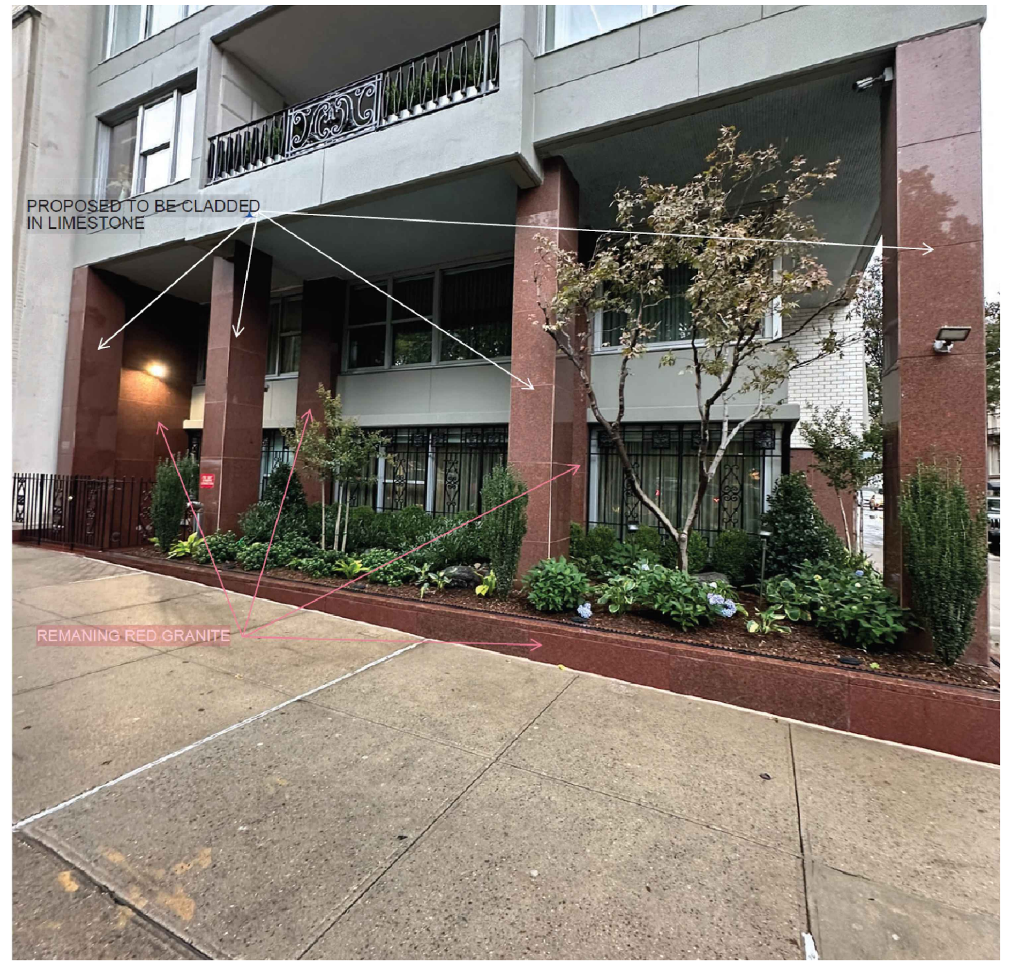
3 WEST ELEVATION - EX. PHOTOGRAPH Scale: NTS
