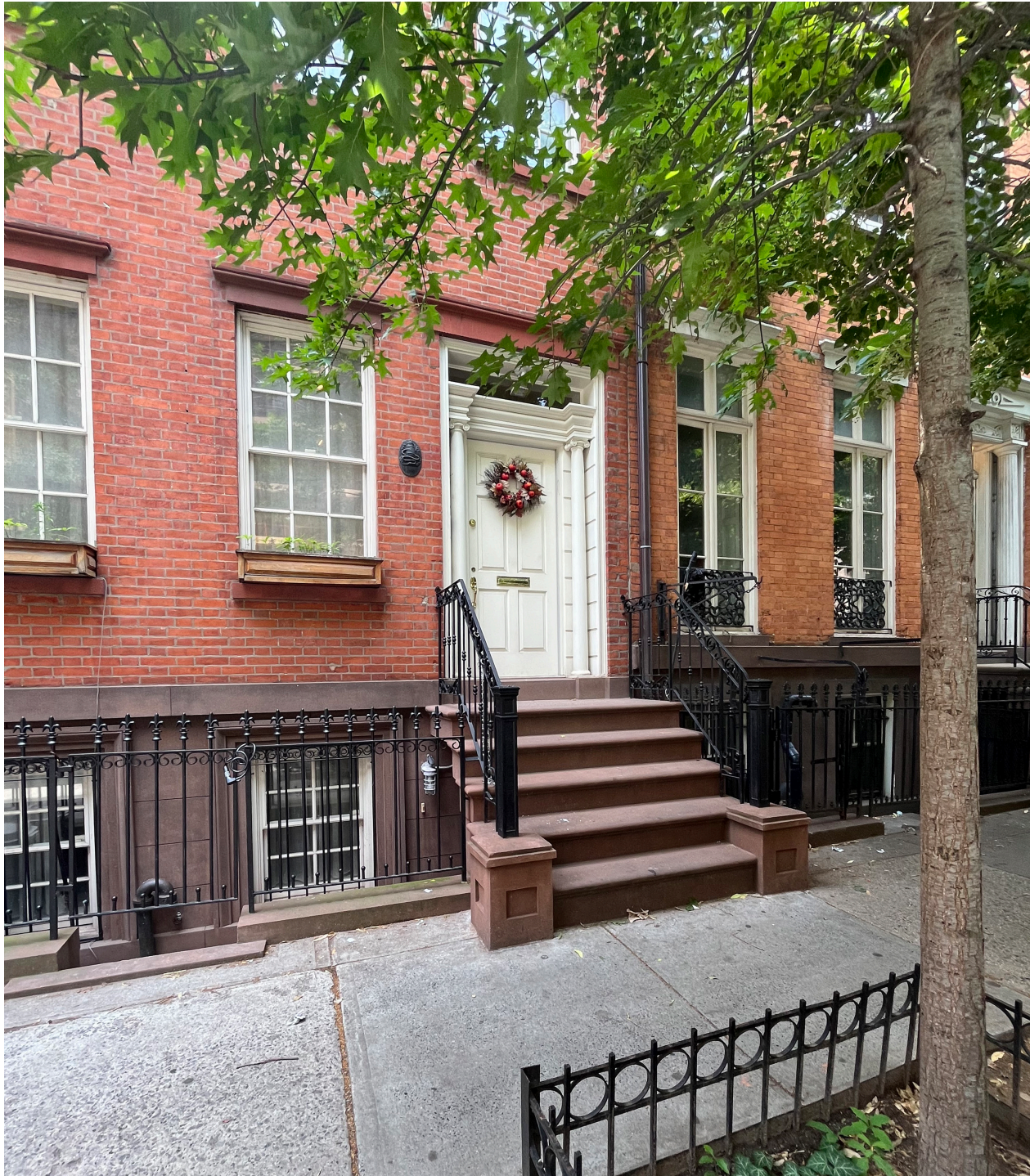
EXISTING CONDITIONS: CLOSE UP
