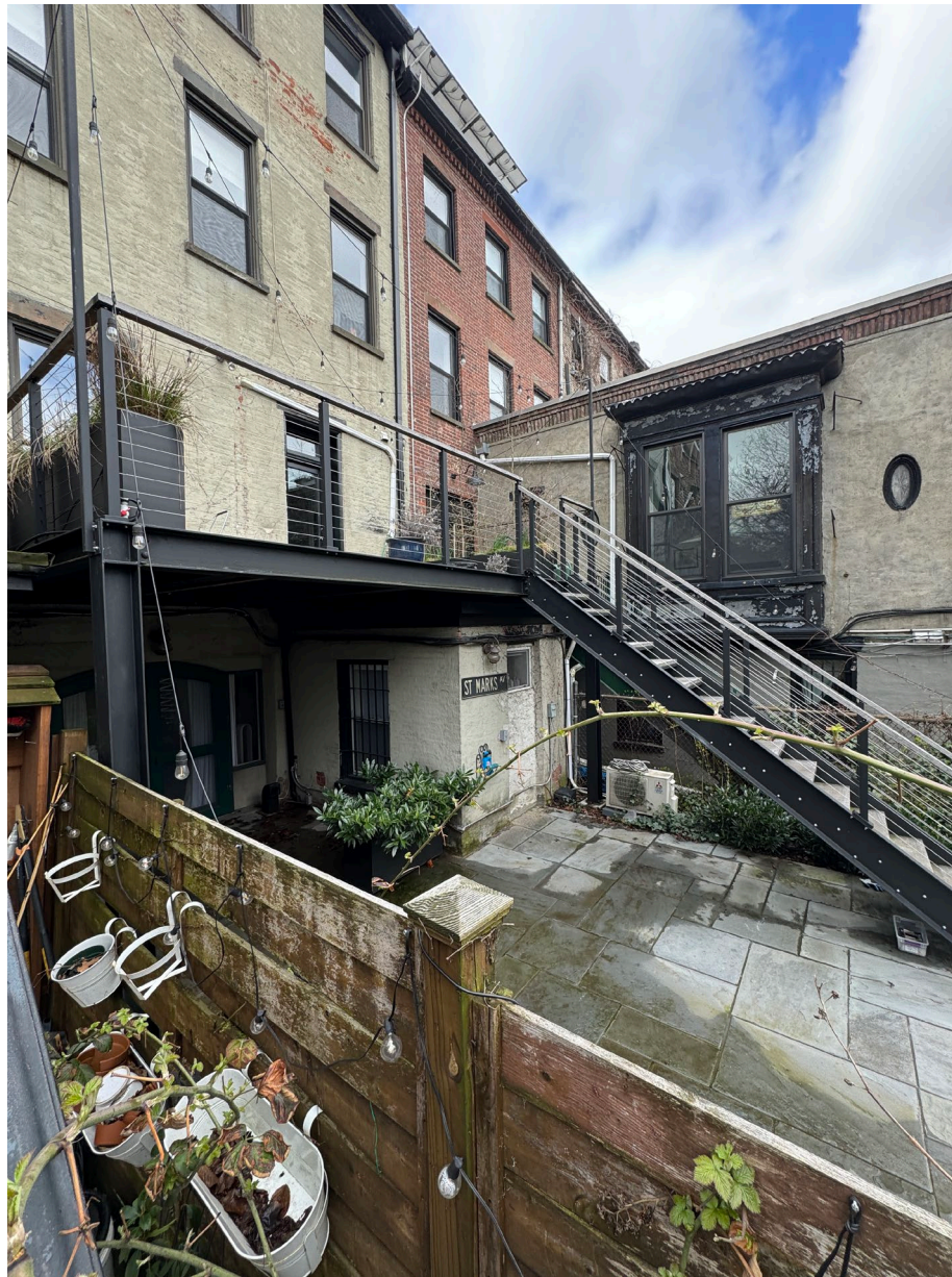
VIEW OF EXISTING REAR ADDITION AND DECK OF 121 ST MARKS AVE
