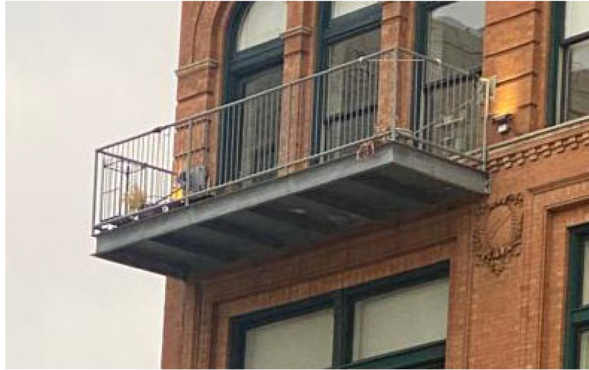
EXAMPLE OF SECOND FLOOR BALCONY
