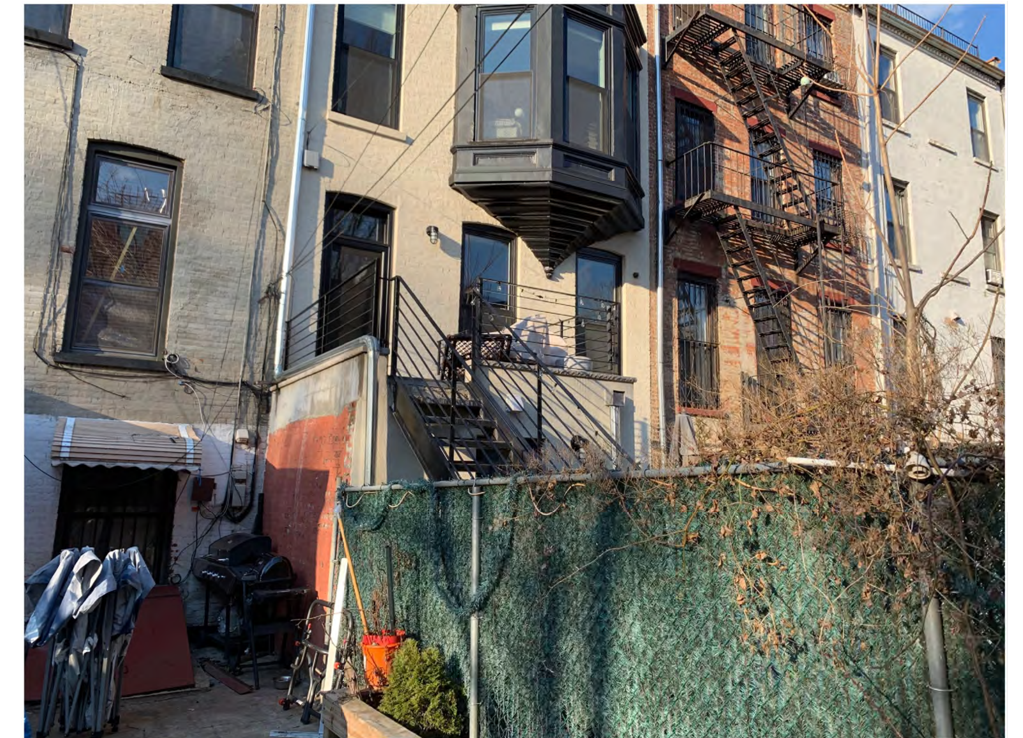
EXISTING FIRE ESCAPE AT 196 MACDONOUGH ST
