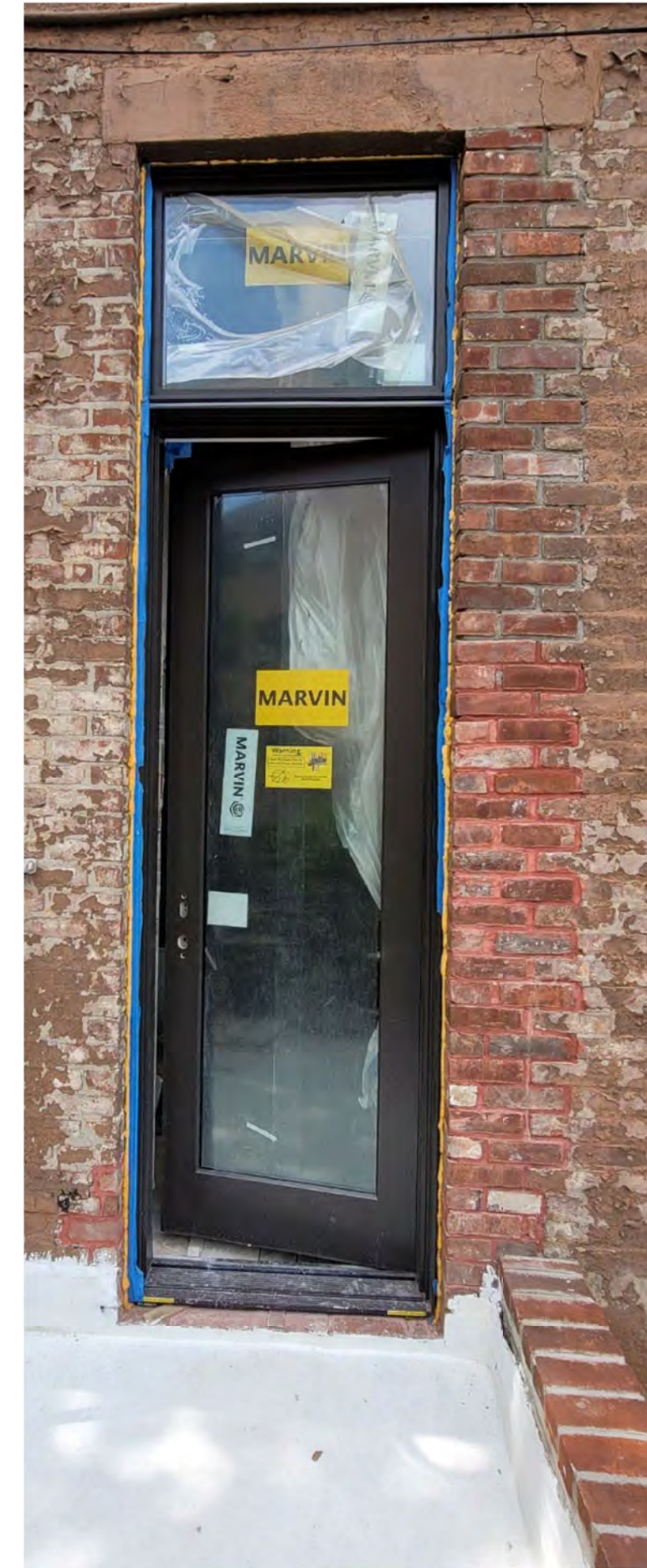
EXAMPLE OF SECOND FLOOR BALCONY
