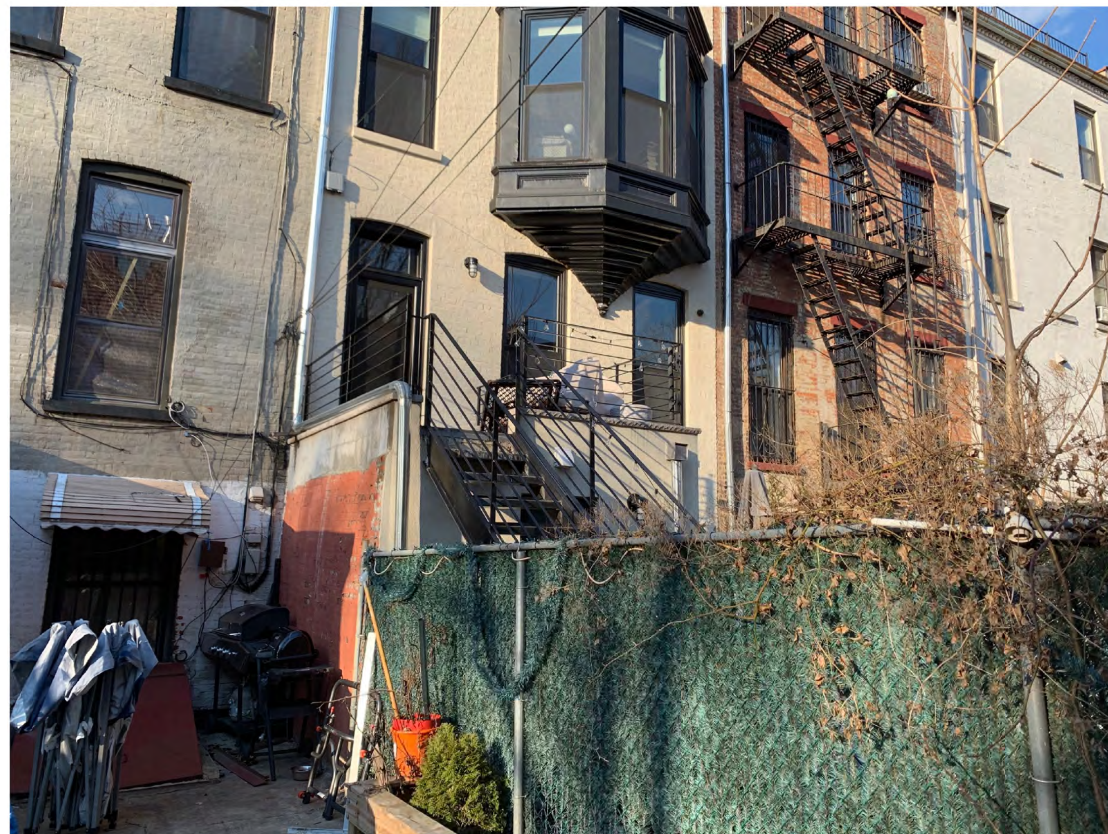
Rear Yard condition of right adjacent property
