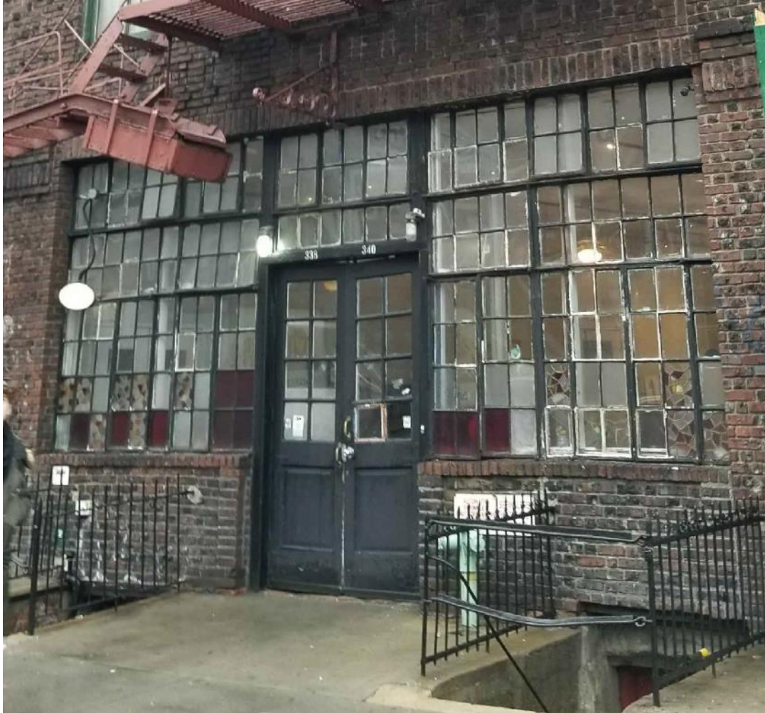
Existing original doors @ North storefront
