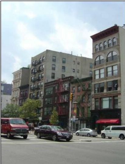
VIEW FORM NORTHEAST CORNER OF BOWERY AND EAST 3RD ST. ③ SCALE N.T.S.
