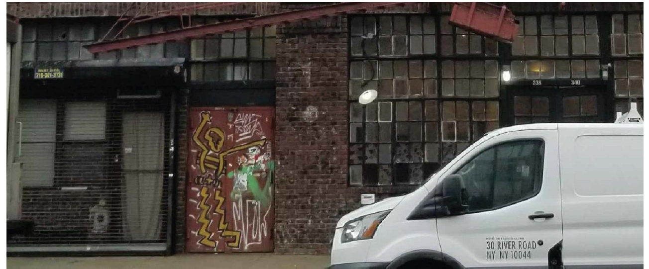
Existing non-original doors @ South storefront
