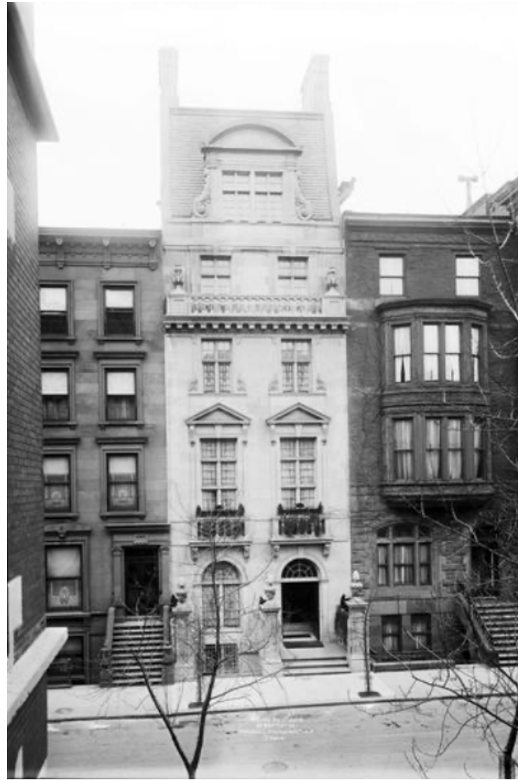
32 E 70 th Street (1914) UES Historic District, designated 1981
