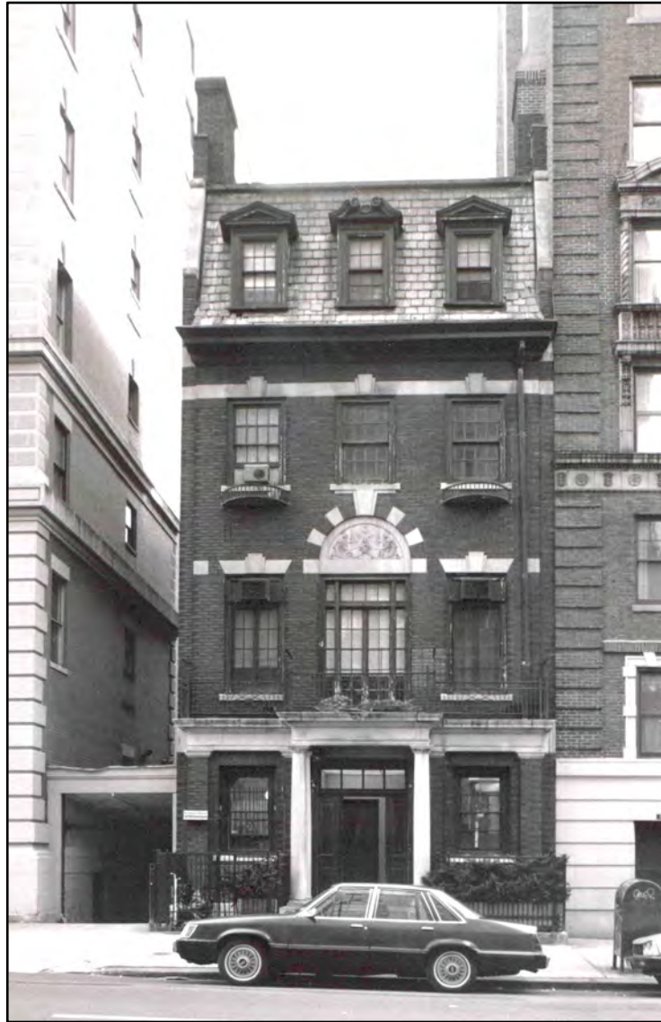
LPC Designation photo, 1990
