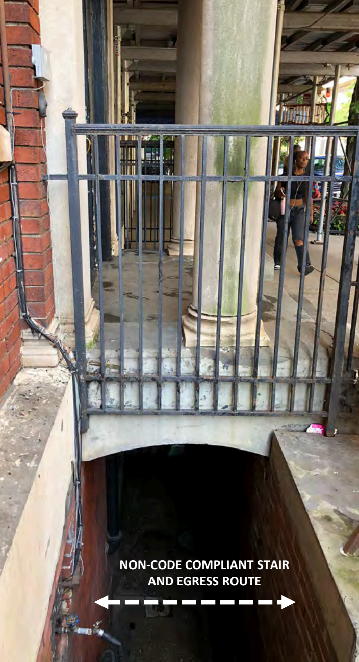
EXISTING AREAWAY STAIR
