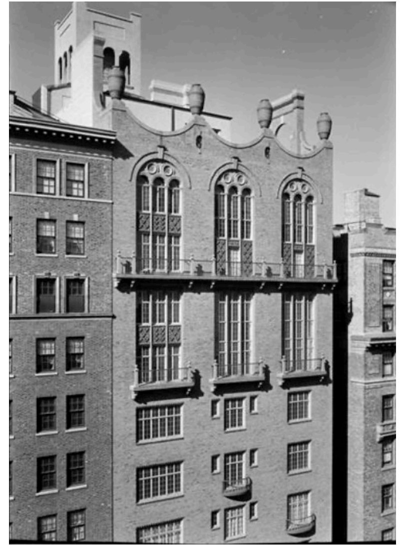
160 E 72 nd Street (1928) UES Historic District, designated 2010
