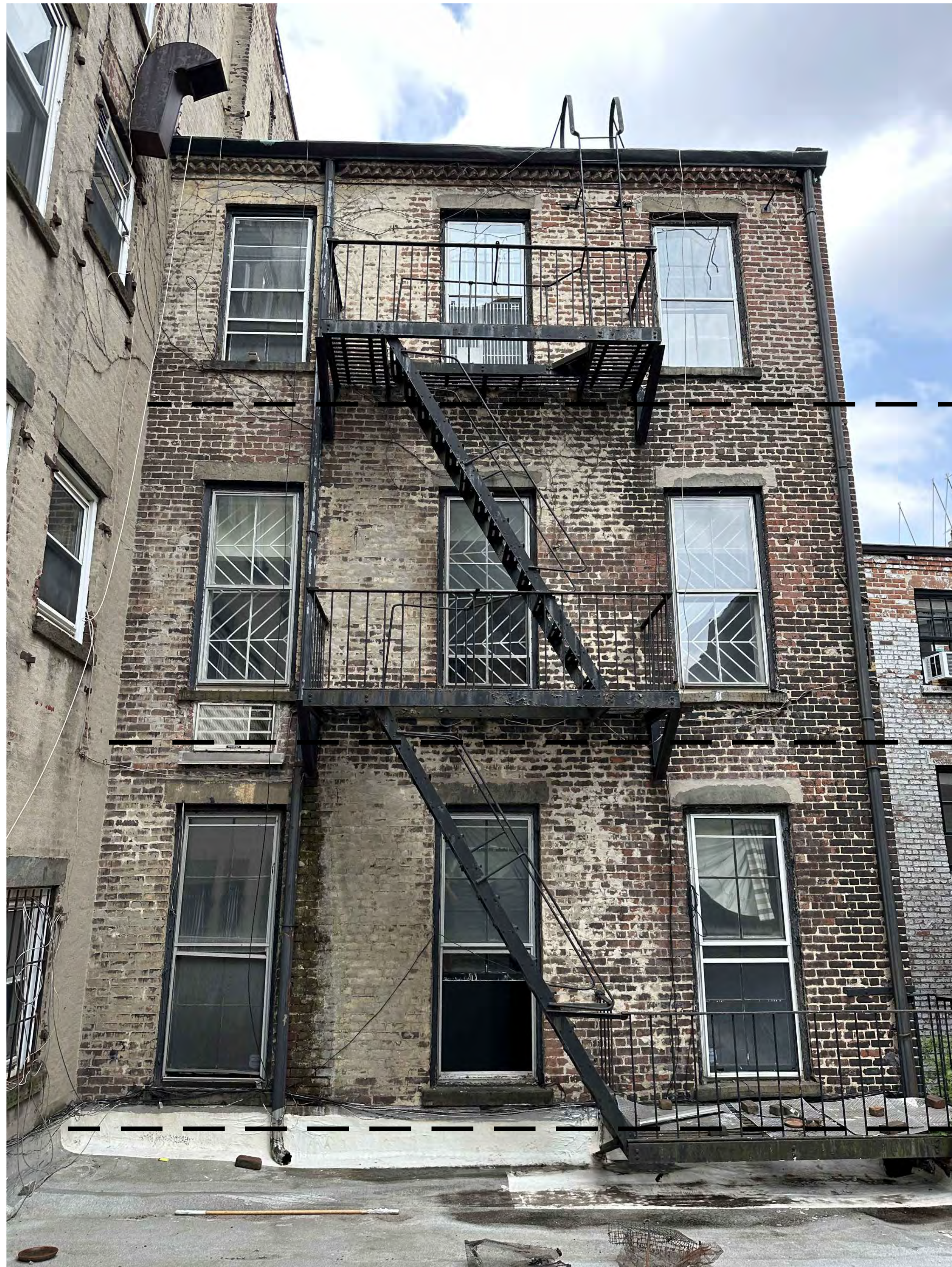
EXISTING REAR FACADE ELEVATION PHOTO
