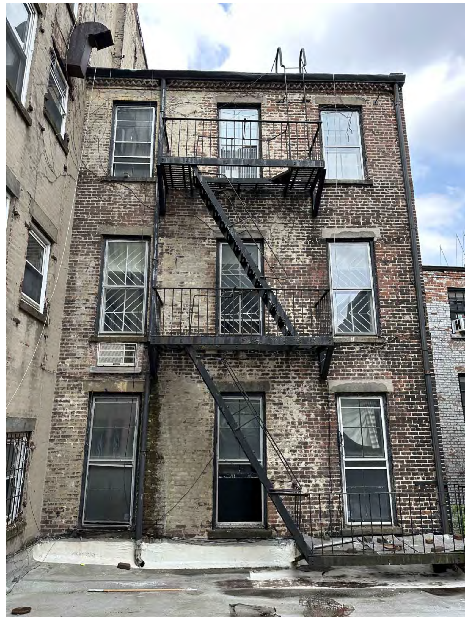
EXISTING REAR FACADE ELEVATION PHOTO
