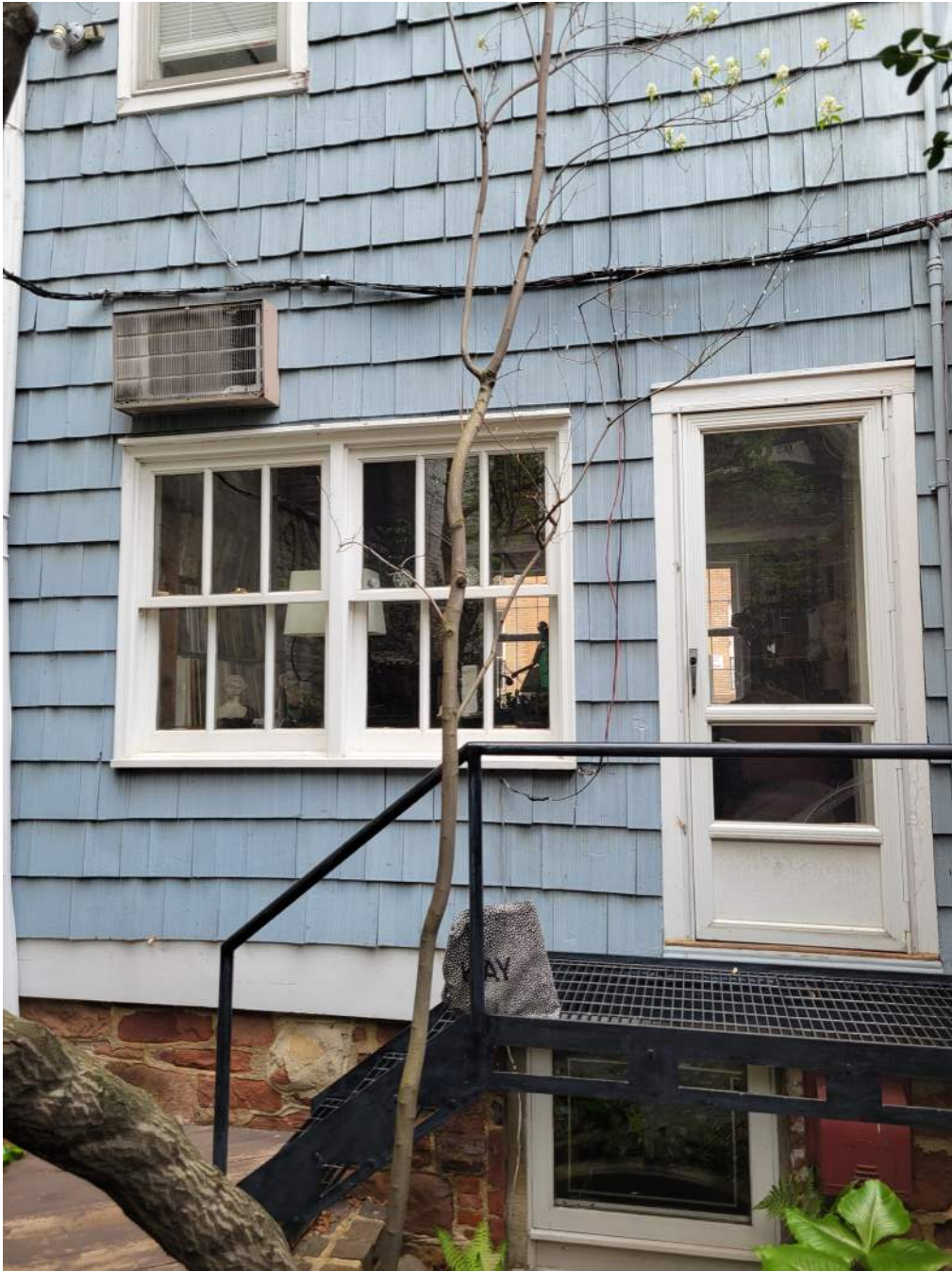
Partial Rear Facade
