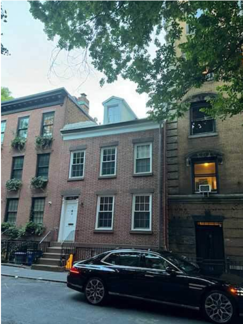
Photo of Primary Facade looking East
