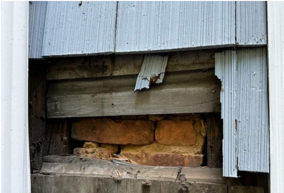
Left: Photo of fire brick infill Right: Photo of rear facade
