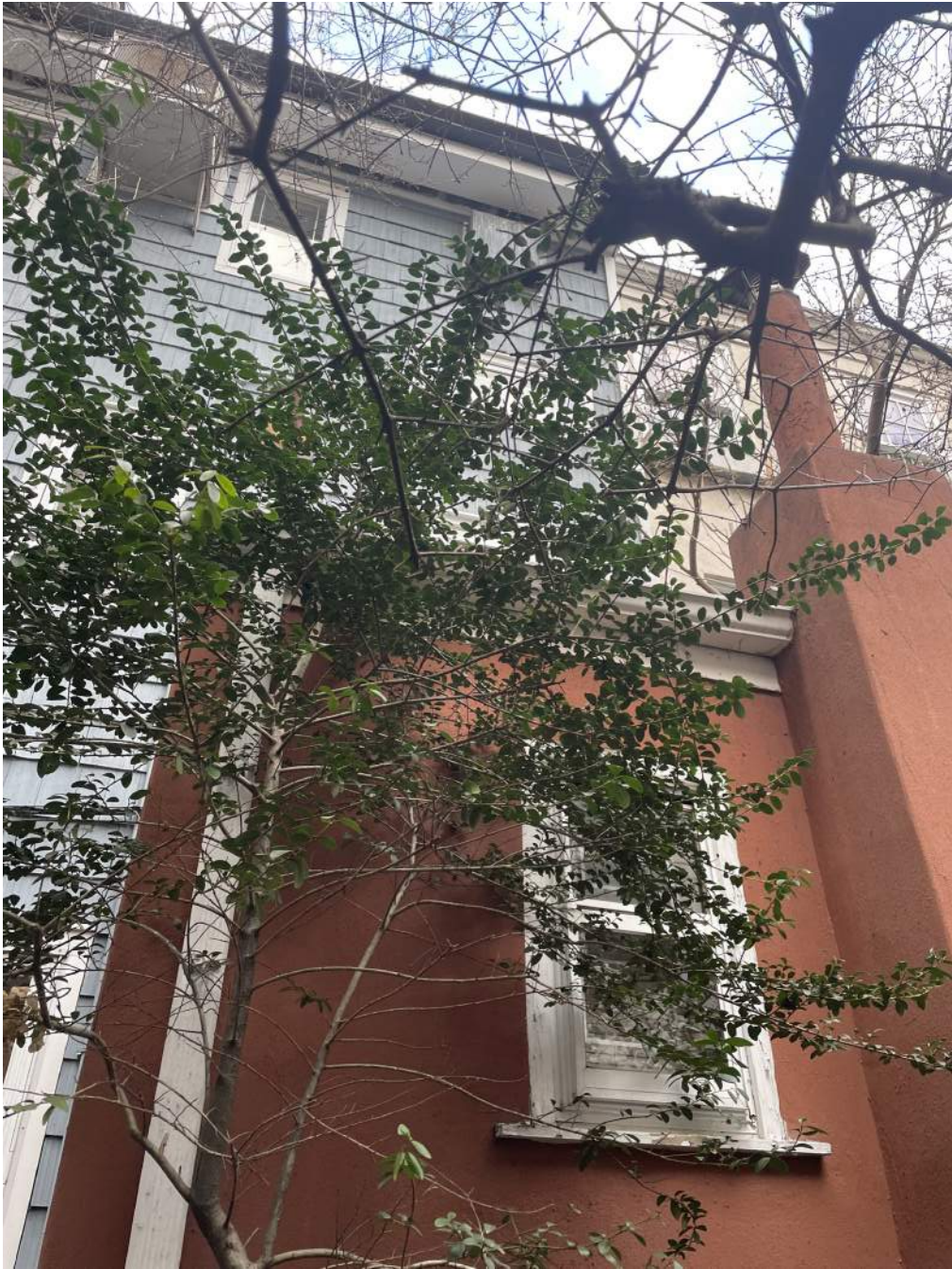
Partial View of the Existing Rear Addition
