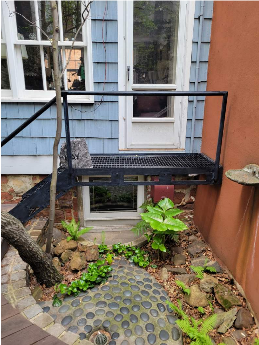
Existing Cellar Window
