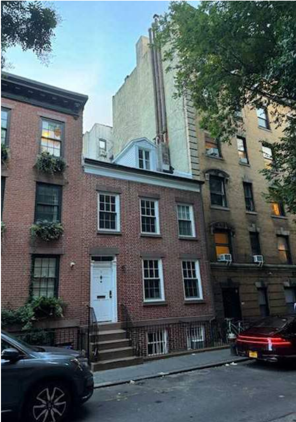
Photo of Primary Facade looking West
