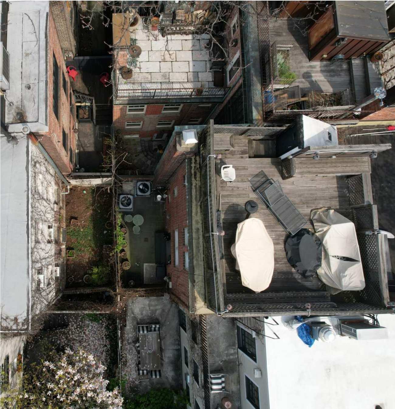
Roof Decks in the Block Center
