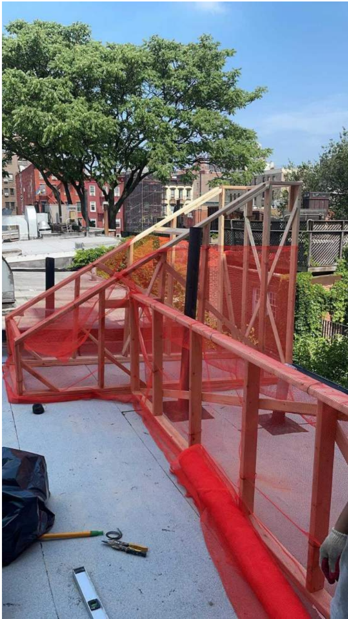
Photo of Bulkhead looking East
