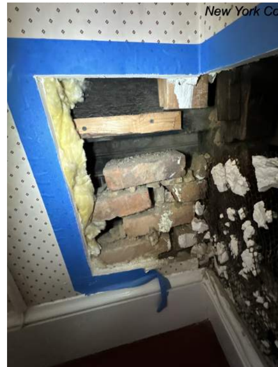
Probe 11 at rear facade showing loose fire brick infill
