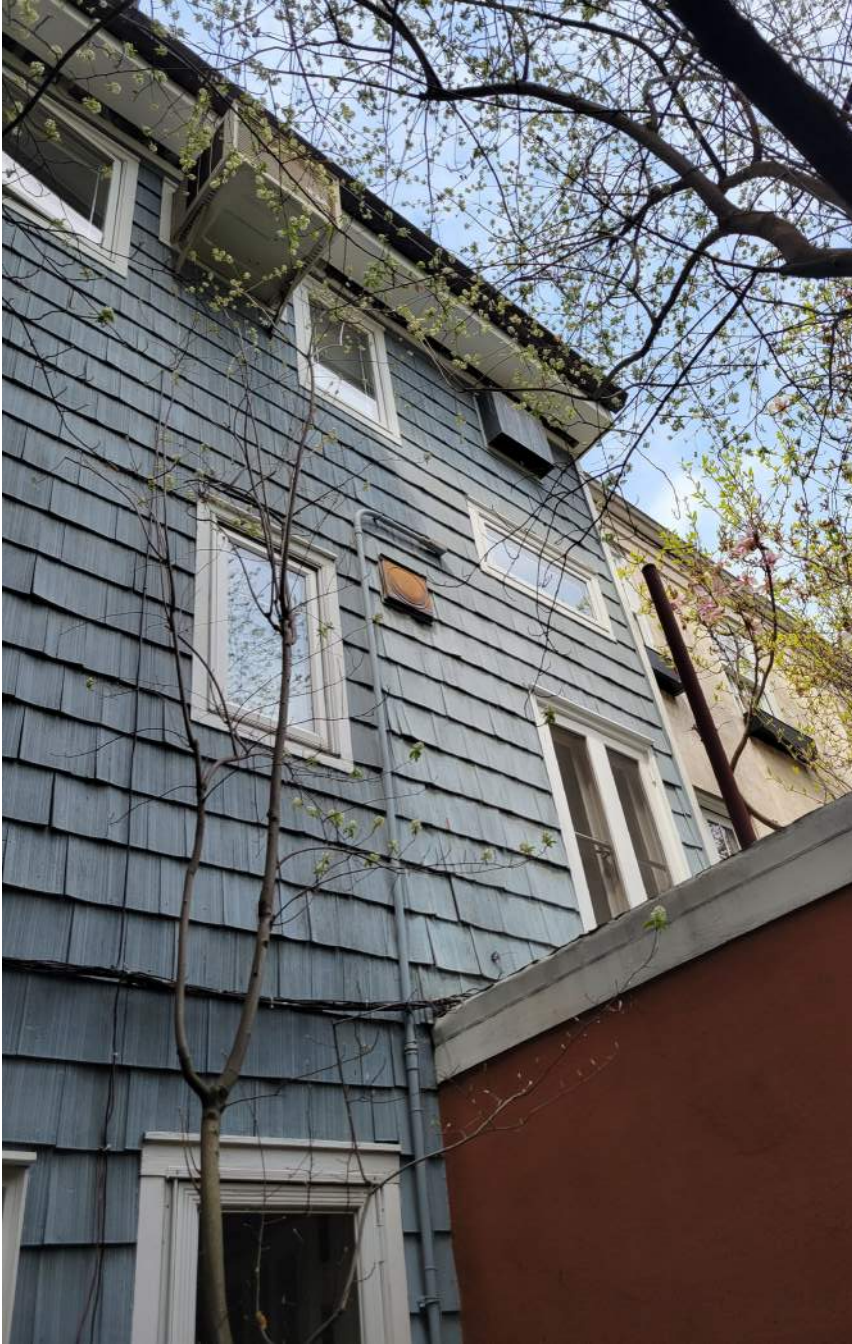
Rear Facade looking East
