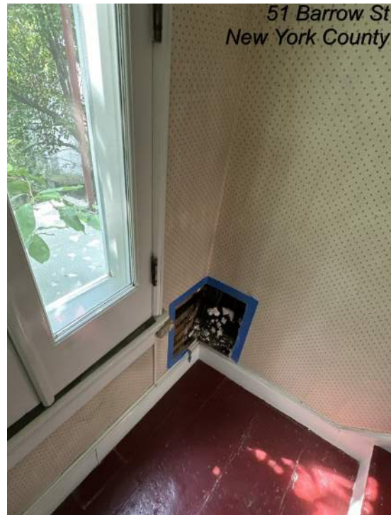
Probe 11 at rear facade showing loose fire brick infill
