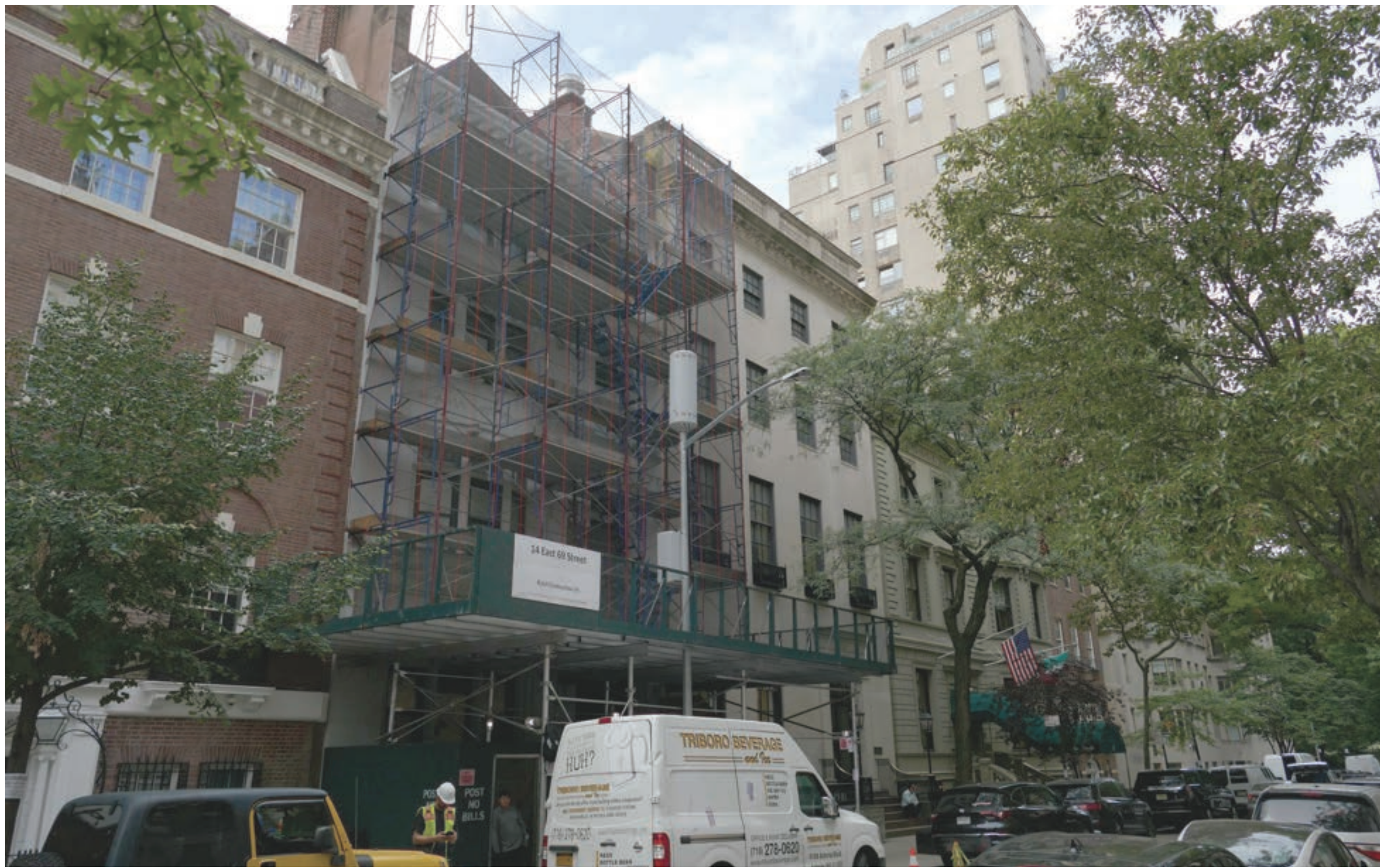
VIEW FROM 69TH STREET
