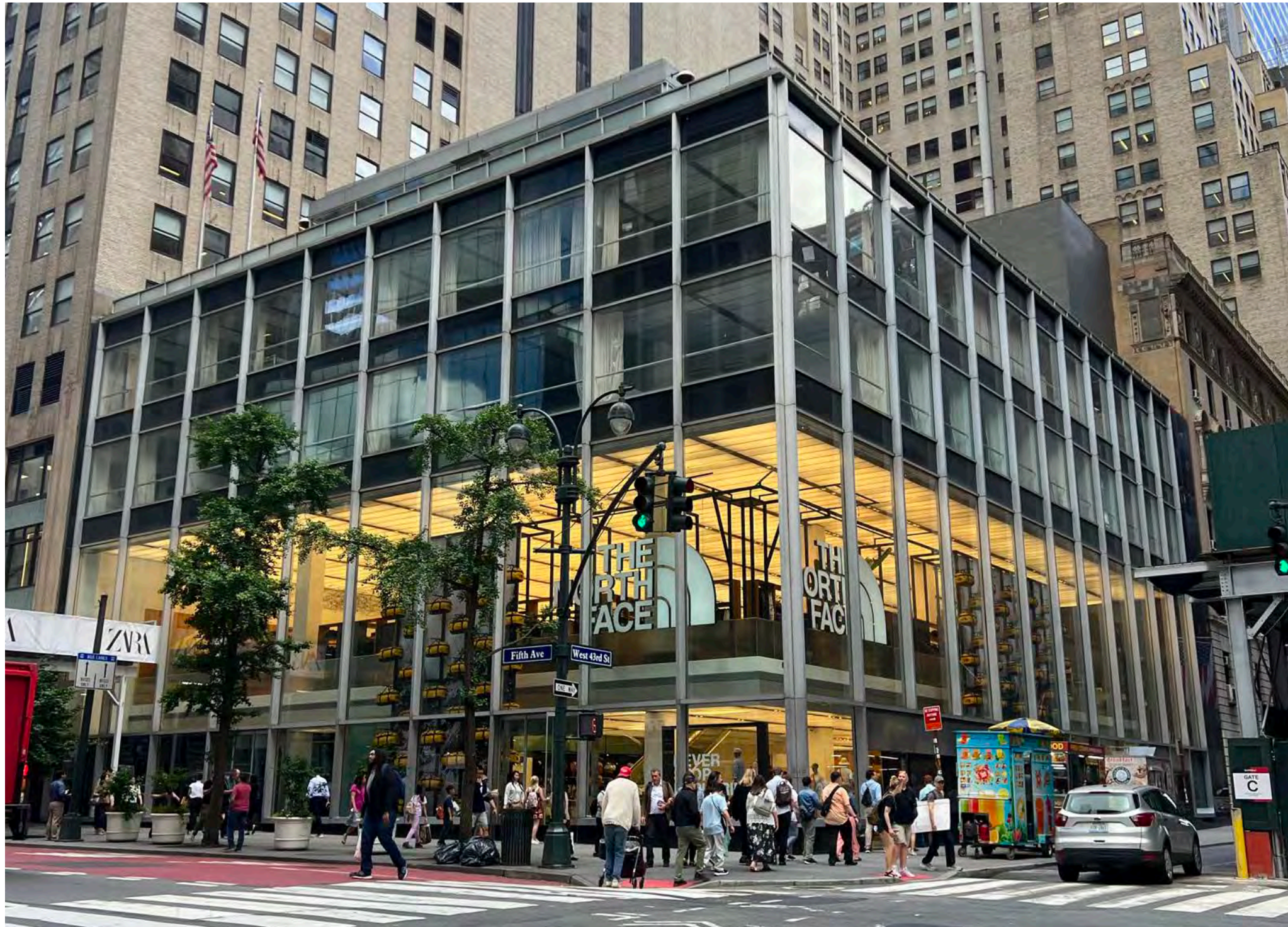
VIEW FROM FIFTH, LOOKING SOUTHWEST.
