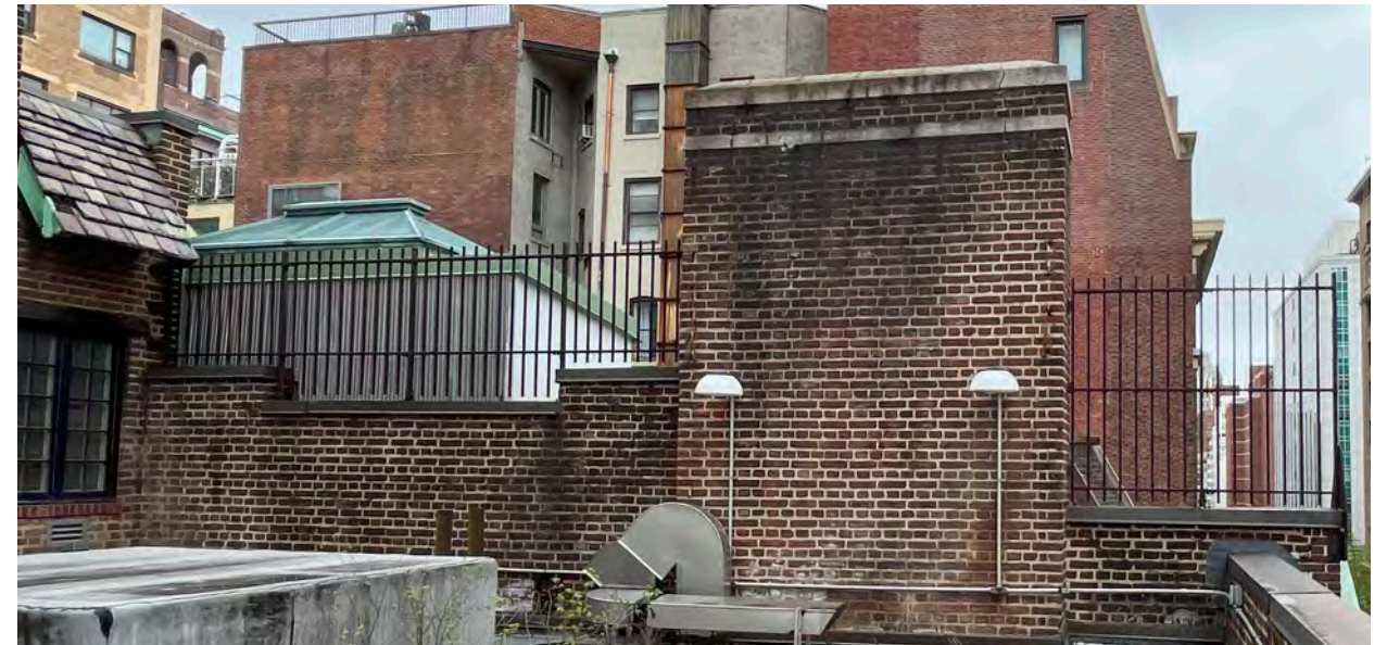
photo of east wall on penthouse level
