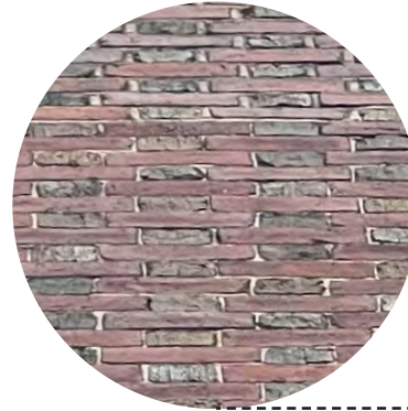
existing brick detail
