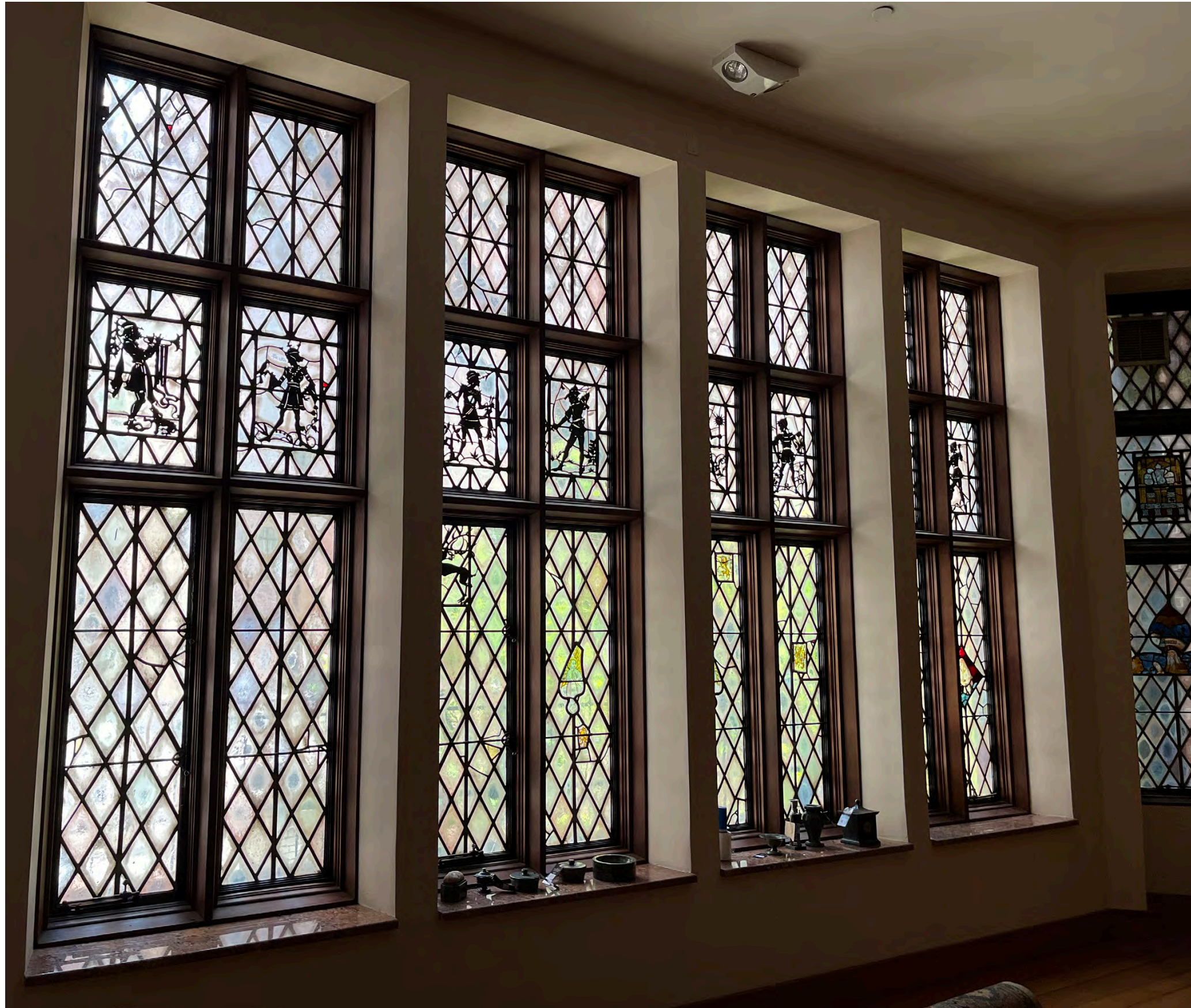
Third floor rear - interior
