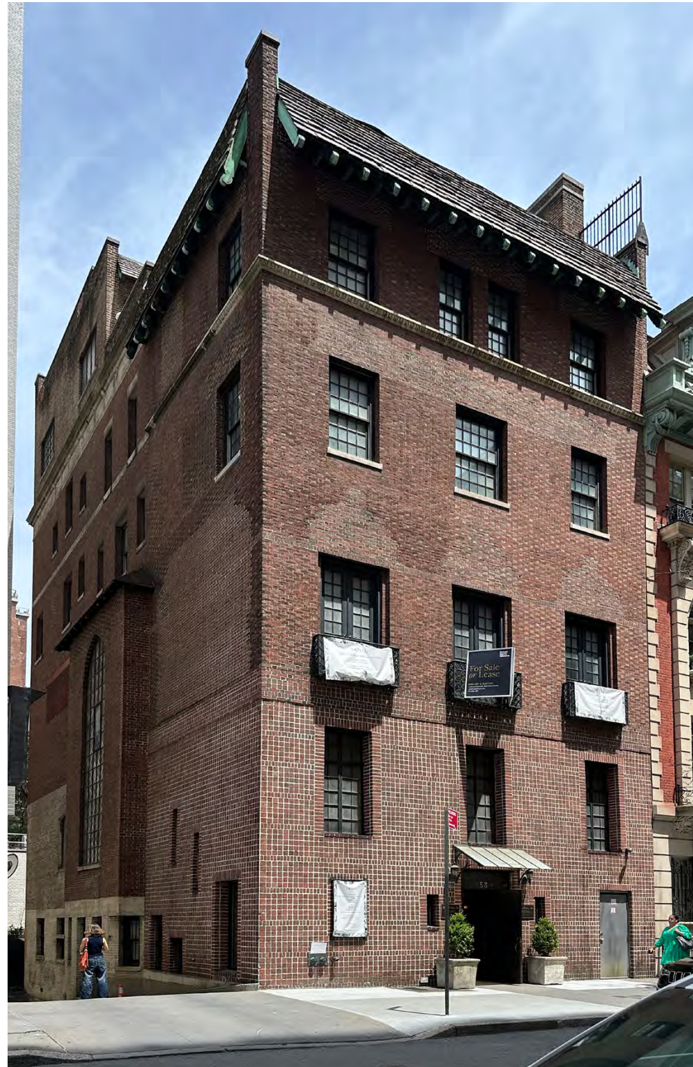
existing facade photo - modified 1926
