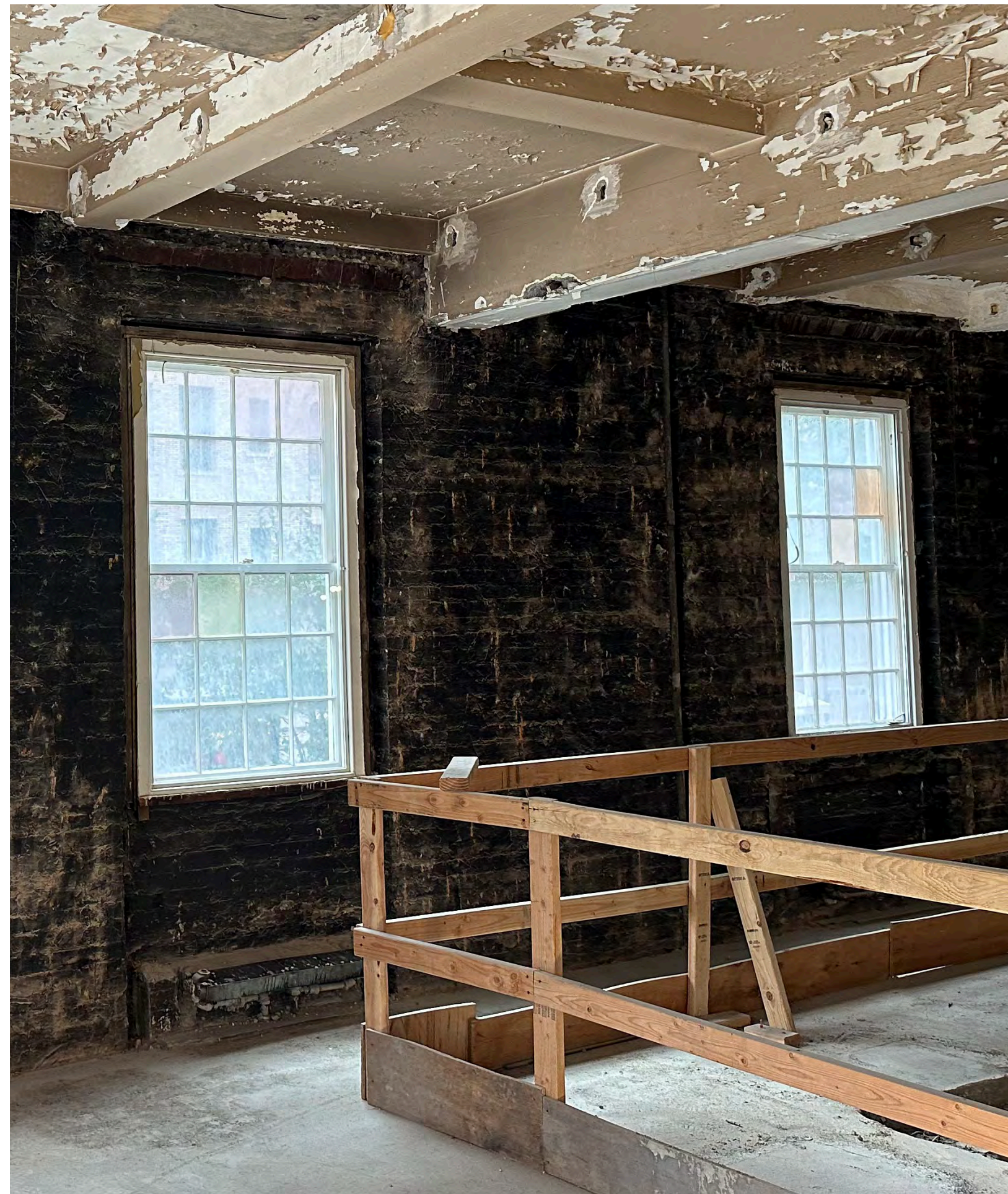
INTERIOR DOUBLE-HUNG WINDOW CONDITIONS
