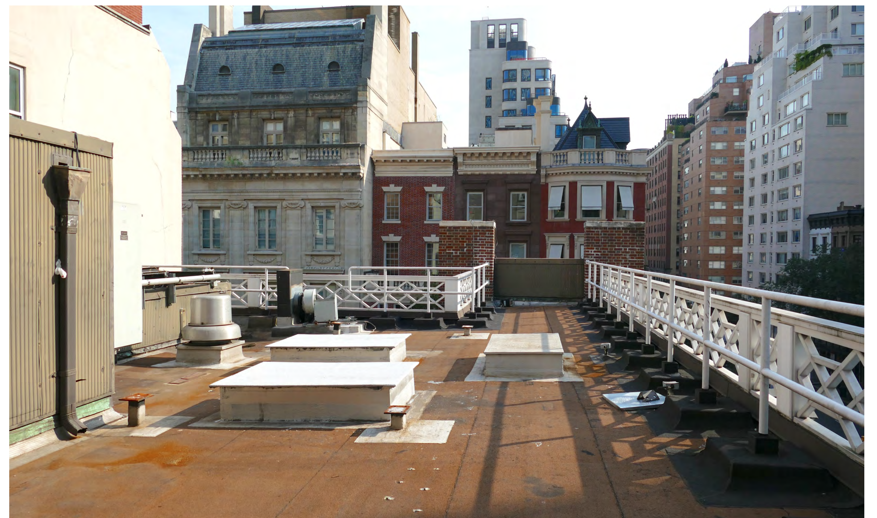
OVERALL VIEW OF ROOF, LOOKING NORTH
