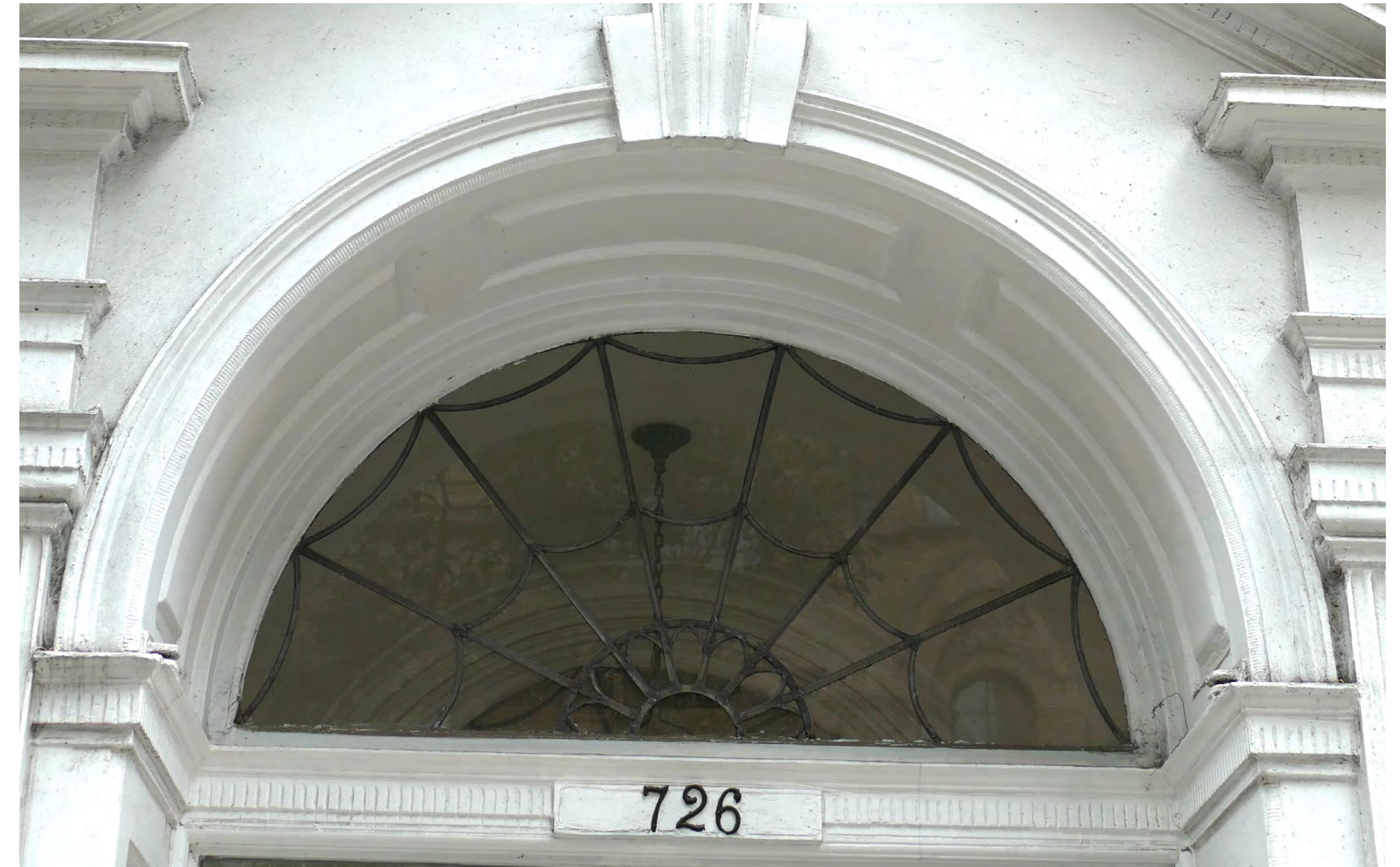
DETAIL VIEW OF WOOD ENTRANCE DOOR SURROUND AND HISTORIC FANLIGHT
