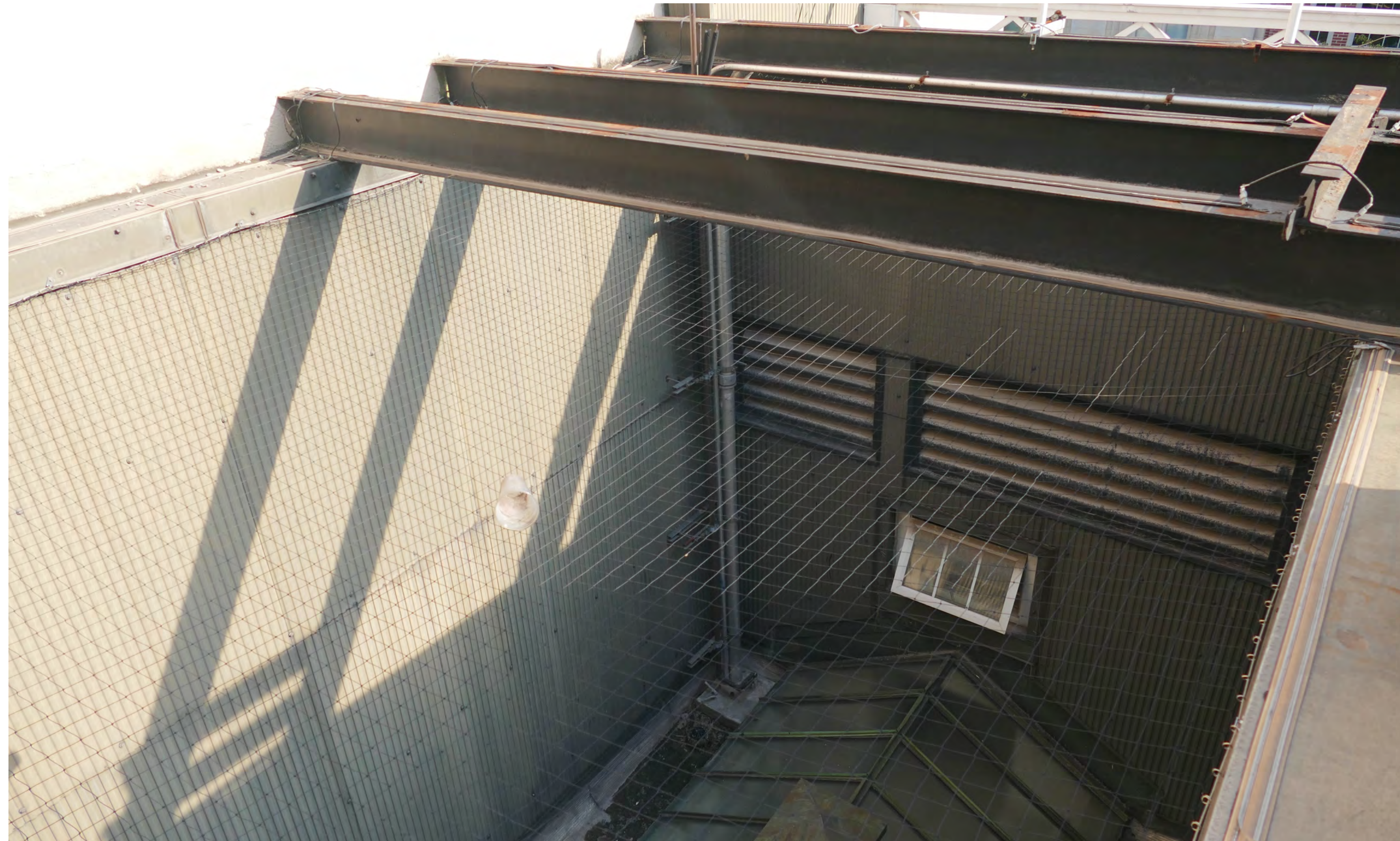
DETAIL VIEW OF LIGHT-WELL AT WEST SIDE OF ROOF
