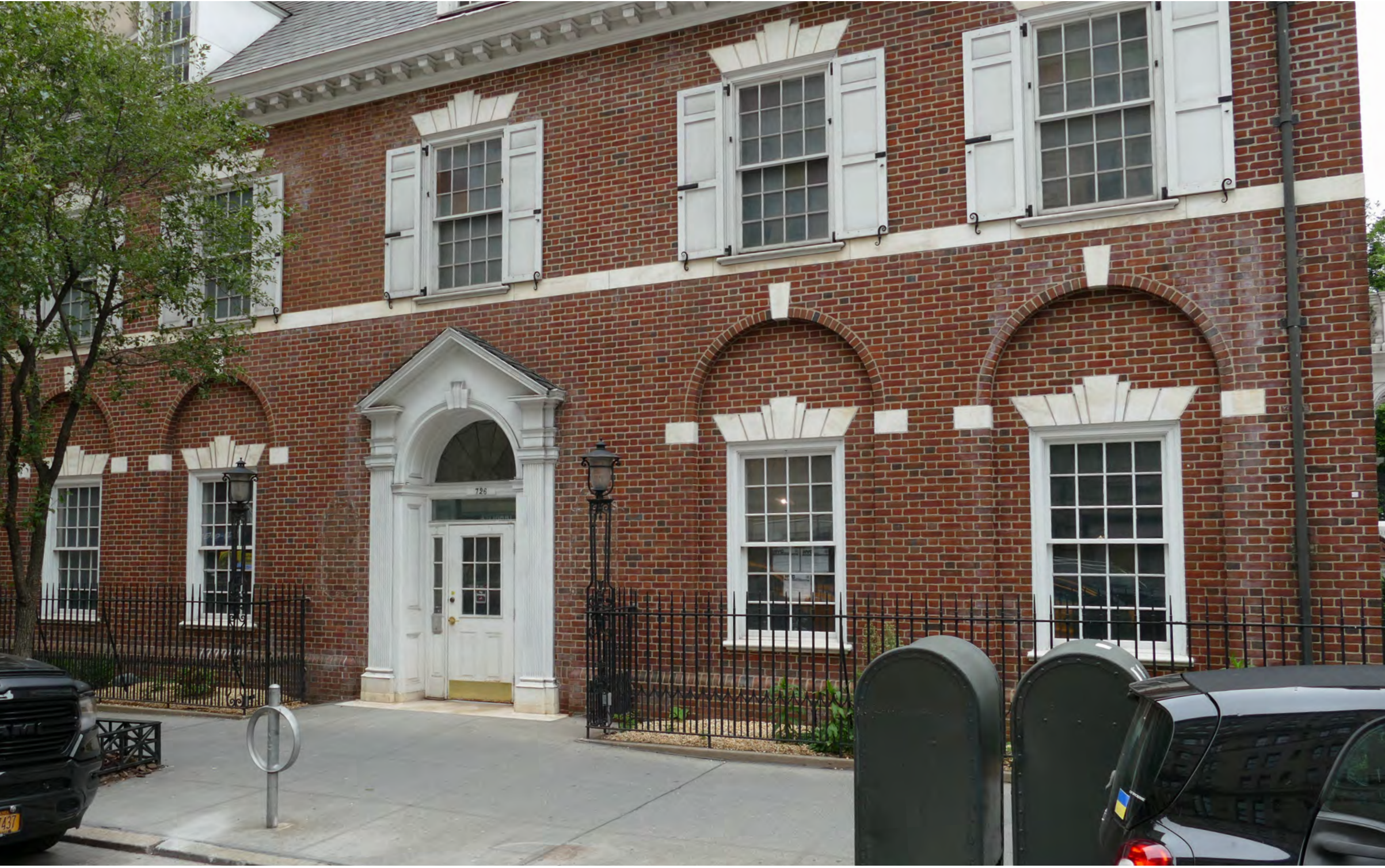
VIEW OF THE MADISON AVENUE FACADE
