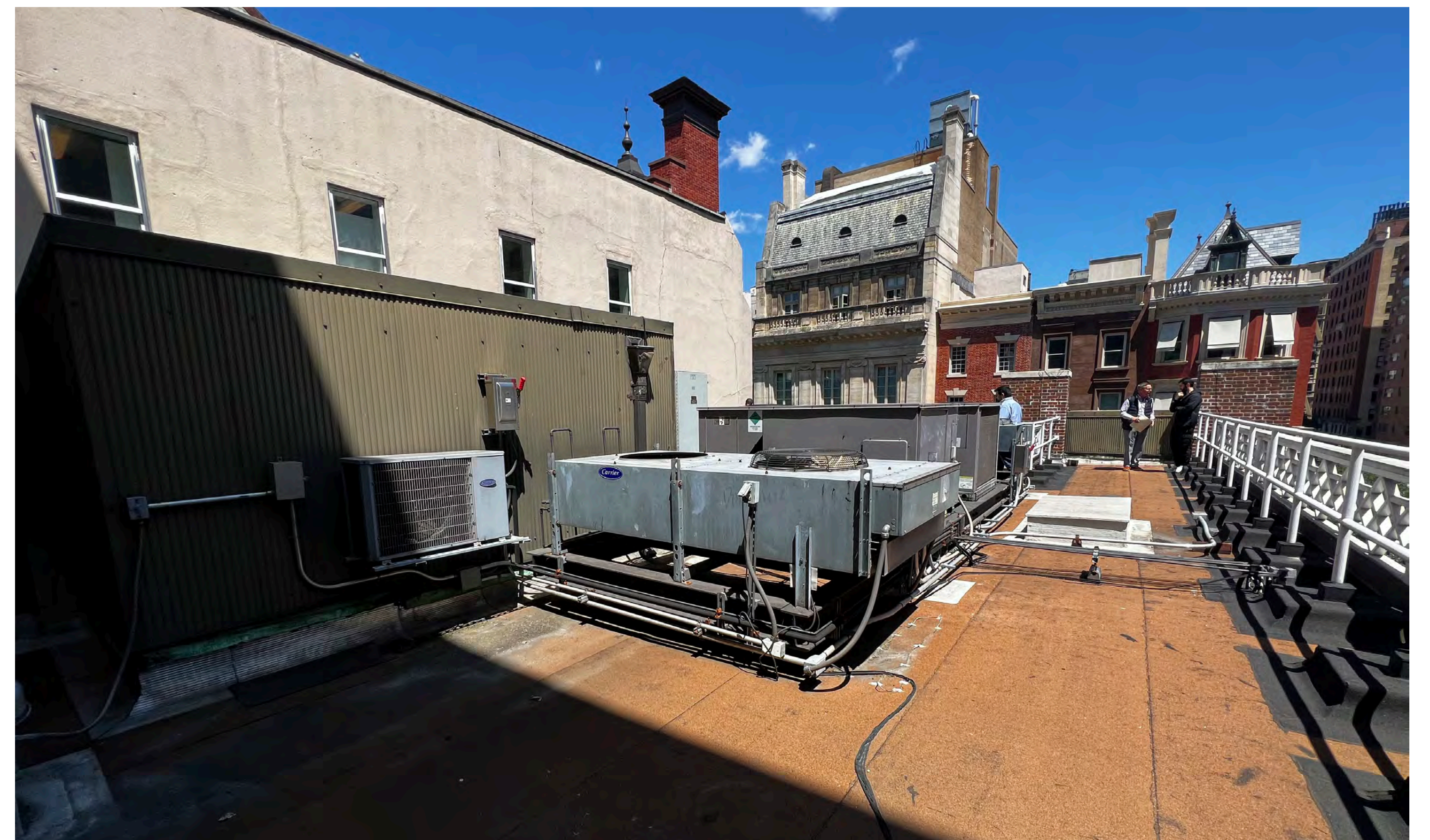
OVERALL VIEW OF ROOF, LOOKING NORTH, BEFORE HVAC REMOVAL
