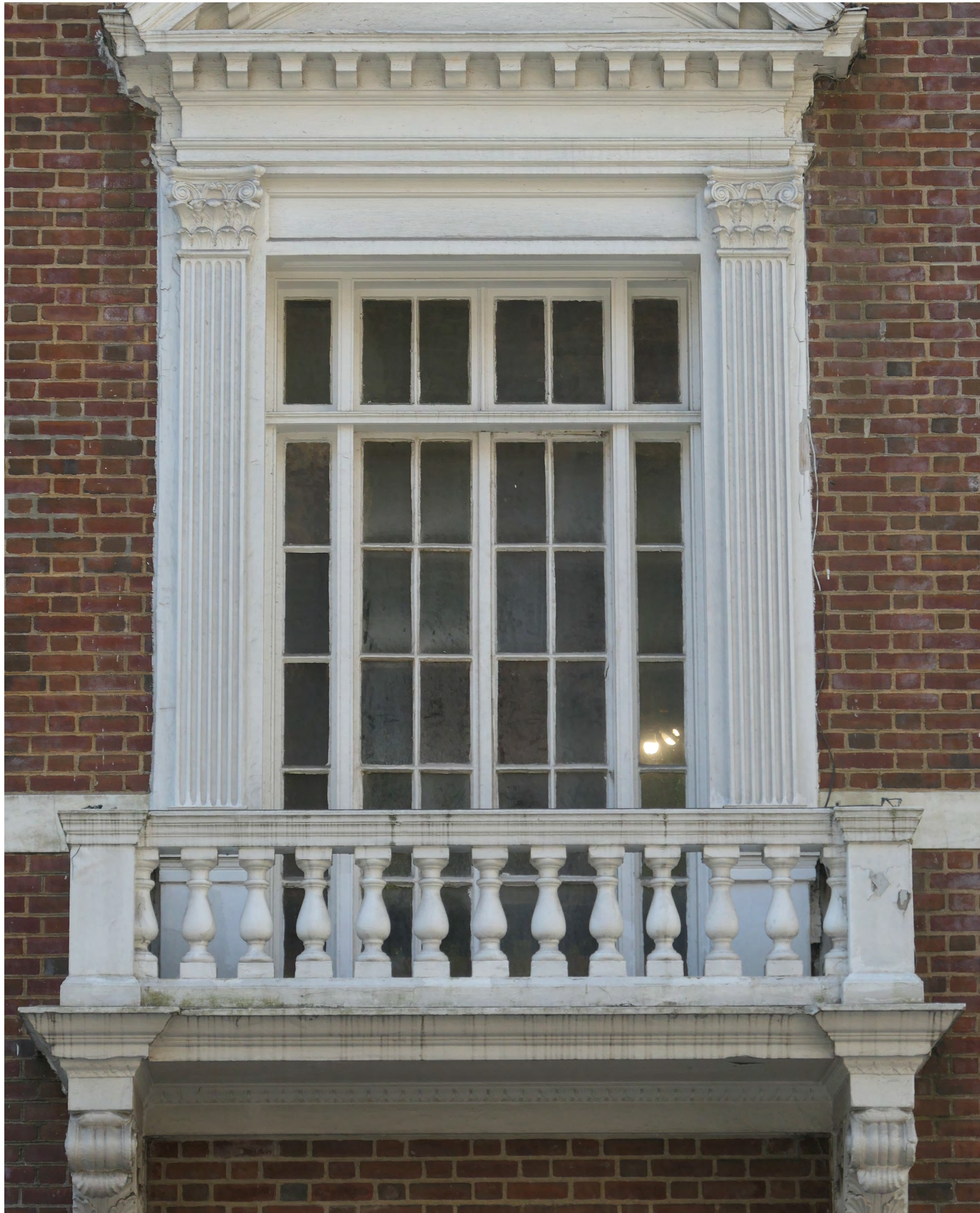
EXISTING SECOND FLOOR CASEMENT DOORS AND SIDELIGHTS ON EAST 64TH STREET
