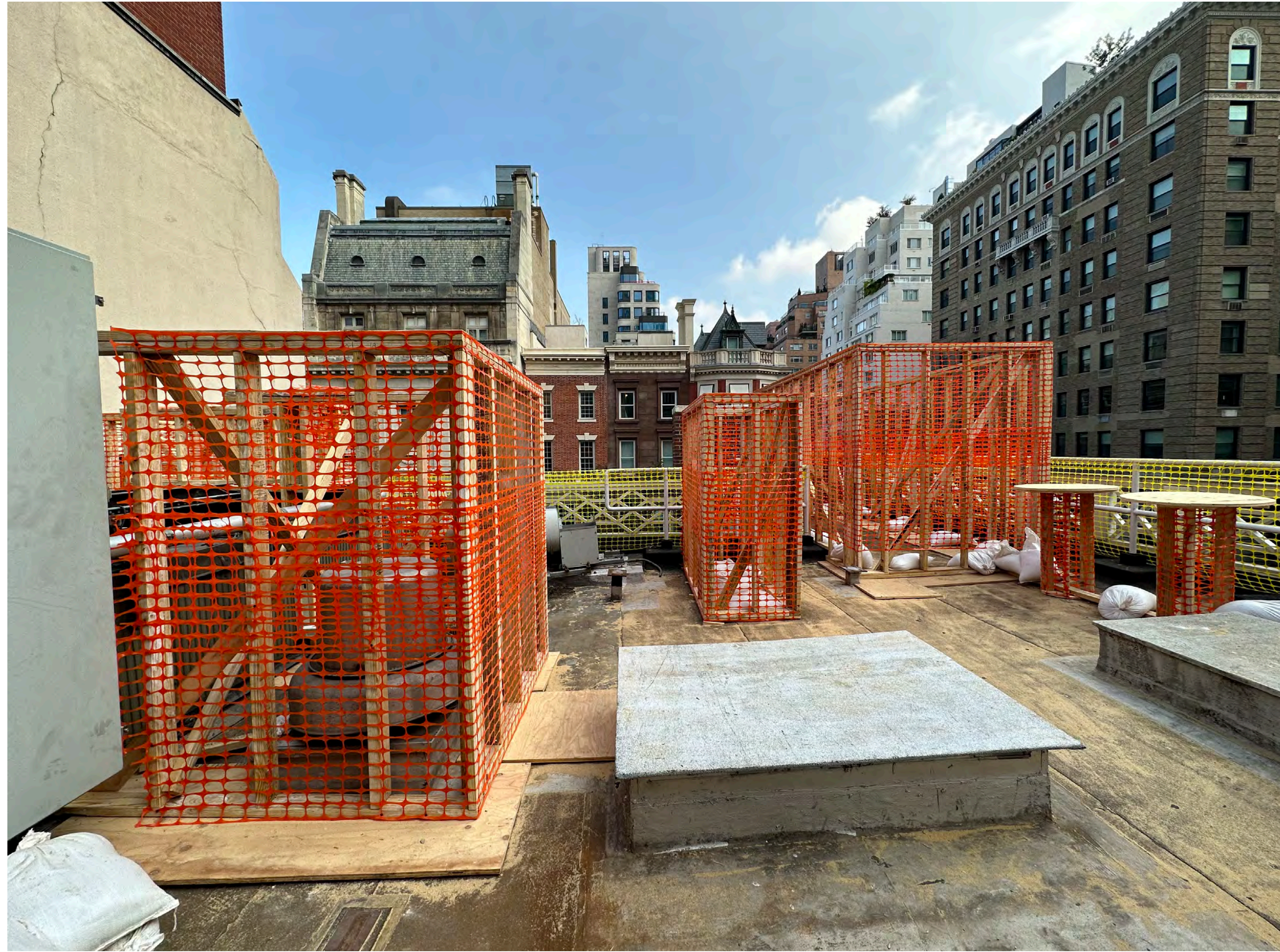
VIEW OF MOCK-UP FROM ROOF
