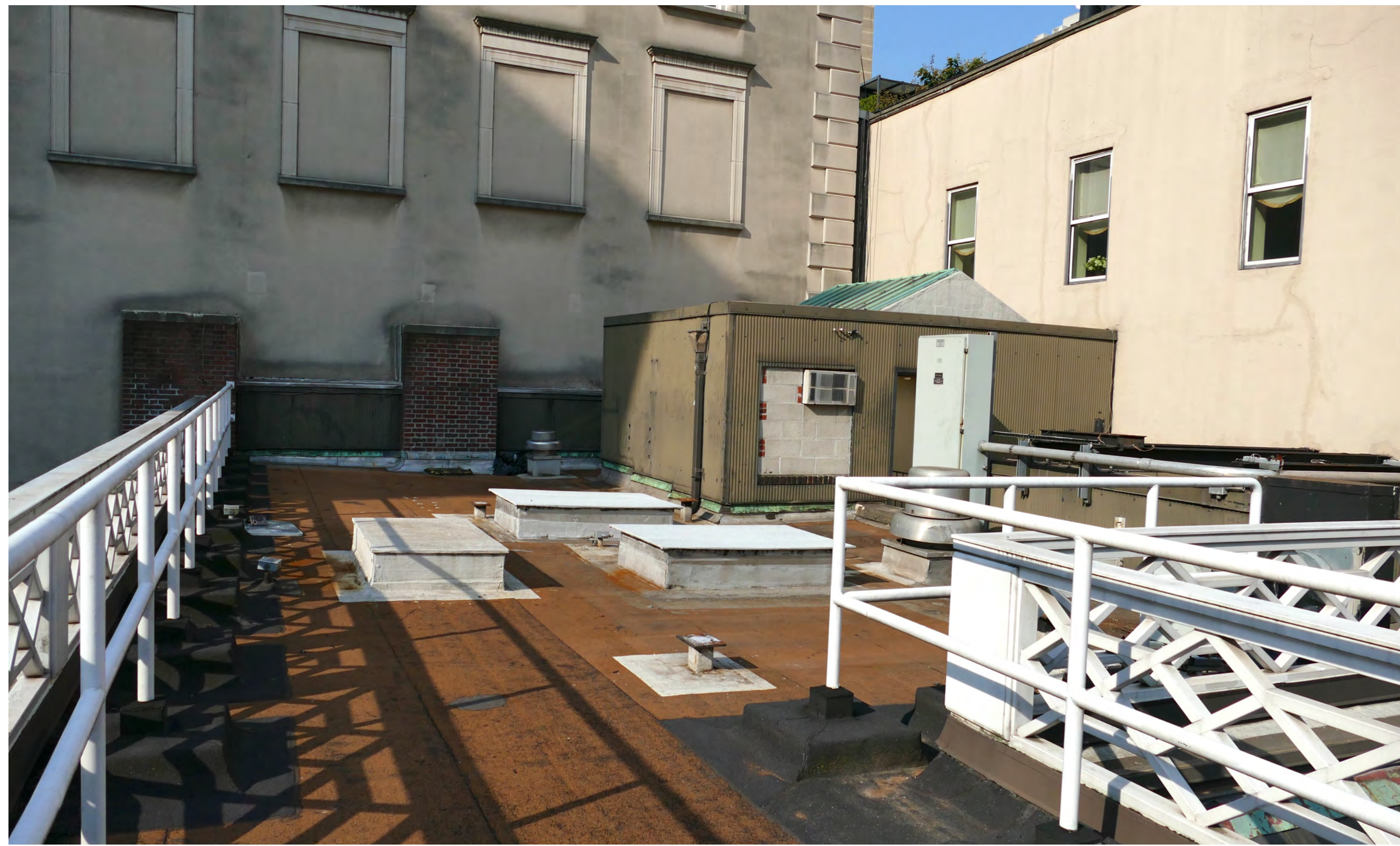
OVERALL VIEW OF ROOF, LOOKING SOUTH
