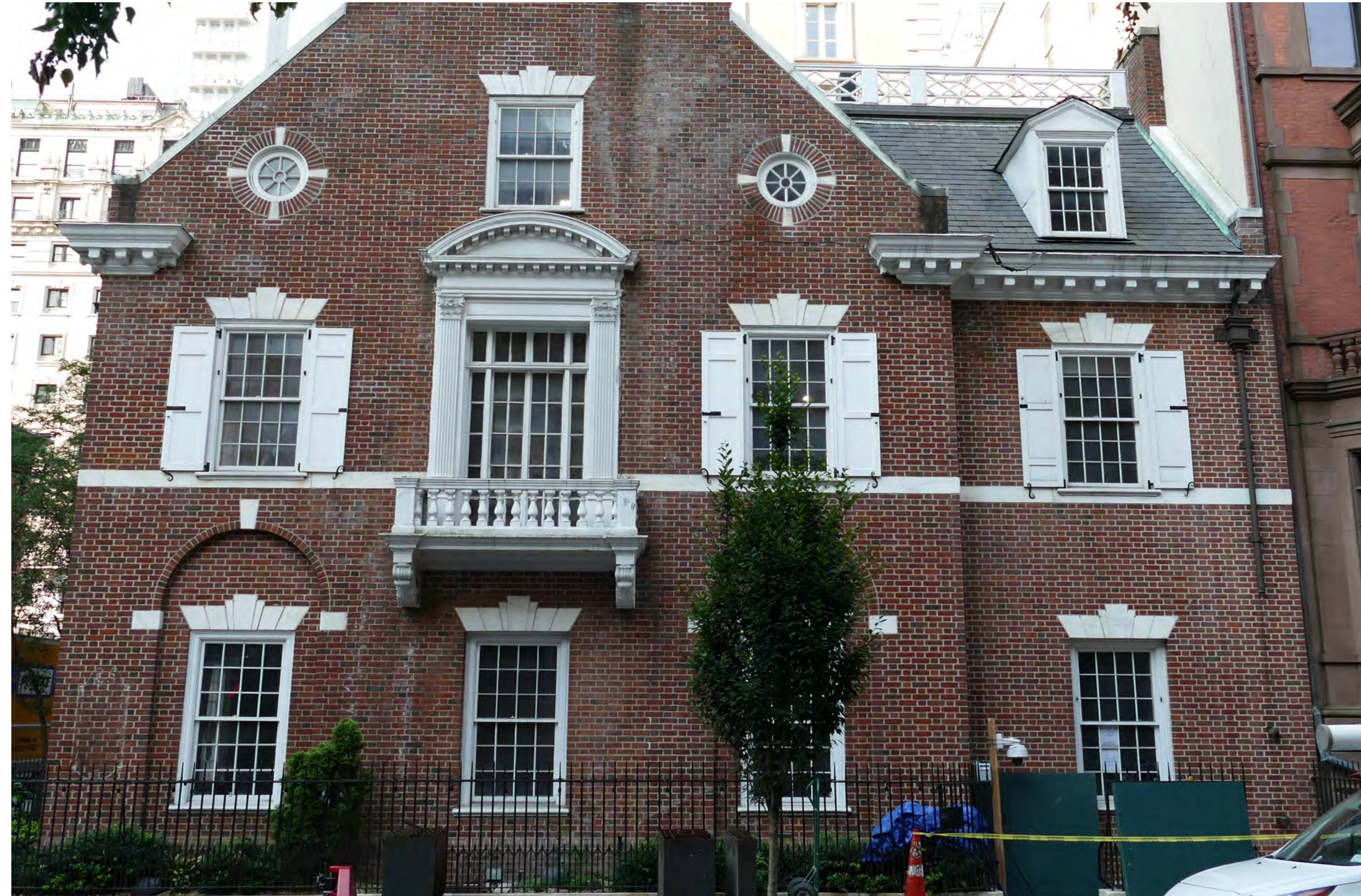
VIEW OF THE EAST 64TH STREET FACADE
