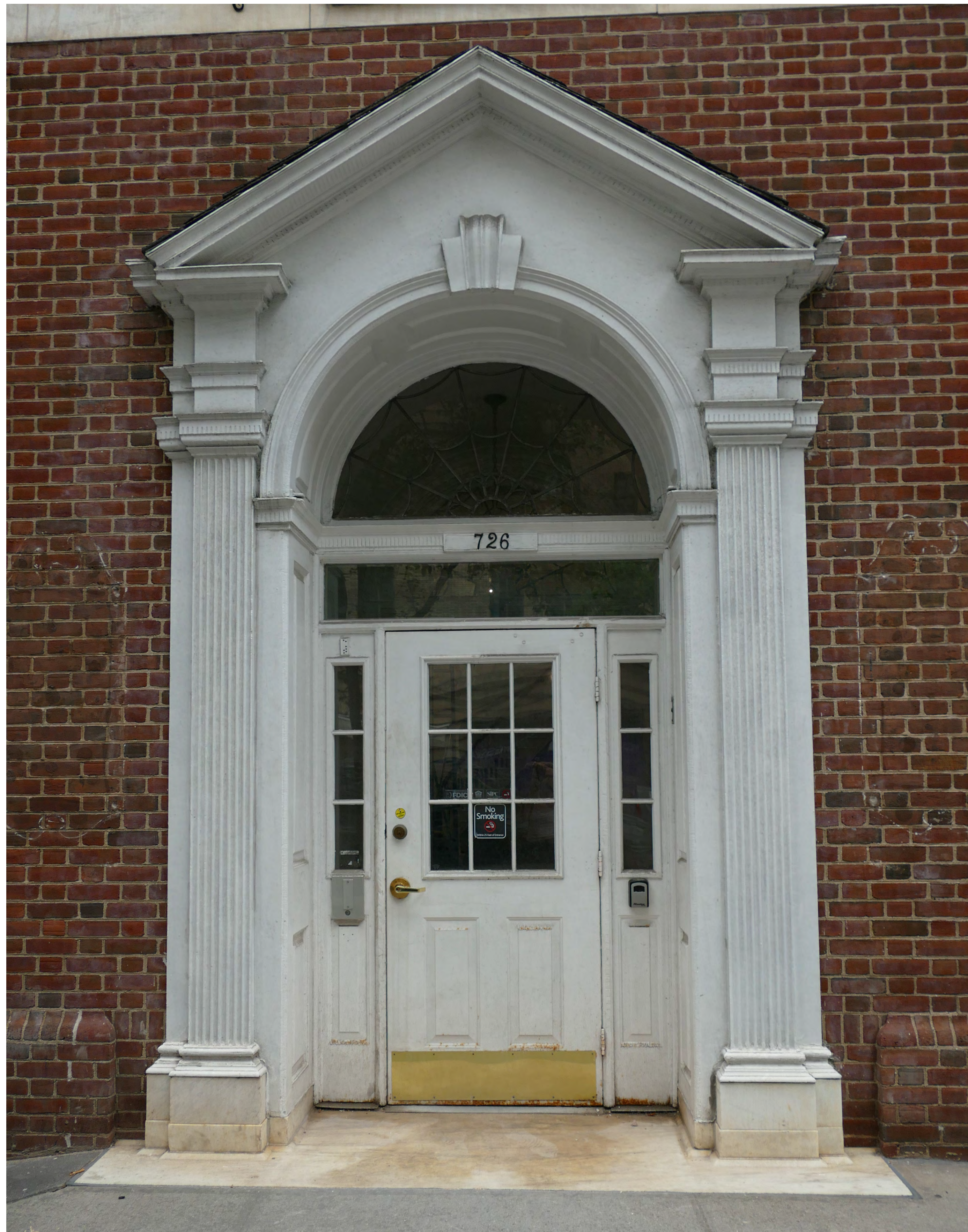
MAIN ENTRANCE DOOR MADISON AVENUE
