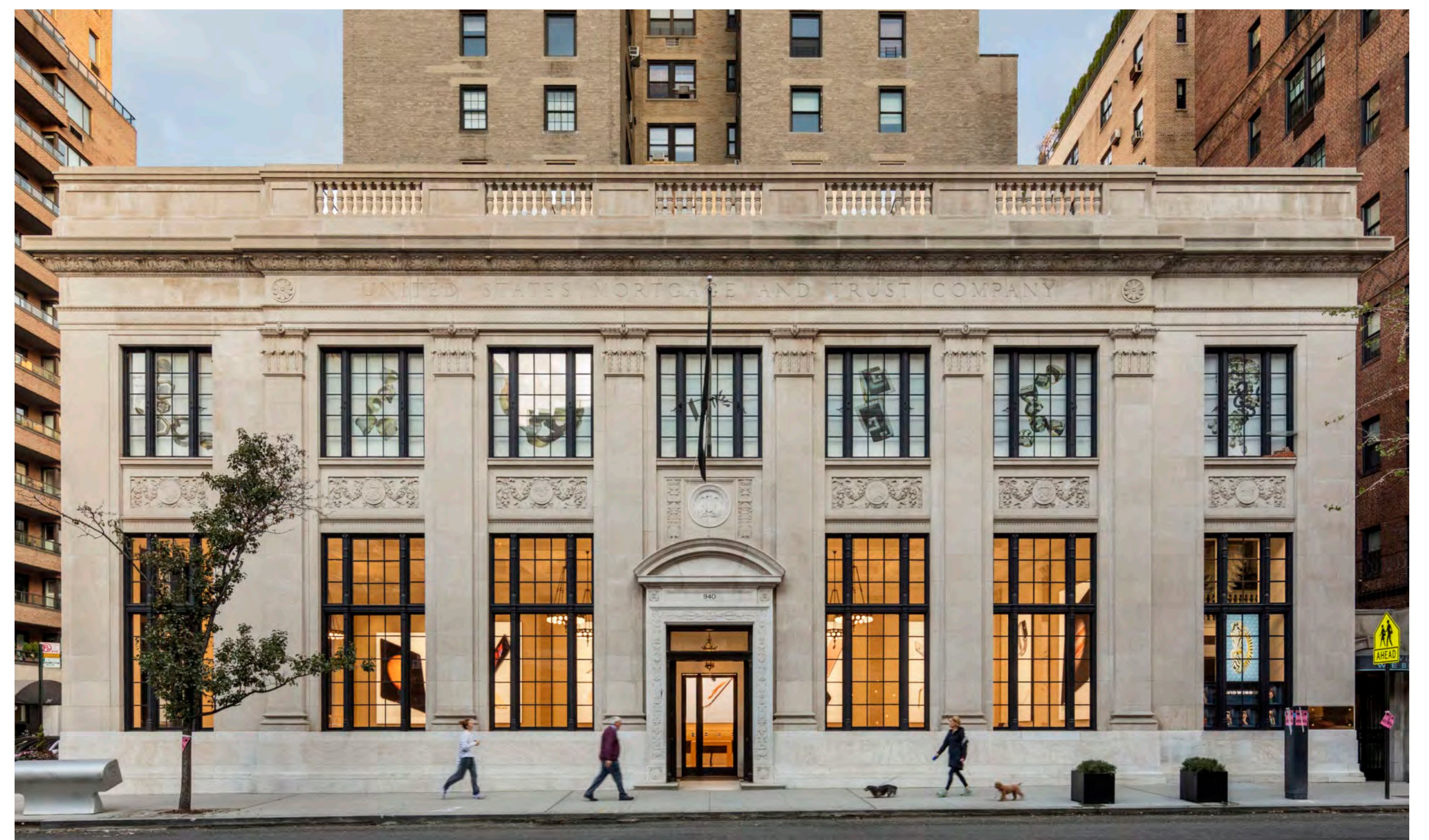
940 MADISON AVENUE, ORIGINALLY UNITED STATES MORTGAGE AND TRUST COMPANY (BOHLIN CYWINSKI JACKSON)
