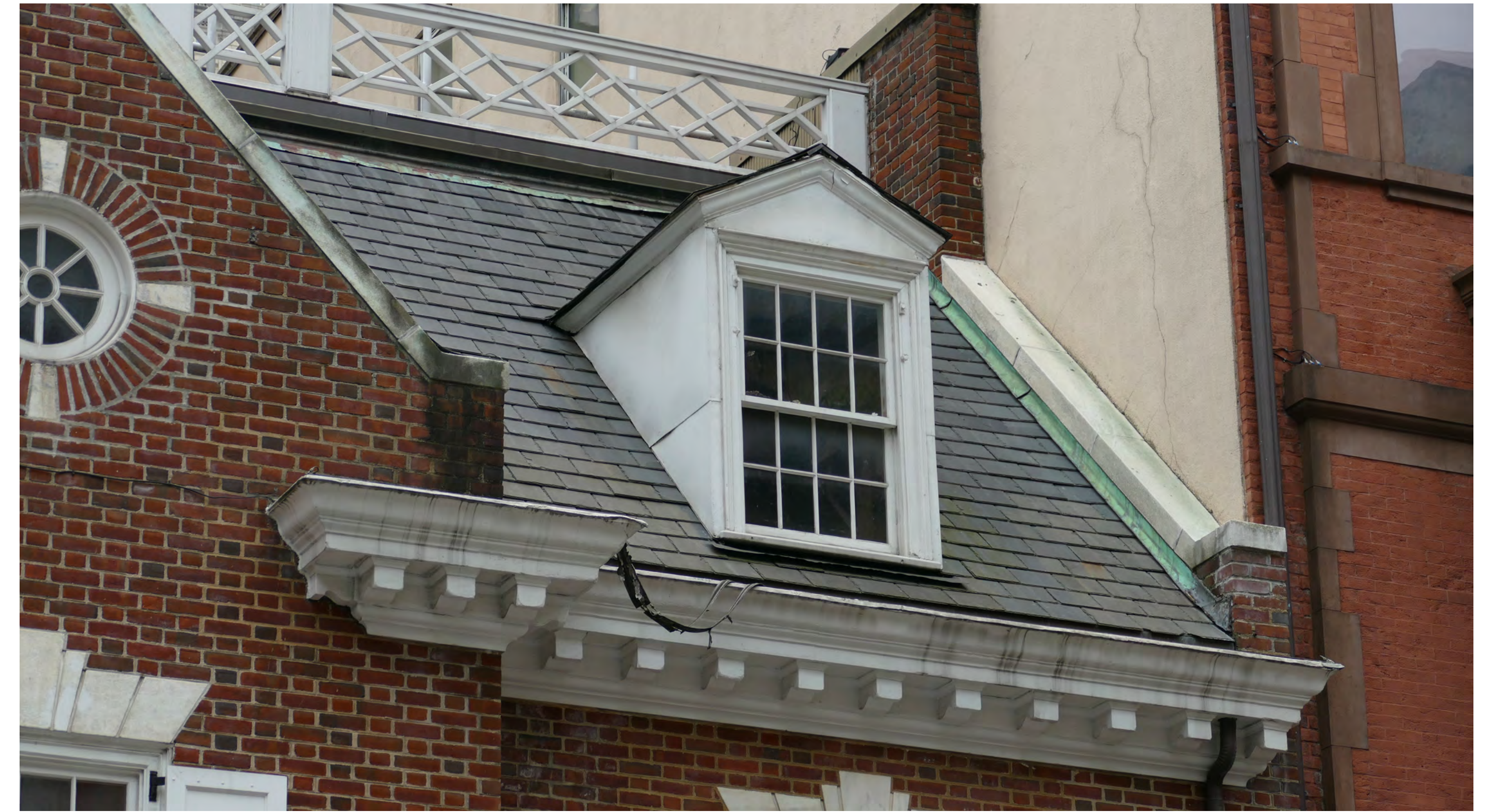
DETAIL VIEW OF A WOOD DORMER ON EAST 64TH STREET
