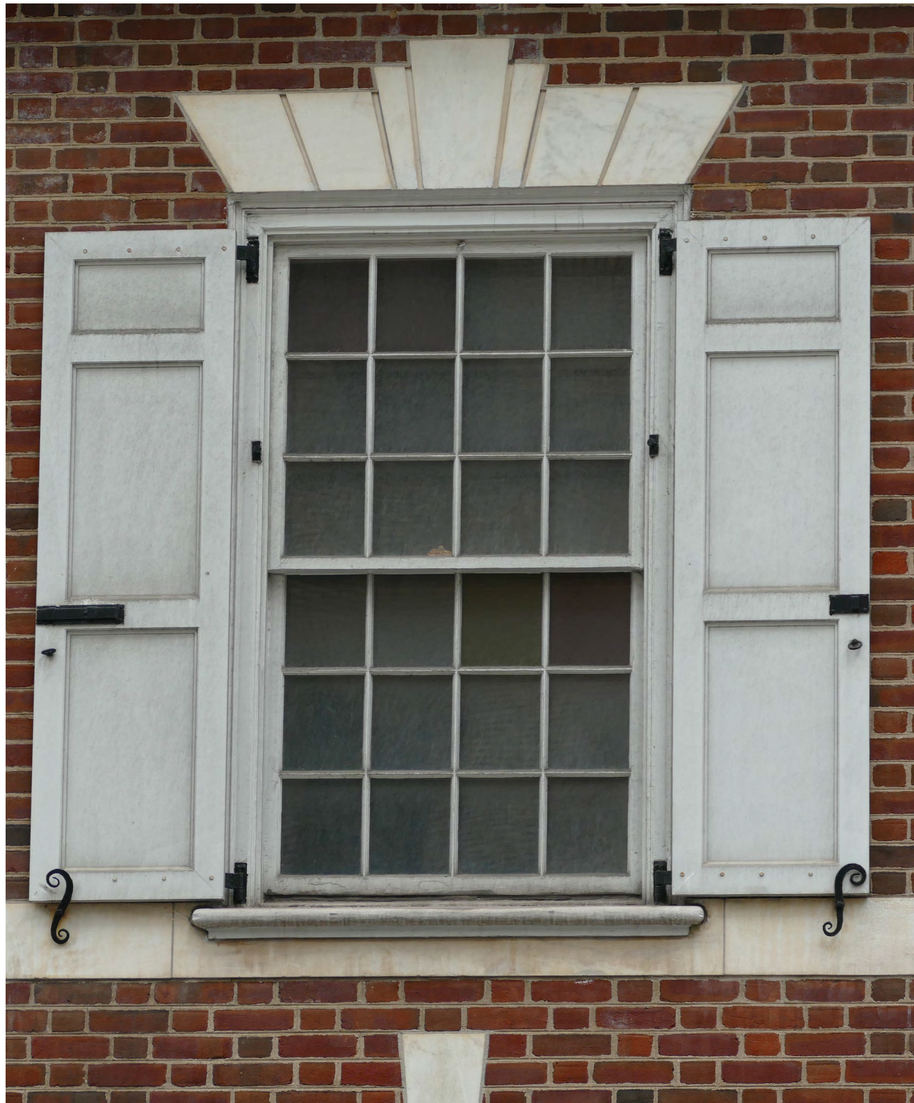
EXISTING DOUBLE-HUNG WOOD WINDOW, TYPICAL CONDITION
