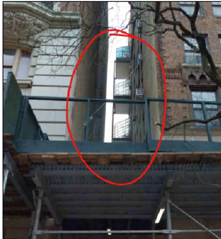
330 WEST END AVENUE (2021) - THE REPLACEMENT OF VISIBLE GREENHOUSES WAS APPROVED, SEEN FROM EAST 76TH STREET.
