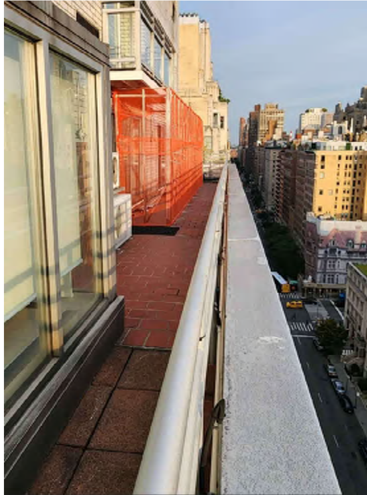
MOCK-UP SOUTH TERRACE AT 14TH FLOOR VIEW FROM 5TH AVE
