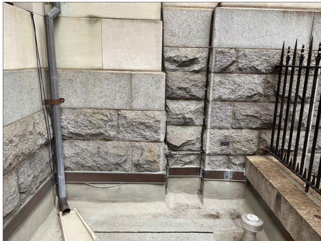
Existing Low Roof Facing South
