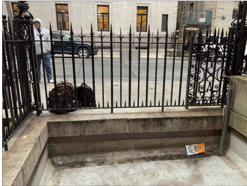
Existing Low Roof Facing 84th St
