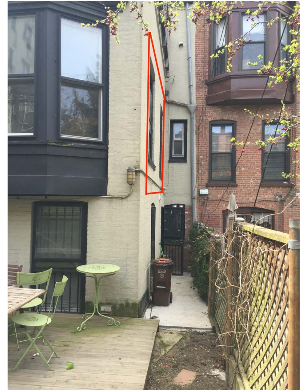
PHOTOGRAPH OF WEST REAR FACADE
