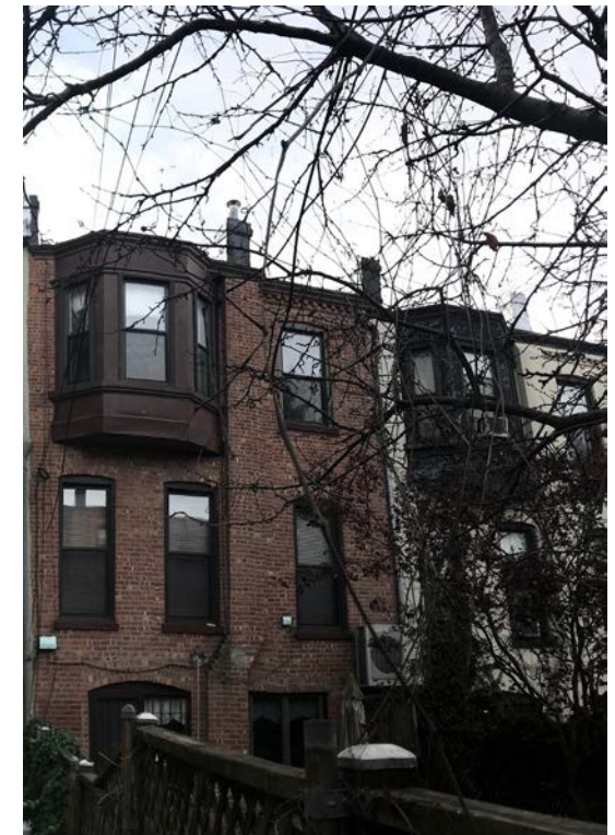
563 9TH STREET REAR FACADE FROM PROPERTY
