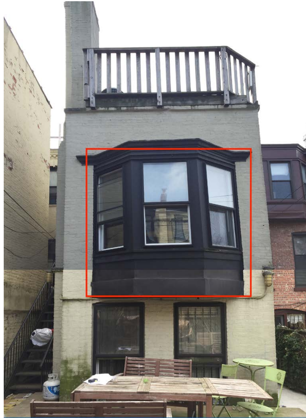
PHOTOGRAPH OF NORTH REAR FACADE
