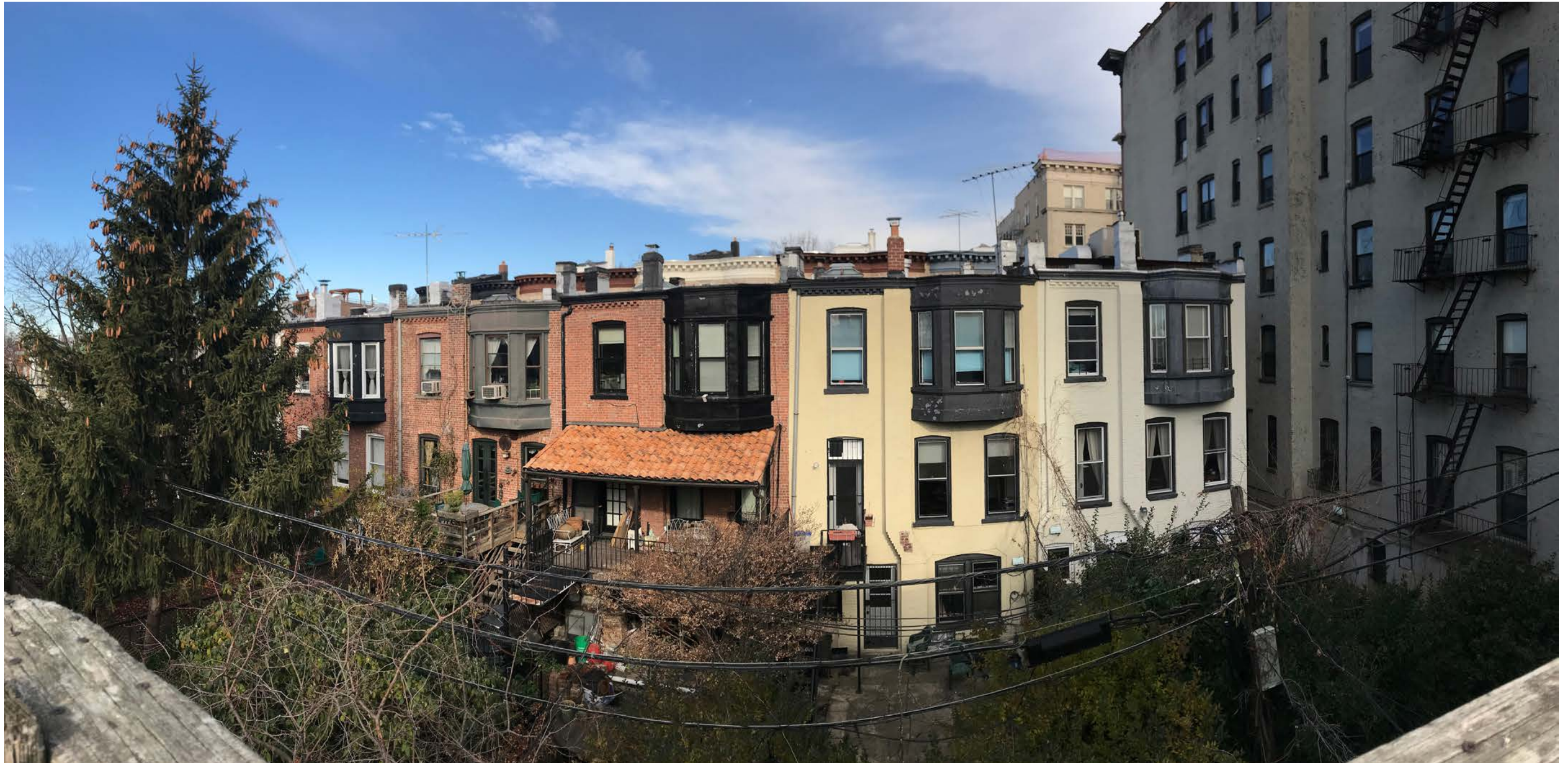
PHOTO PANORAMA OF EXISTING CONDITIONS AT BACKYARD
