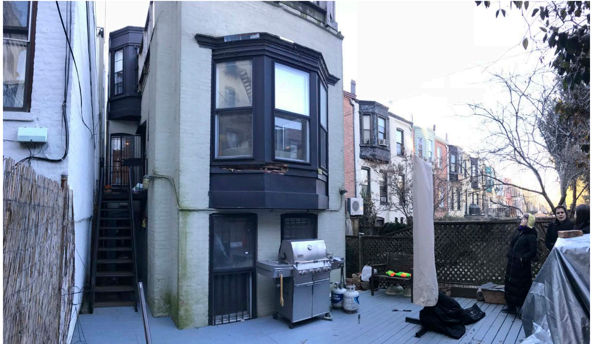
PHOTO OF REAR FACADE IN CONTEXT
