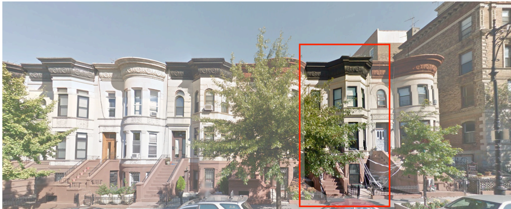
FRONT FACADE IN CONTEXT
