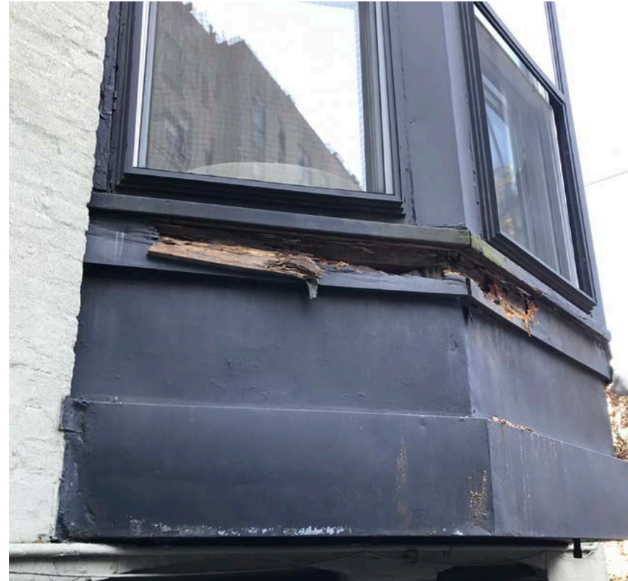
EX'G CONDITIONS AT BAY WINDOW RIGHT SIDE
