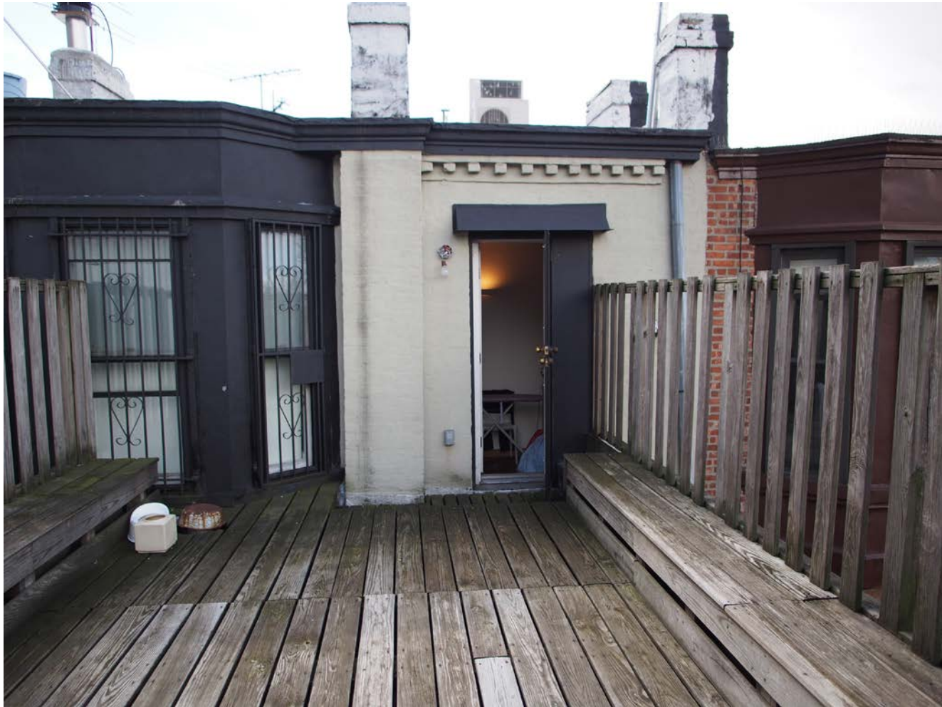
PHOTOGRAPH OF EXISTING CONDITION AT TERRACE
