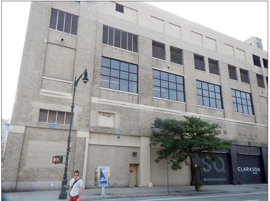
Eastward view to the northern portion of the St. John's Terminal Building's west façade 1
