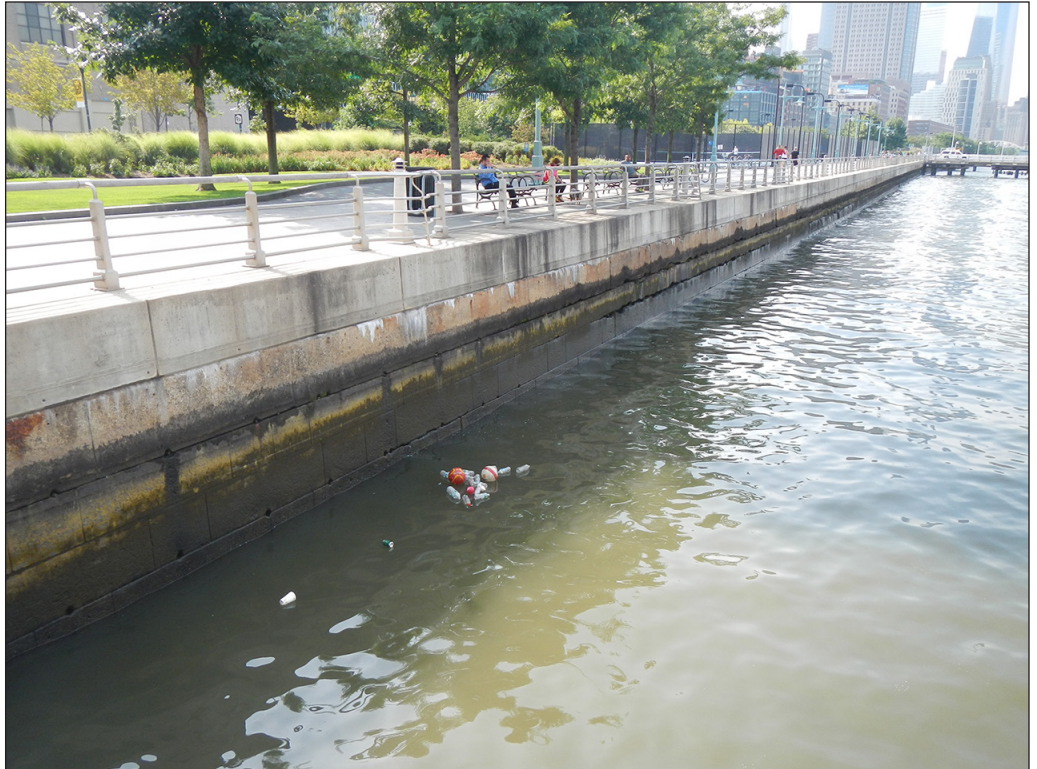
Hudson River Bulkhead, portion visible from south of Pier 40 6
