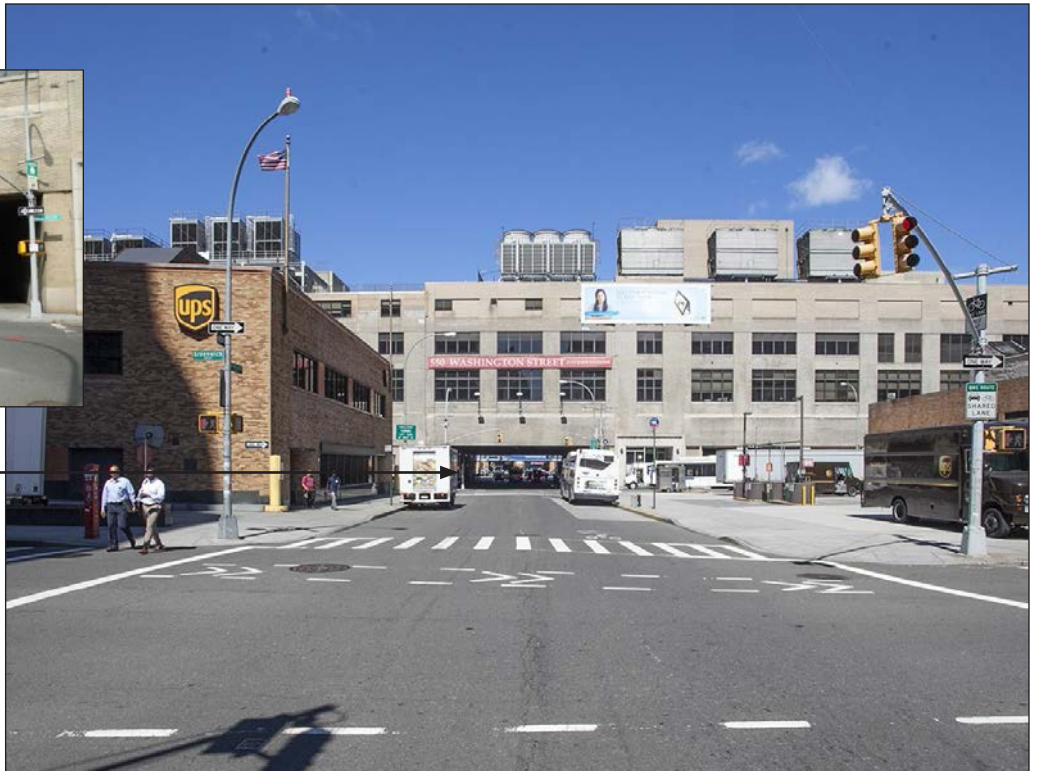
Western view on West Houston Street to the St. John's Terminal Building's east façade and underpass 5
