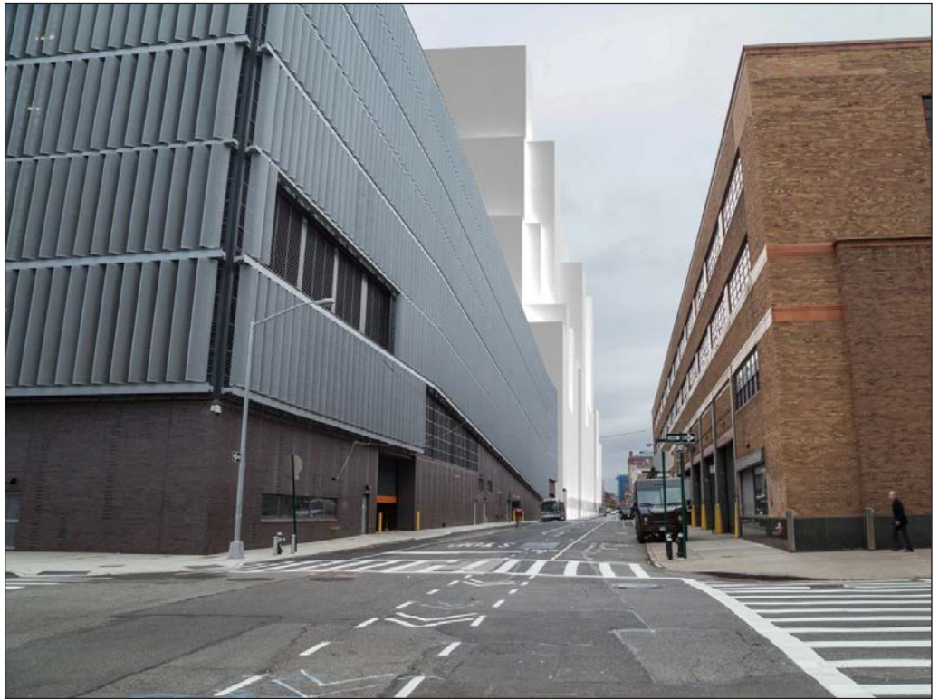
With Action View with the South Site Office Building 39b
