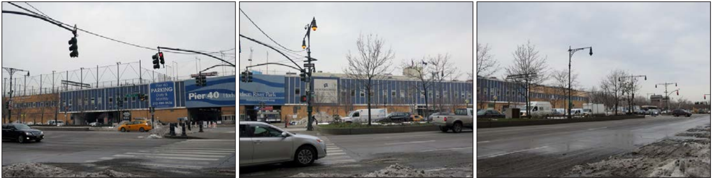
Western view to the Pier 40 Headhouse from the development site 9
