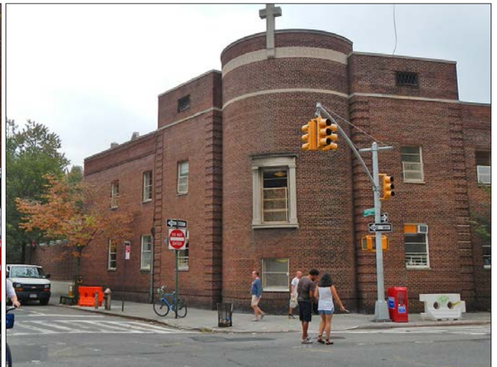
Barrow Street building within the Church of St. Luke in the Field complex in the Greenwich Village Historic District 17
