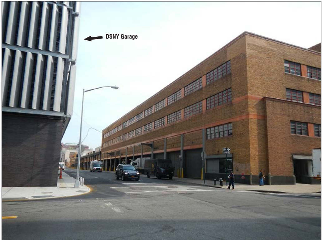
UPS facility on Washington Street across from the development site 11
