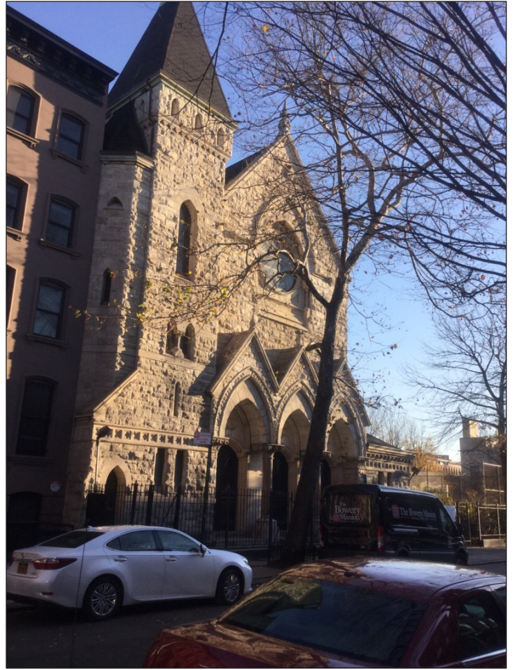
North side of West 130th Street C3
