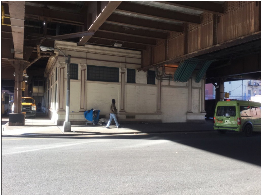
Metro-North 125th Street Station 10c
