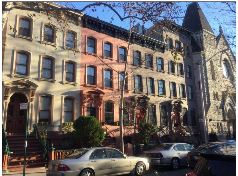
North side of West 130th Street C2
