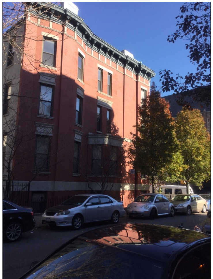
2056-2034 Madison Avenue view from East 129th Street A2
