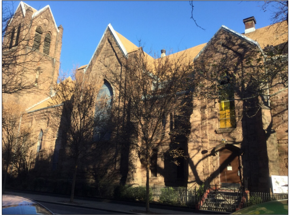
Former St. James Methodist Episcopal Church 8c
