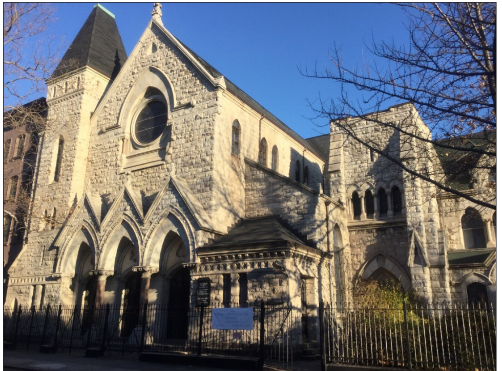
North side of West 130th Street C4
