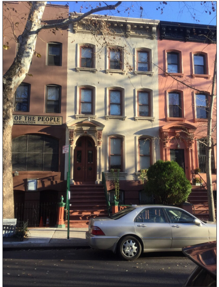
North side of West 130th Street C1
