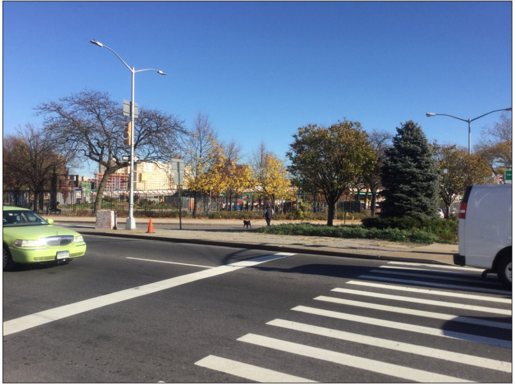
At-grade entrance ramps to Harlem River Drive creates irregular block shapes and a physical barrier in the study area. Green spaces and parks, such as the Crack is Wack Playground seen in the background, occupy the blocks created by the ramp network. View from Second Avenue at East 127th Street looking northeast. 26
