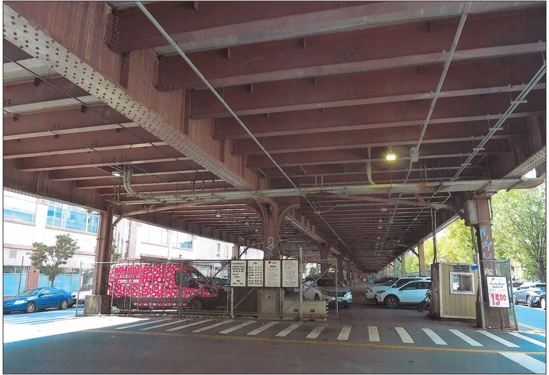
Current Condition 47a
