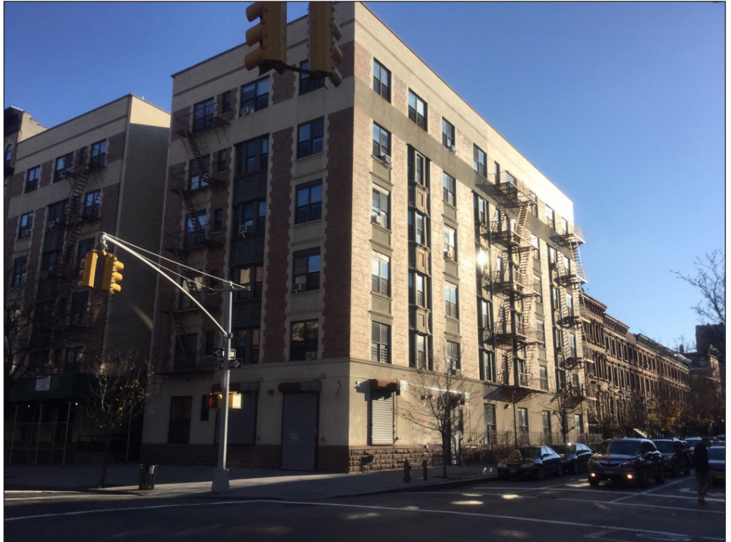
An older, six-story building extends along East 126th Street with smaller, three-story buildings beyond. View from Madison Avenue looking northeast.
