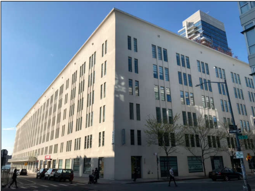
2. View looking north from Kent Avenue and North 3rd Street.
