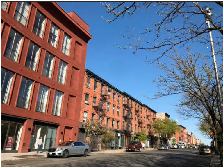
5. North side of Grand Street east of Wythe Avenue in the Grand Street Historic District.
