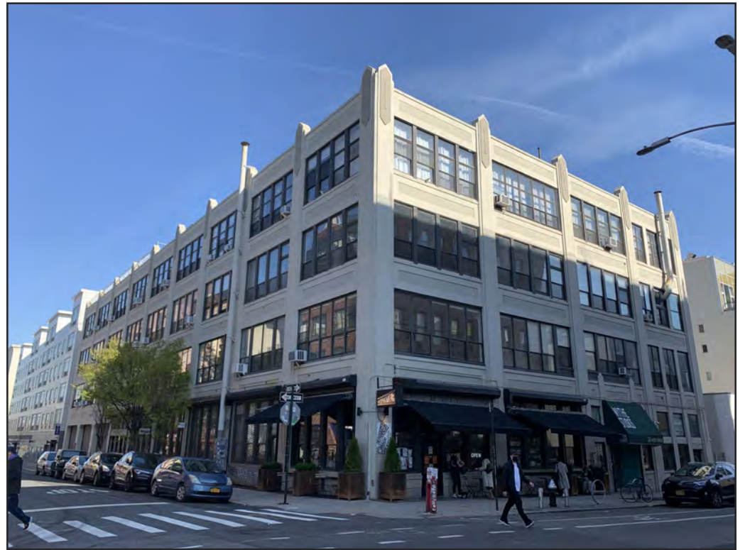
2. Rokeach & Sons Warehouse (S/NR-eligible)
