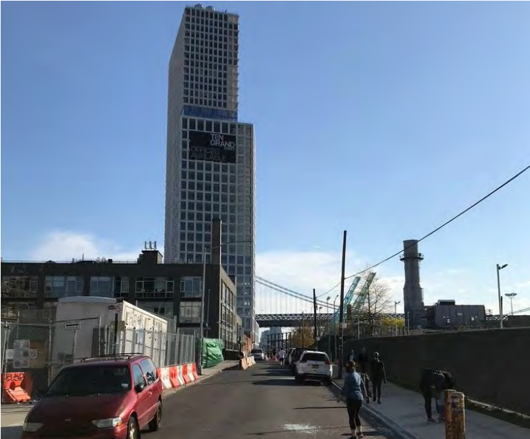
10. View looking south along River Street in the Project Area towards the Green Desk office building, Ten Grand Street, Williamsburg Bridge, and NYPA stacks.
