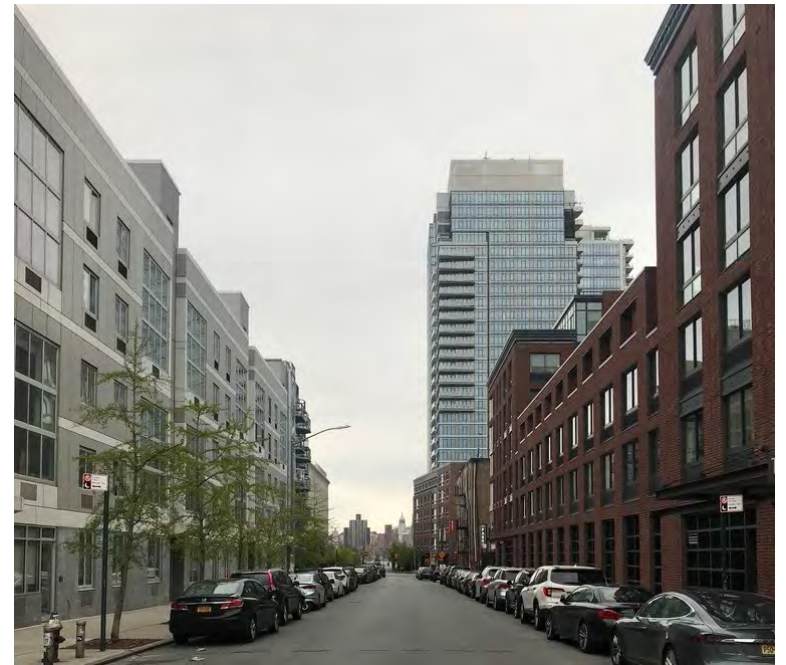
7. New mid-rise buildings on North 4th Street, with a new waterfront tower in the background.
