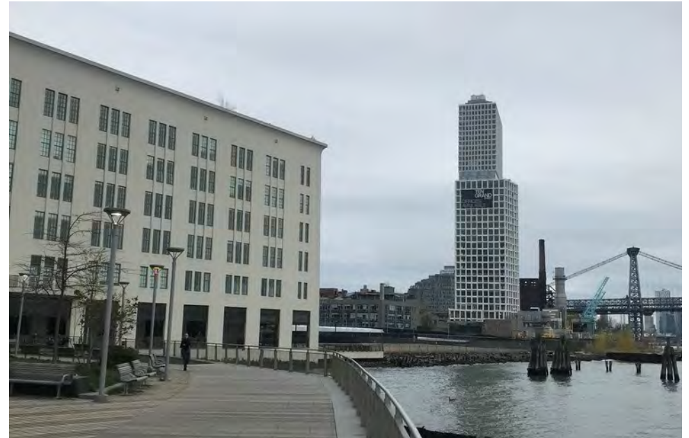
4. View looking south from North 5th Street Park at the Austin, Nichols & Co. Warehouse, Project Area, Ten Grand Street, and the Williamsburg Bridge.
